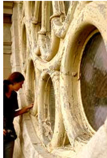
A condition assessment of the frame supporting the stained glass window is as important as evaluating the stained glass itself. Photo: Neal A. Vogel.
