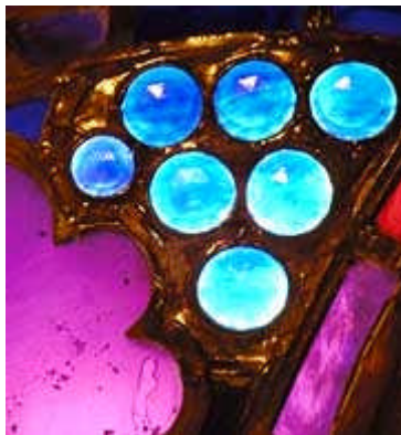
The faceted jewels set in a lead overlay from 1920 were made possible by one of the many glass innovations of the Tiffany Glass & Decorating Company several decades earlier. Photo: Neal A. Vogel.
