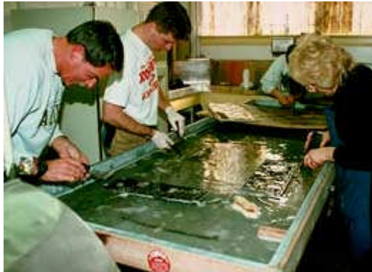
Disassembling leaded glass in warm water helps to soften the putty, minimize breakage, and reduce exposure to airborne dust. Photo: Neal A. Vogel.
