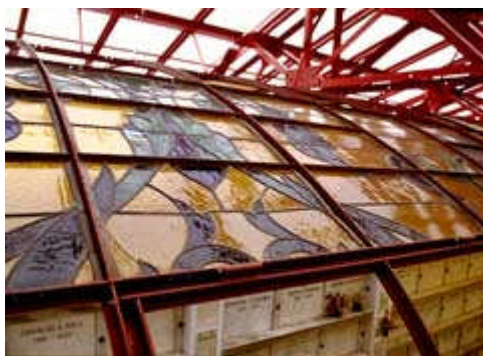
Before repairs began on the vaulted glass ceiling, a new diffusing skylight was installed to correct recurring leaks. Catacombs (ca. 1920), Cypress Lawn Memorial Park, Colma, California. Photo:
