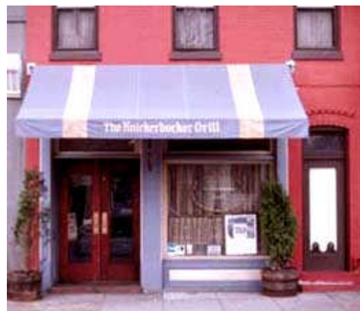
Awnings reduce heat gain in the summer and, when they are raised in the winter, radiant heat from the sun provides free
