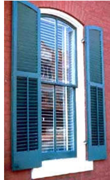
Shutters can be used to minimize the problem of summer heat gain by shading the windows. Photo: NPS files.
