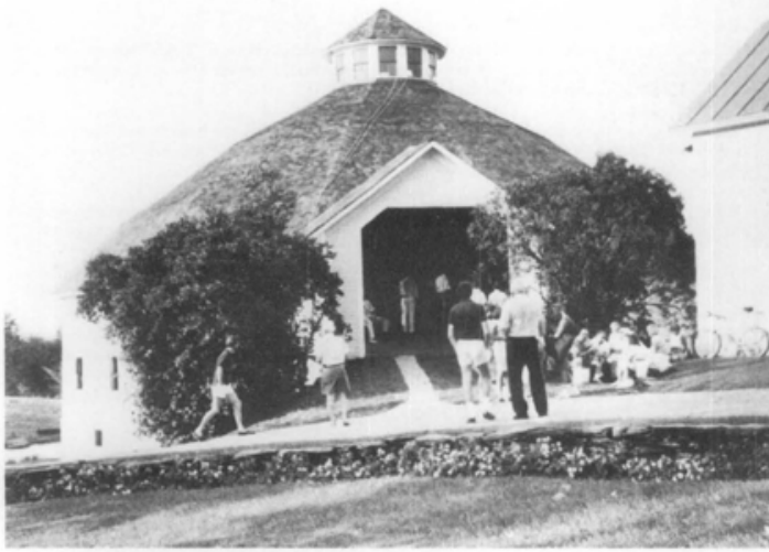
Fig. 10. This 1910 Vermont round barn is 80 feet in diameter. Disused and decaying, the building was converted to a community center, with artists' studios and spaces for weddings, parties and conferences. The barn underwent extensive structural repair and other work. Careful selection of new use permitted the building to be rehabilitated while retaining its principal spaces and features—and its historic character—intact. Photos: Jay White.
