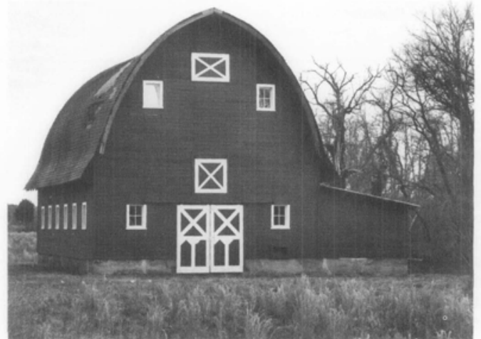
In the early 20th century barn patterns were developed by agricultural schools and prefabricated units were sold by mail-order firms. This Maryland barn was bought about 1920 from a Sears catalogue. Photo: Robert J. Hughes
