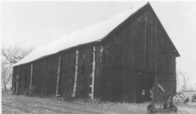
Panels on this 1900 Kentucky tobacco barn open to aid in the curing process. Photo: Christine Amos, Kentucky Heritage Council.
