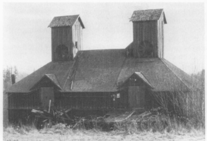
The two ventilating towers are the character-defining aspect of this Oregon hop-drying barn. Photo: Allan Nelson.
