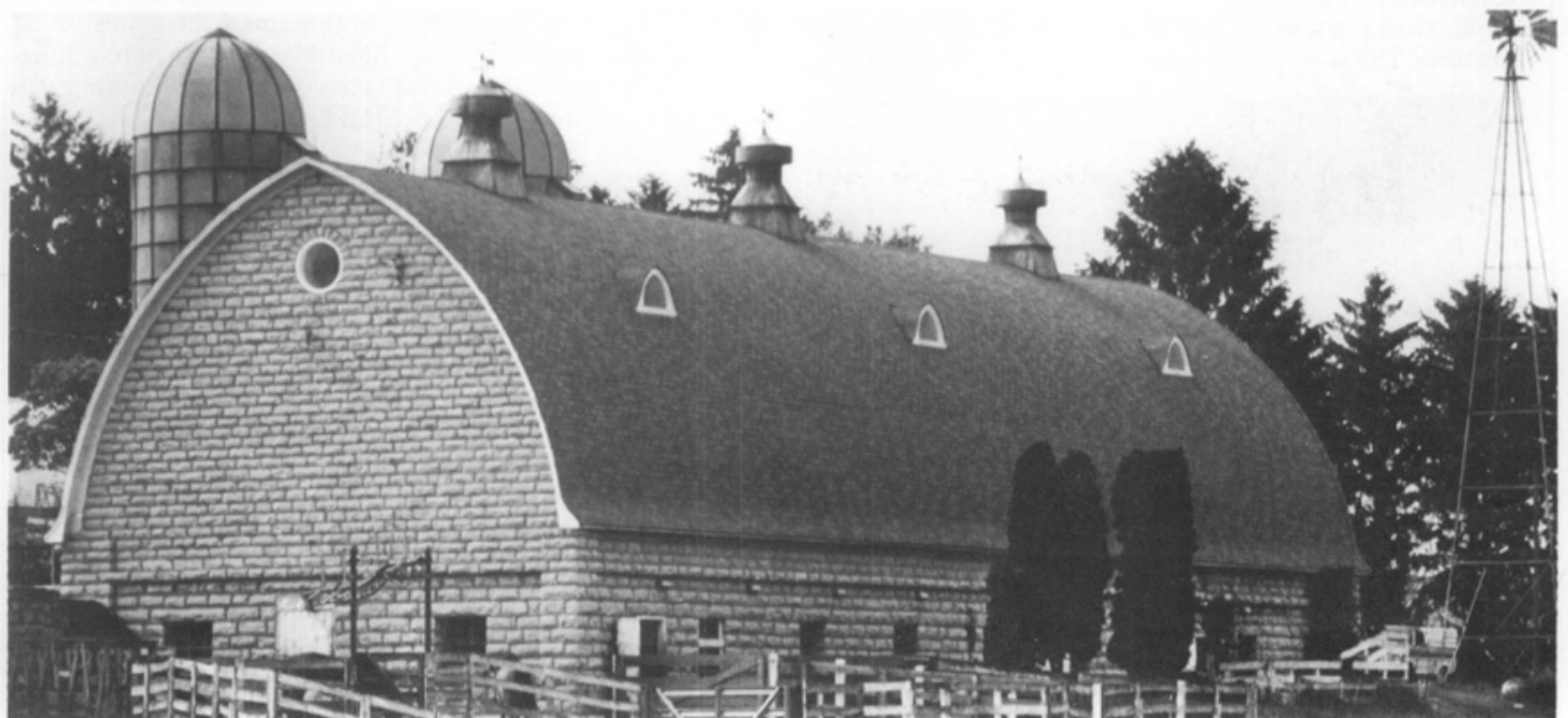
Fig. 1. Arch roof, native limestone walls two feet thick at the base, porthole window, dormers, silos, rooftop ventilators, weathervanes, windmill, fences, fields, and family pride in the builder are all components of the historic character of this Iowa barn. Photo: John Walter, Successful Farming.
