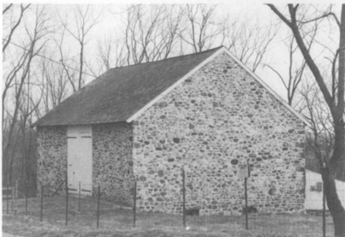
Fig. 3. The stone walls of this Delaware barn are its most notable feature. Built about 1810, the barn is a bank barn. Photo: Valerie Cesna, Delaware Bureau of Archeology and Historic Preservation.
