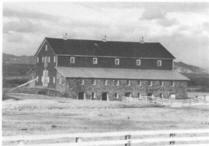
Fig. 2. Mountains, fields, fences, sheds, trees: The setting of this enormous Montana barn is an important element of its character. The barn was built in 1887–1889 after disastrous livestock losses in the winter of 1886–1887. It could hold 500 cattle and store a quarter-million cubic feet of hay. Photo: John N. DeHaas, Jr., Montana Historical Society.
