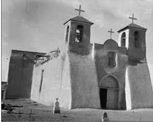
San Francisco de Assisi Mission Church in Rancho de Taos, NM, was constructed of adobe between 1772 and 1819 and, because of its distinctive sculptural quality, is one of the most famous and frequently photographed of the mission churches. Photo: HABS Collection, NPS.
