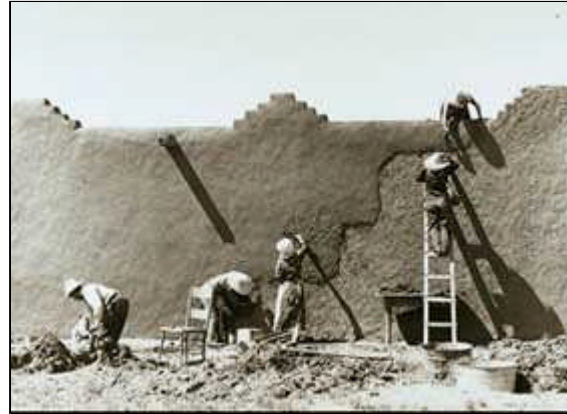
Traditionally, adobe surface coatings that protected the fragile adobe building fabric were renewed every few years. Women are seen here recoating an adobe wall with mud plaster mixed with straw at Chamisal, New Mexico. Photo: Russell Lee, Farm Security Administration Collection, Library of Congress.
