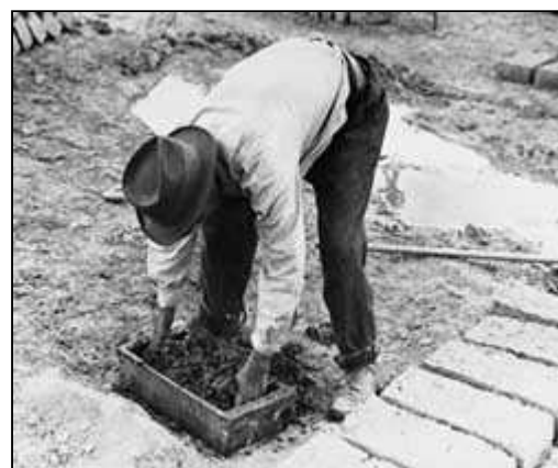
A mixture of mud and straw is pressed into a mold to form an adobe brick. After the adobe brick is removed from the mold, it must dry in the open air for a month or more before it can be used. Photo: Russell
