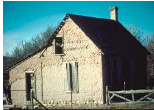
A traditional mixture of mud and straw plaster should be applied to stabilize the exterior of this house. Photo: NPS files.
