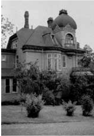
Special problems inherent in the design of an elaborate historic roof can be controlled through regular maintenance. The shape and detailing are essential elements of the building's historic character, and should not be modified, despite the use of alternative surface materials. Photo: NPS files.
