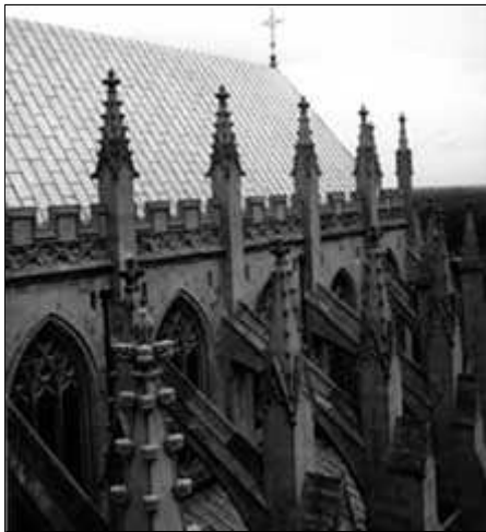
Good design and quality materials for the roof surface, fastenings, and flashing minimize failures. Photo: NPS files.
