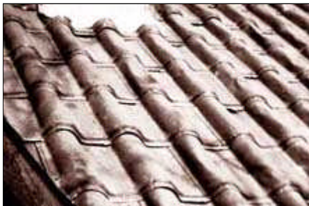
Galvanized sheet-metal shingles imitating the appearance of pantiles remained popular from the second half of the 19th century into the 20th century. Photo: NPS files.
