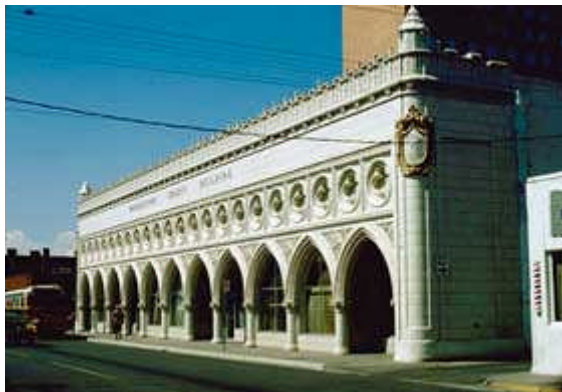
Glazed architectural terra-cotta was a practical and highly decorative building material. Photo: NPS files.
