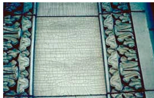
Water and air-borne moisture entering the glazed architectural terra-cotta causes expansion of the porous clay body, increasing its volume. This upsets the "fit" of the glaze and makes its surface shatter, which is commonly called "crazing." Photo: NPS files.
