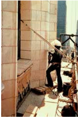
A worker cleans out mortar joints in preparation for repointing the architectural terra-cotta Photo: NPS files.
