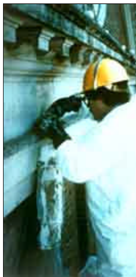
The chemical poultice-type paint remover uses a paper backing that keeps the lead waste contained for proper disposal. Local laws required containment and neutralization of any after-wash water run off. Photo: NPS files.
