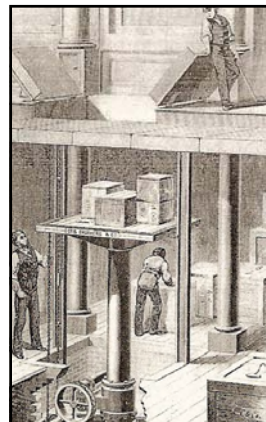
Hydraulic Elevator (Warehouse)
