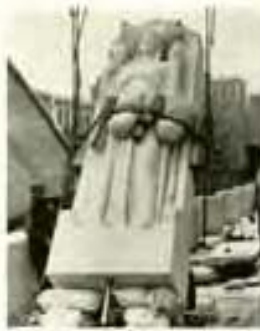
Hoisting a block of Indiana Limestone.
