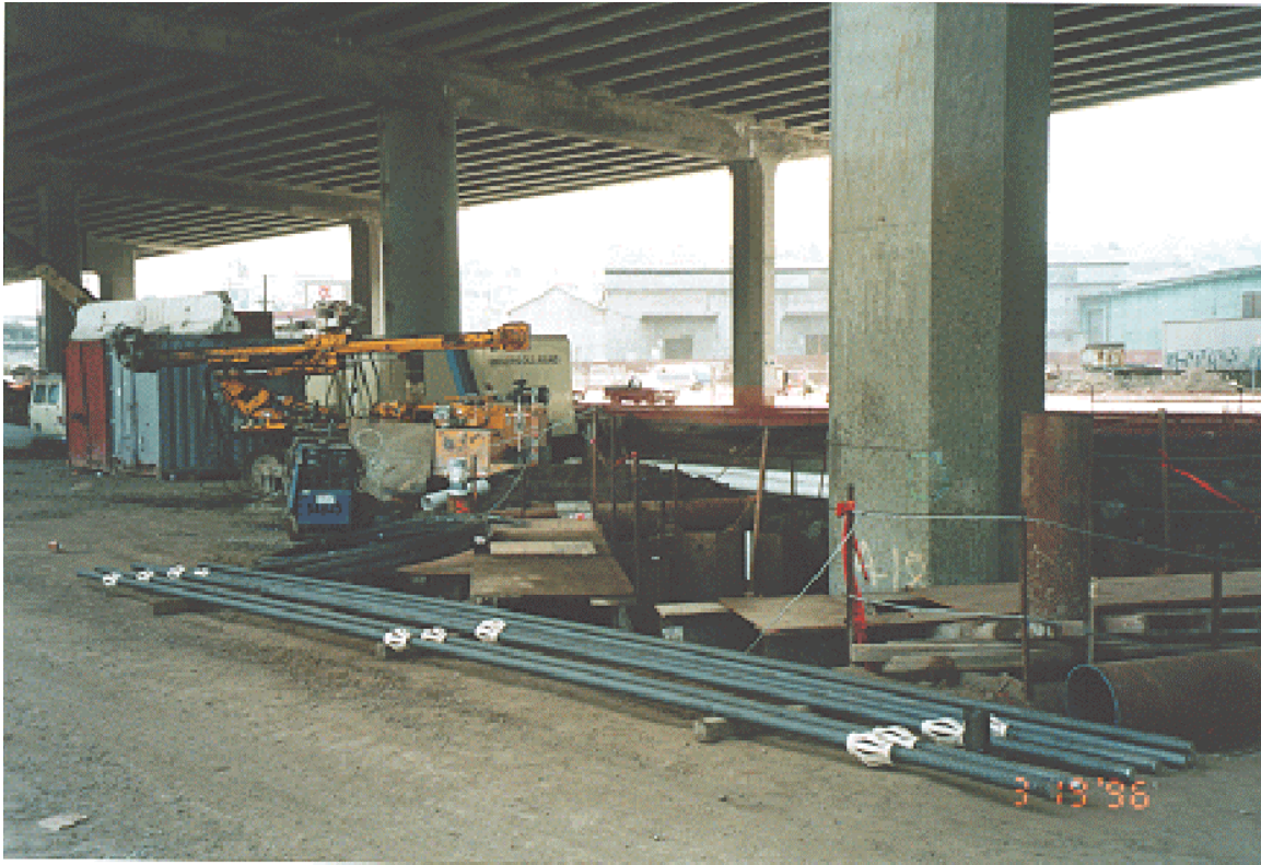
Figure 8-3. Storage of Reinforcing Steel.
