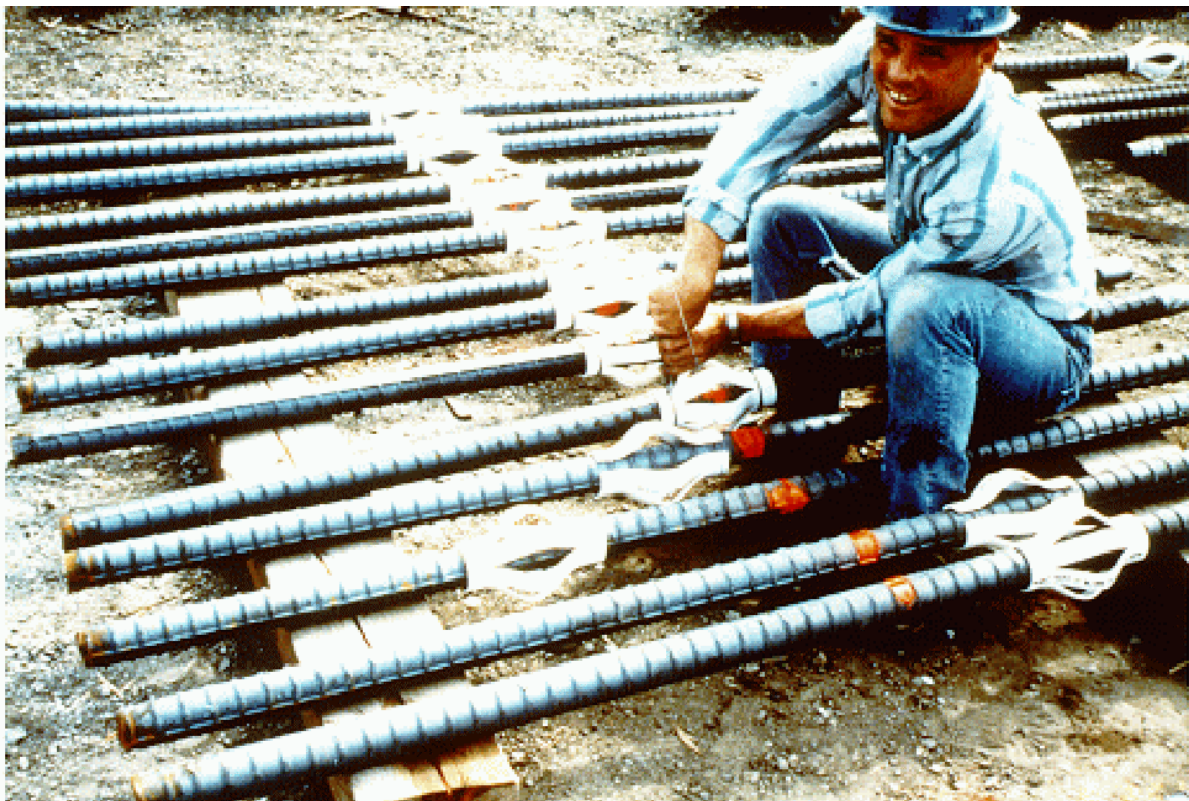
Figure 8-5. Reinforcement Centralizers.
