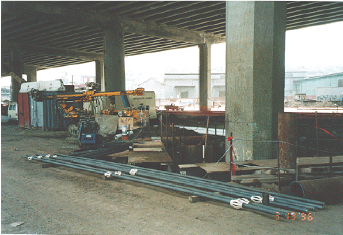
Figure 8-3. Storage of Reinforcing Steel.
