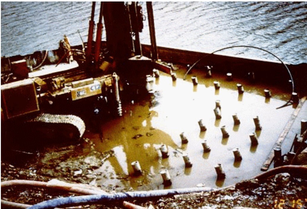
Figure 3-4. Micropiles Used Under New Abutments for Bridge Over Mahoning Creek, Armstrong County, PA (after Pearlman and Wolosick, 1992).
