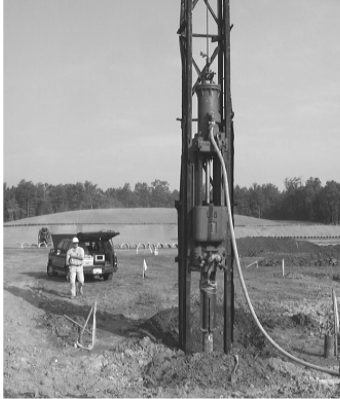
Figure 7-12. Dynamic Test Set-Up for Micropile (after Gomez et al., 2004).
