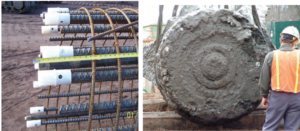
Figure 8-17 Chairs for Base of Reinforcing Cage
