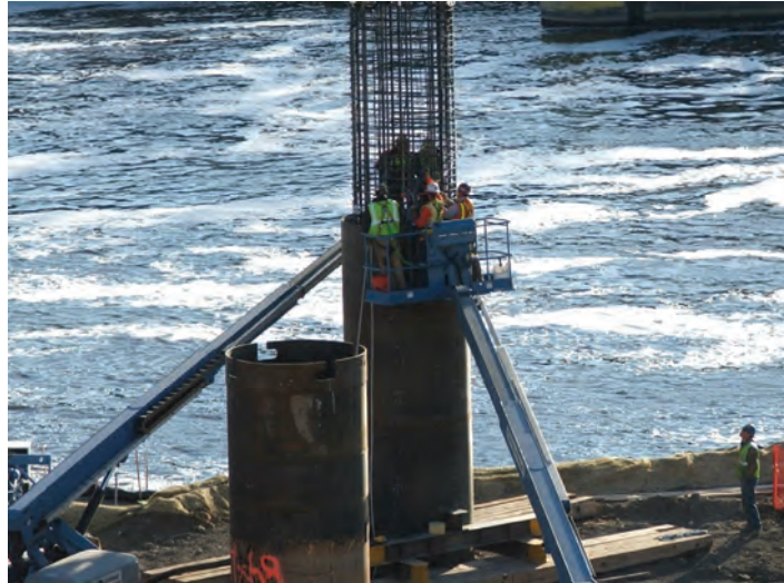
Figure 4-16 Use of Surface Casing to Overcome Artesian Groundwater
