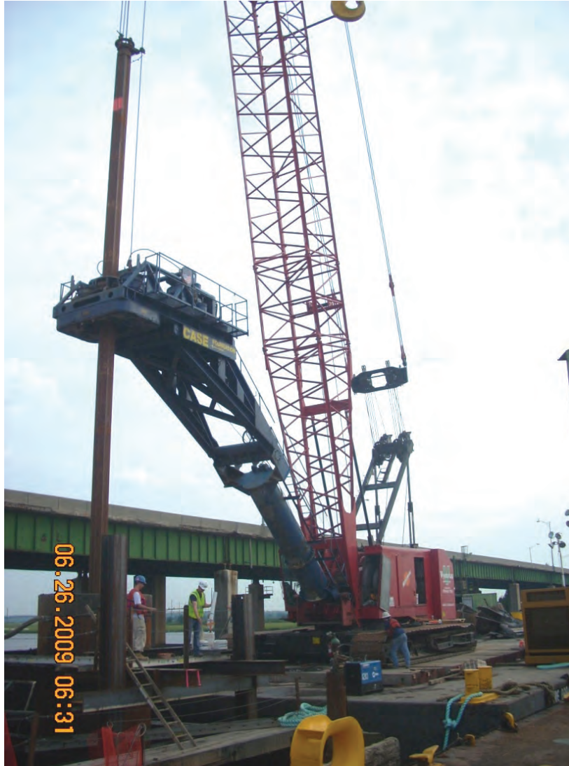
Figure A-12 Crane-Mounted Drilling Machine for Construction Over Water (Photo courtesy of Paul Axtell)
