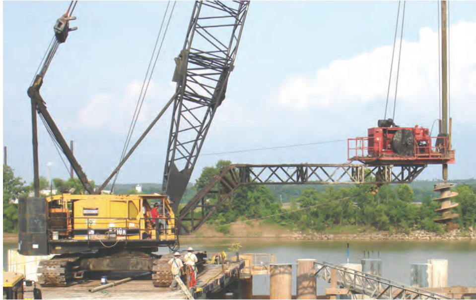
Figure 5-5 Crane Mounted Drilling Rig
