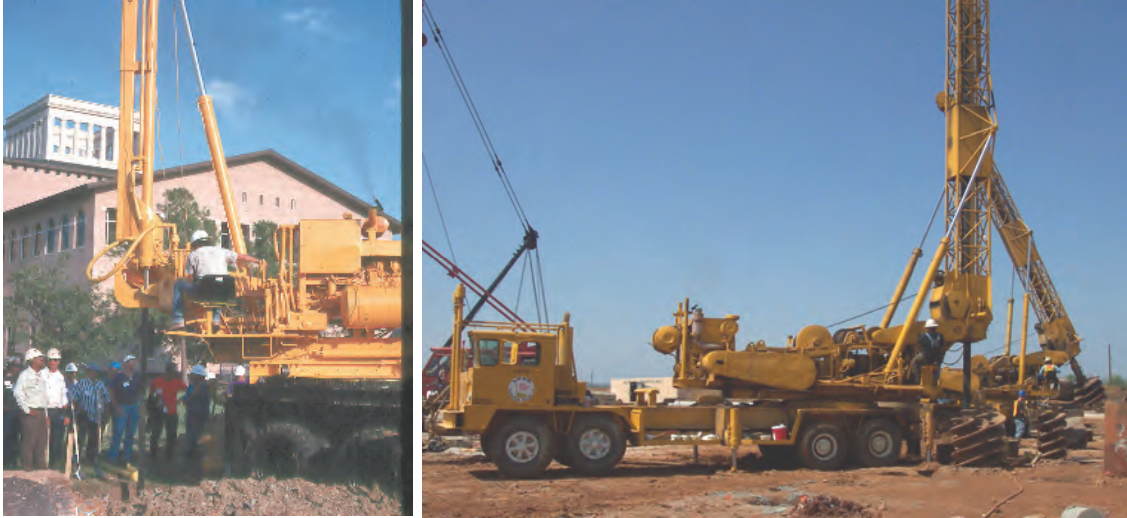
Figure 5-4 Truck Mounted Drilling Rigs
