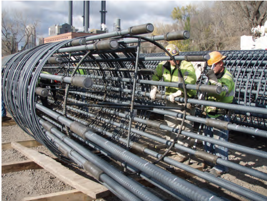
Figure 8-1 GR75 Reinforcement Cage Being Assembled, Showing Threaded Couplers
