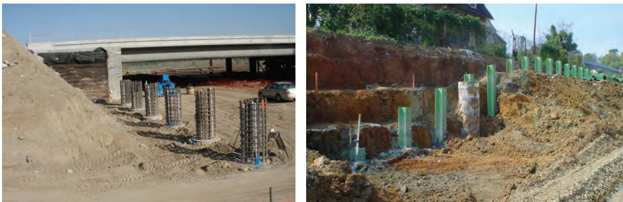
Figure 1-17 Drilled Shafts Used to Support Earth Retaining Structures
