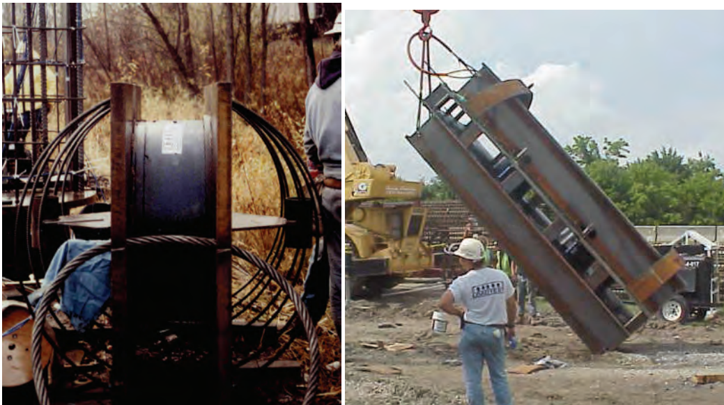
Figure 17-59 Bi-directional Lateral Testing Apparatus Using Embedded O-cells
