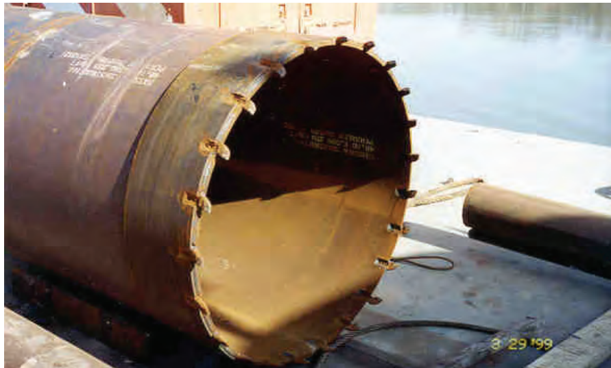
Figure 4-11 Cutting Teeth on the Casing to Assist Penetration into the Bearing Stratum
