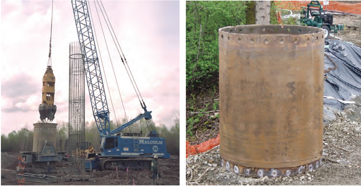
Figure 6-3 Segmental Casing Installation with Oscillator System
