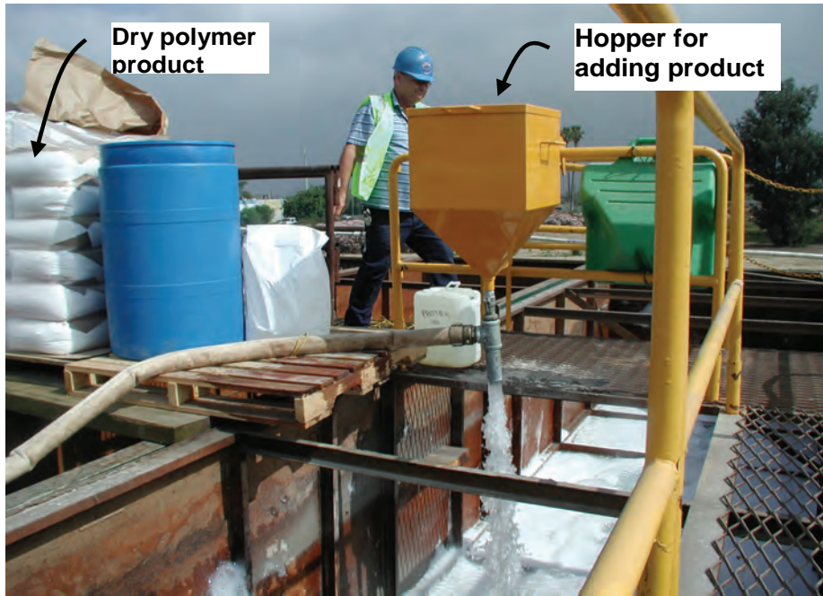
Figure 7-6 Field Mixing Polymer Slurry by Circulating Between Tanks
