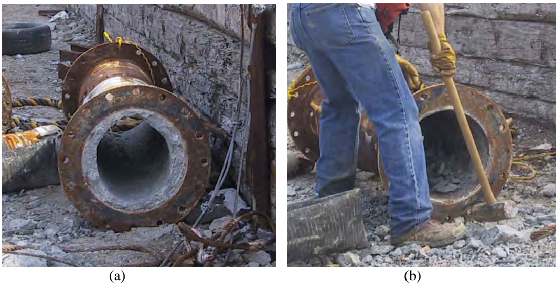
Figure 9-7 Tremie Must be Clean; (a) Tremie Contaminated with Hardened Concrete; (b) Worker Cleaning Tremie
