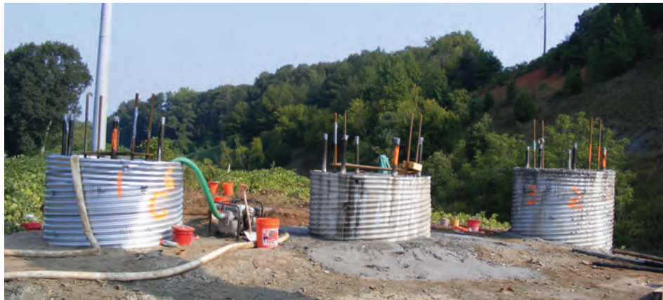
Figure 6-16 Corrugated Metal Pipe (CMP) Used as Permanent Liner
