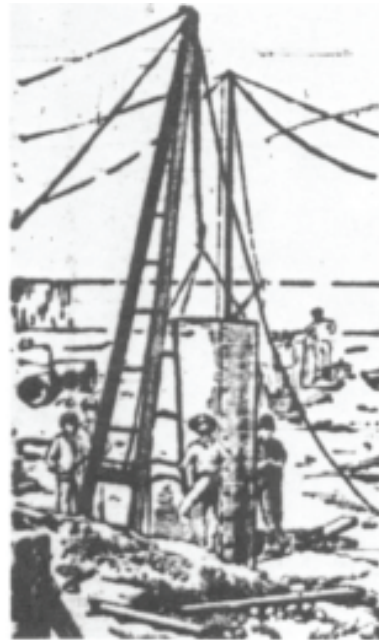
Figure 1-5 “Caisson” Foundation Construction in Kansas City (Hoffmann, 1966)
