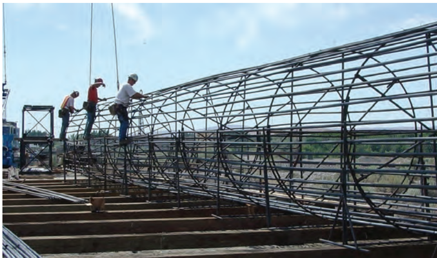
Figure 8-2 View of a Rebar Cage Being Assembled, Showing Longitudinal Steel
