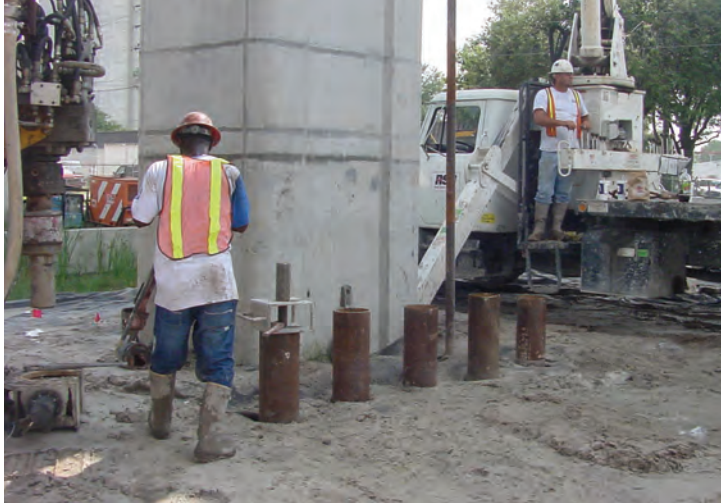
Figure 21-6 Use of Micropiles to Supplement an Existing Foundation (McGillivray and Brown, 2007)
