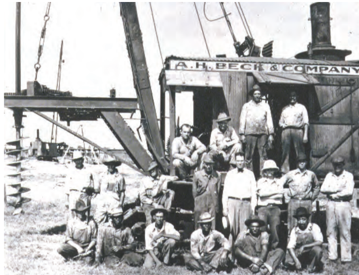
Figure 5-1 An Early Drilled Shaft Machine and Crew
