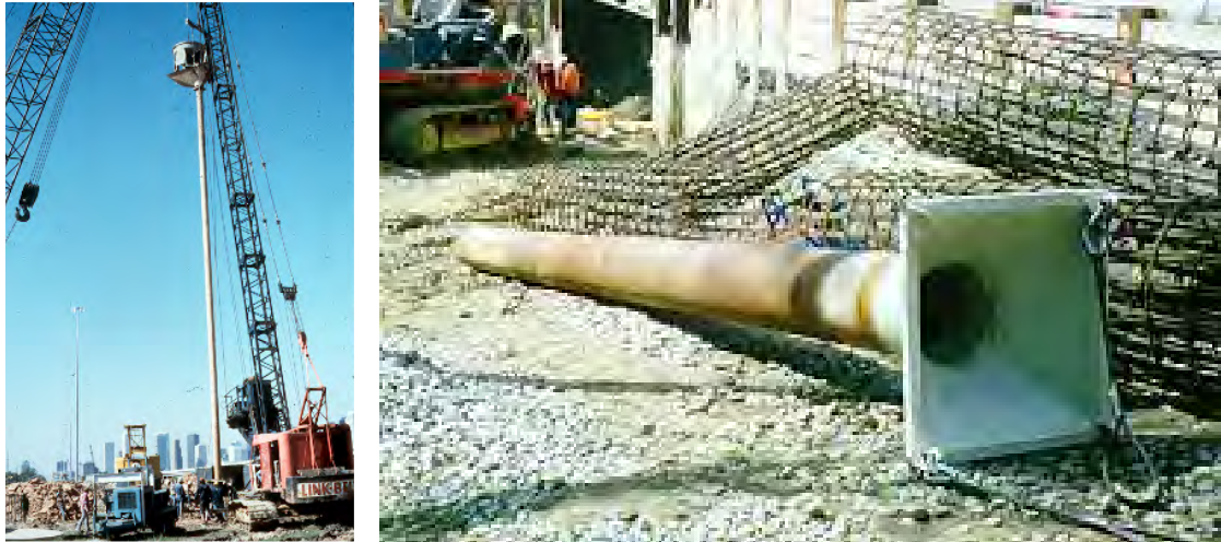
Figure 9-8 Solid Tremie Pipes
