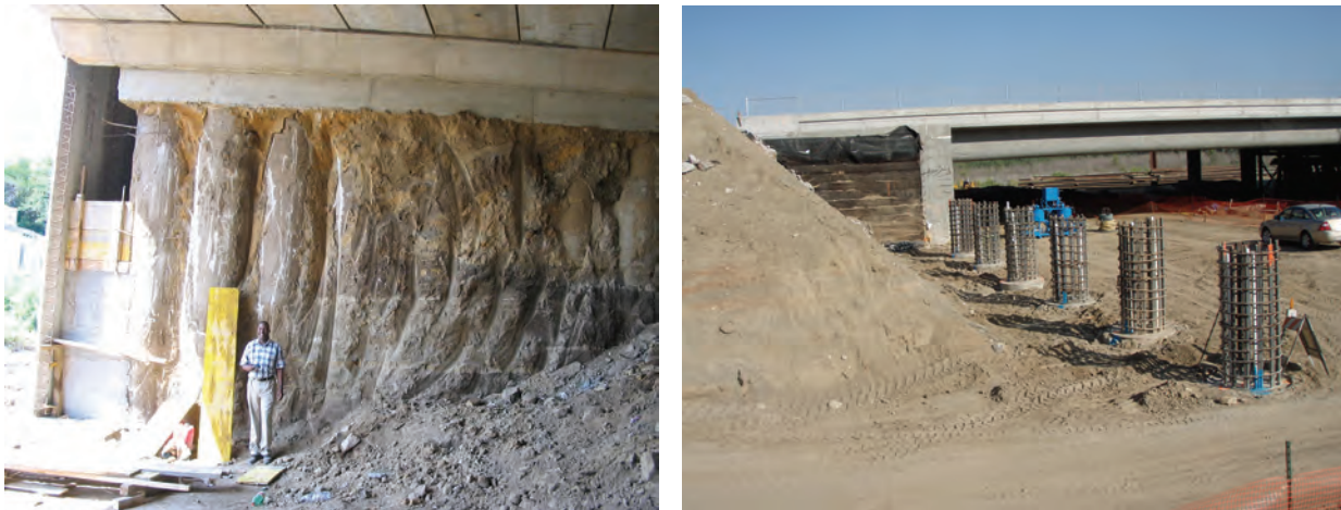
Figure 12-7 Drilled Shaft Abutment Foundations
