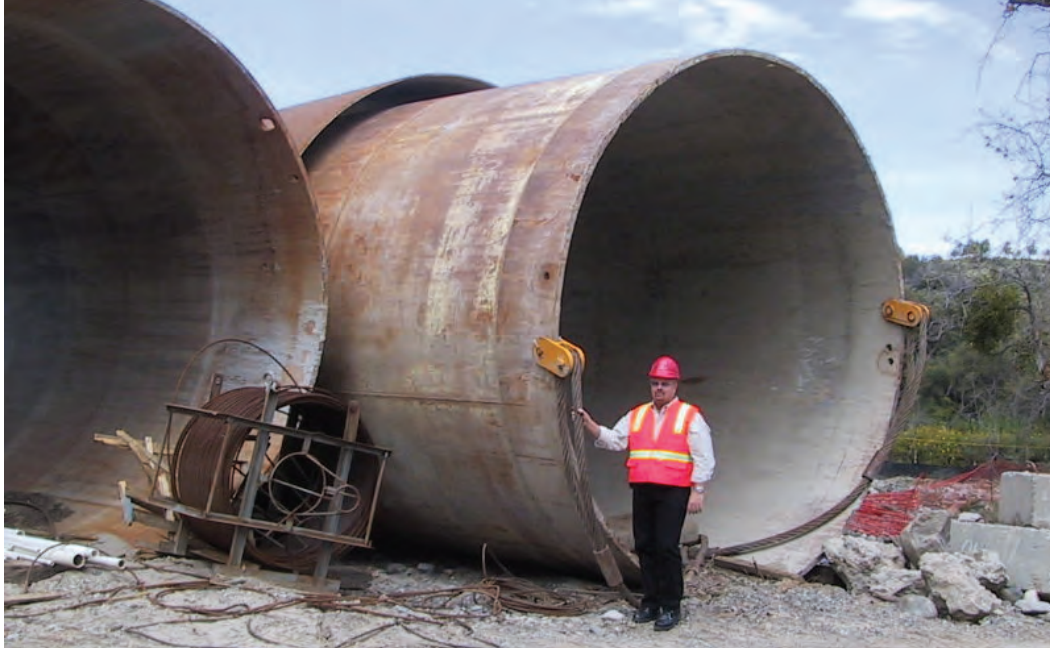
Figure 6-2 Exceptionally Large Temporary Casings
