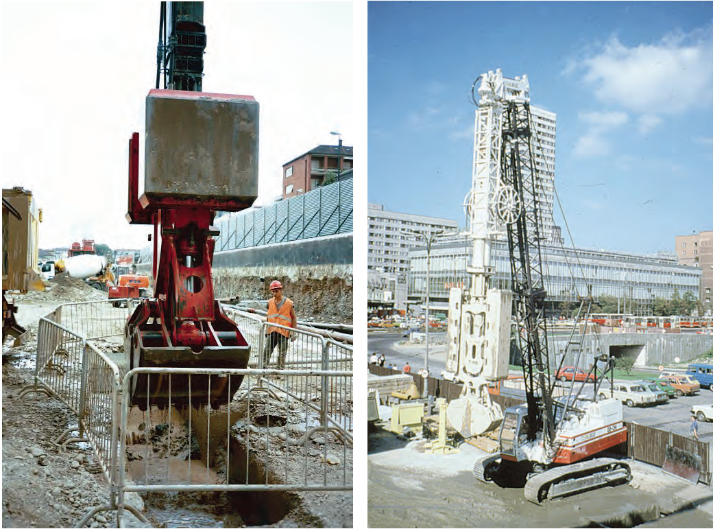
Figure 5-13 Excavation of a Diaphragm Wall or Barrette Using a Clam
