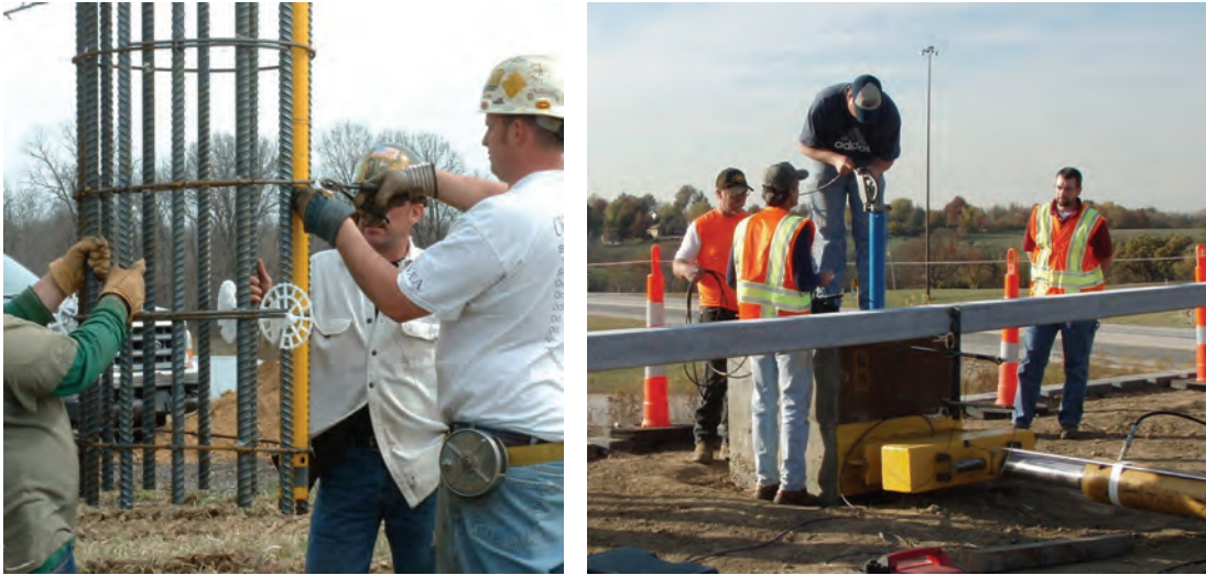
Figure 17-62 Measurements of Lateral Displacement in a Lateral Test Shaft below Grade Using an Inclinometer
