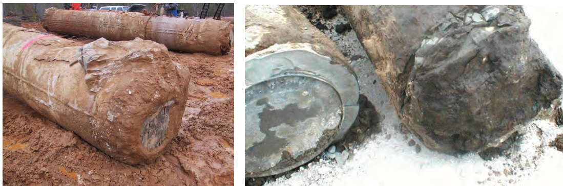
Figure 4-23 Exhumed Shafts after Grouting
