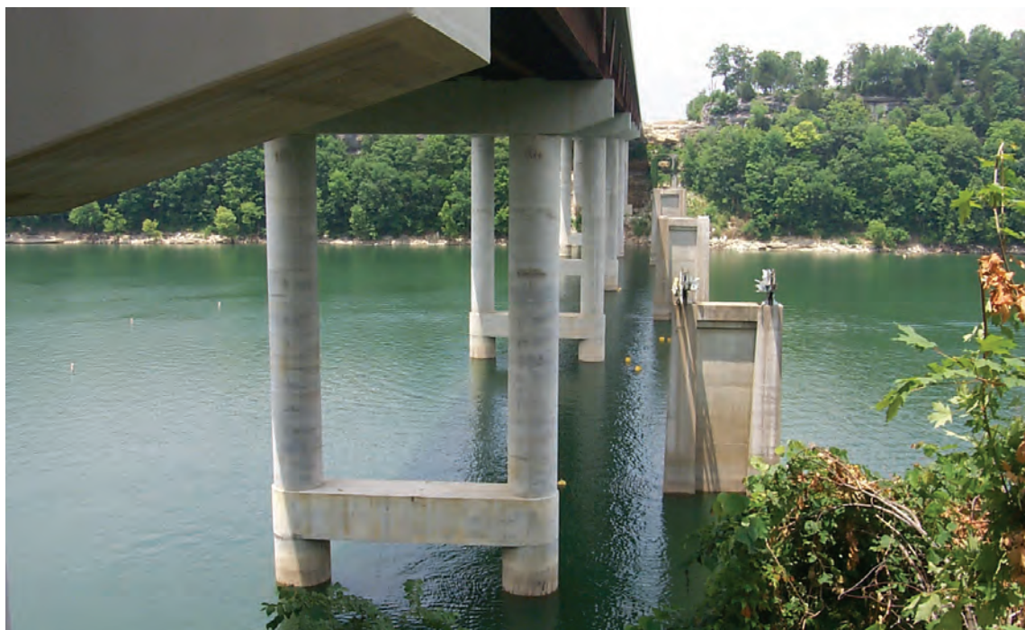
Figure 12-4 Drilled Shafts for Bridge Over Water, Somerset, KY
