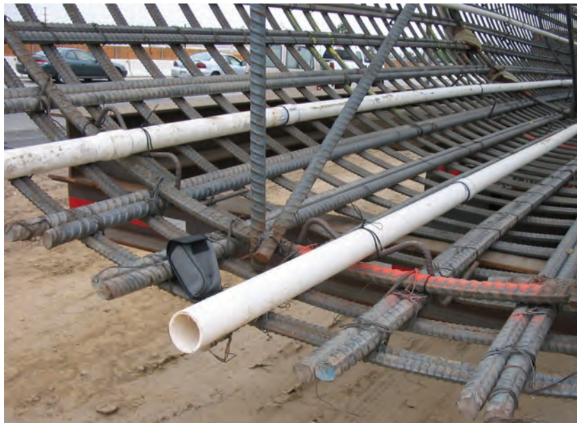
Figure 8-19 Transverse Stiffeners Attached with Tack-Welds to Sizing Hoops
