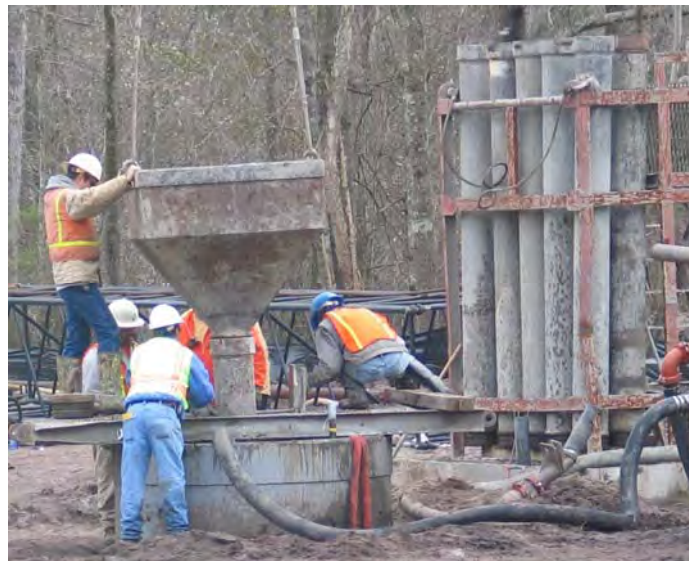
Figure 9-9 Assembly of Segmental Tremie for Concrete Placement
