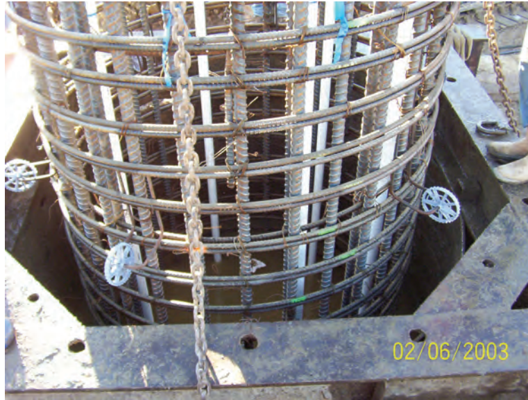
Figure 8-7 Bundled Hoops Used to Improve Flow of Concrete through Transverse Reinforcement
