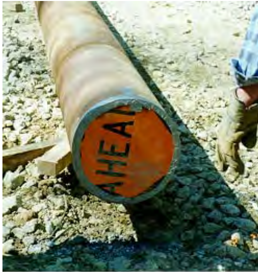
Figure 9-10 Closure Plates for Closed Tremie
