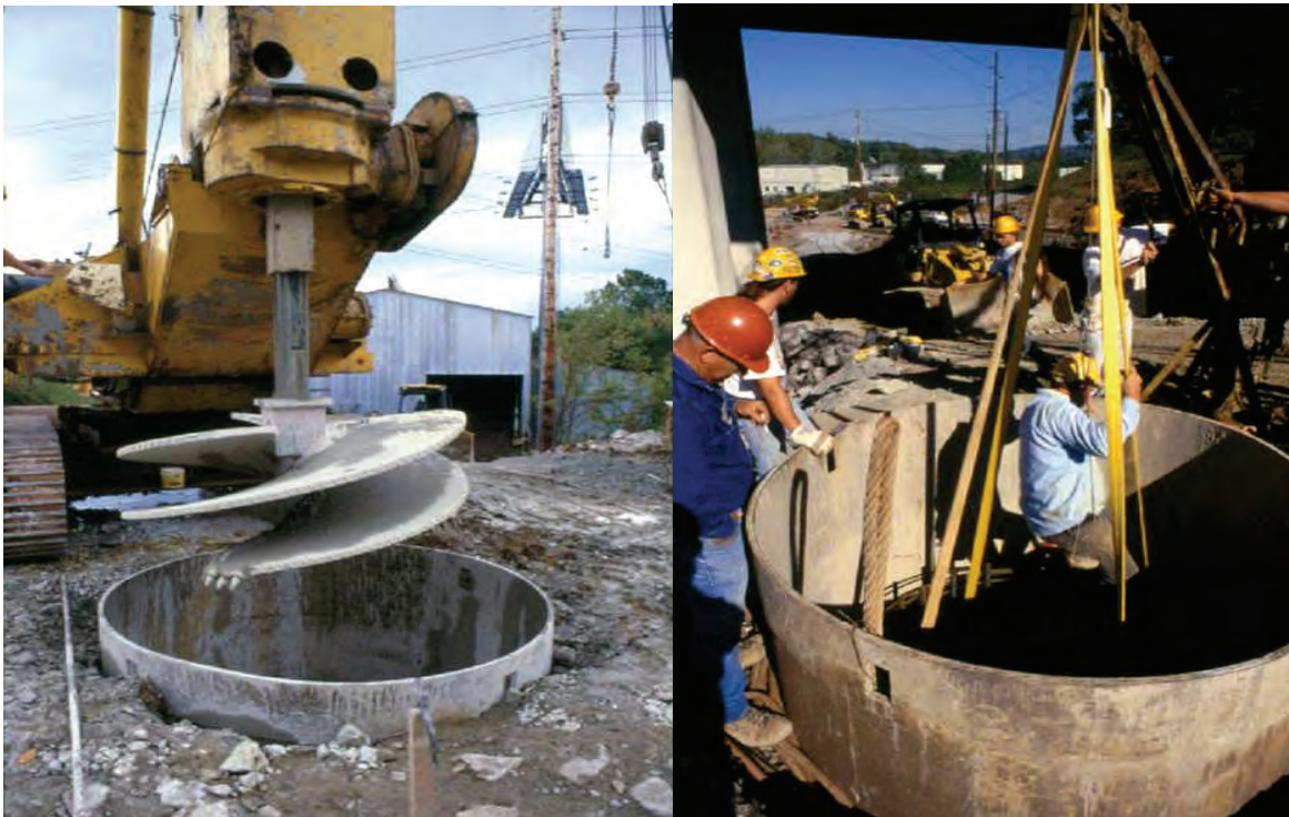
Figure 4-6 Drilling into Rock through a Cased Hole
