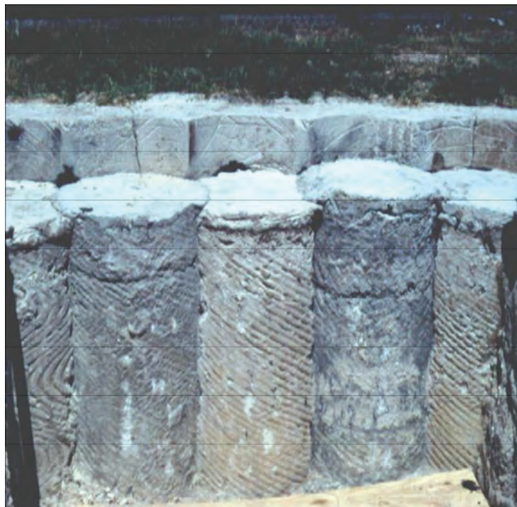
Figure 6-11 Exposed Surface of Drilled Shafts Constructed Using Oscillated and Rotated Casing
