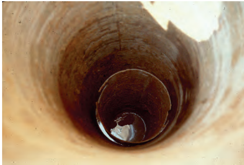
Figure 4-13 Telescoping Casing
