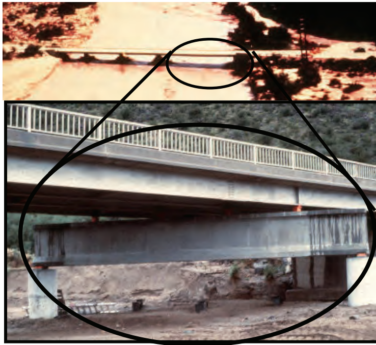
Figure 1-14 Drilled Shafts Installed for Deep Scour Problem
