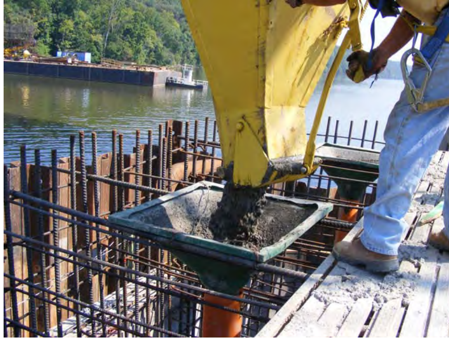
Figure 9-2 Placement into a Dry Excavation Using a Drop Chute
