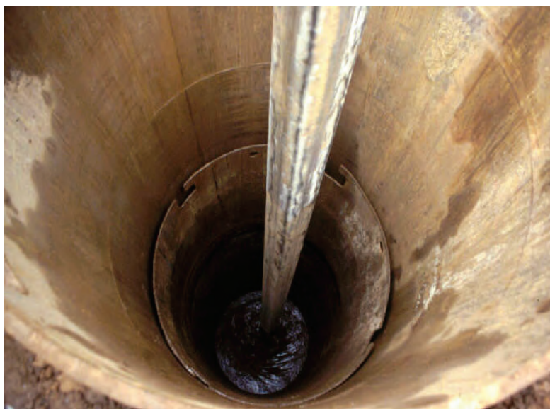
Figure 6-7 Use of Telescoping Casing
