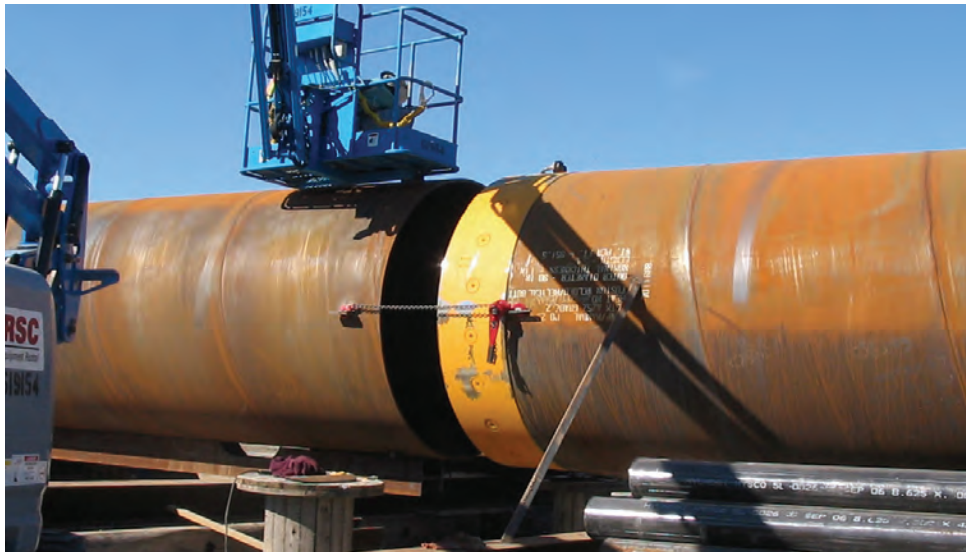
Figure 6-4 Installation of Casing Joint on Standard Pipe
