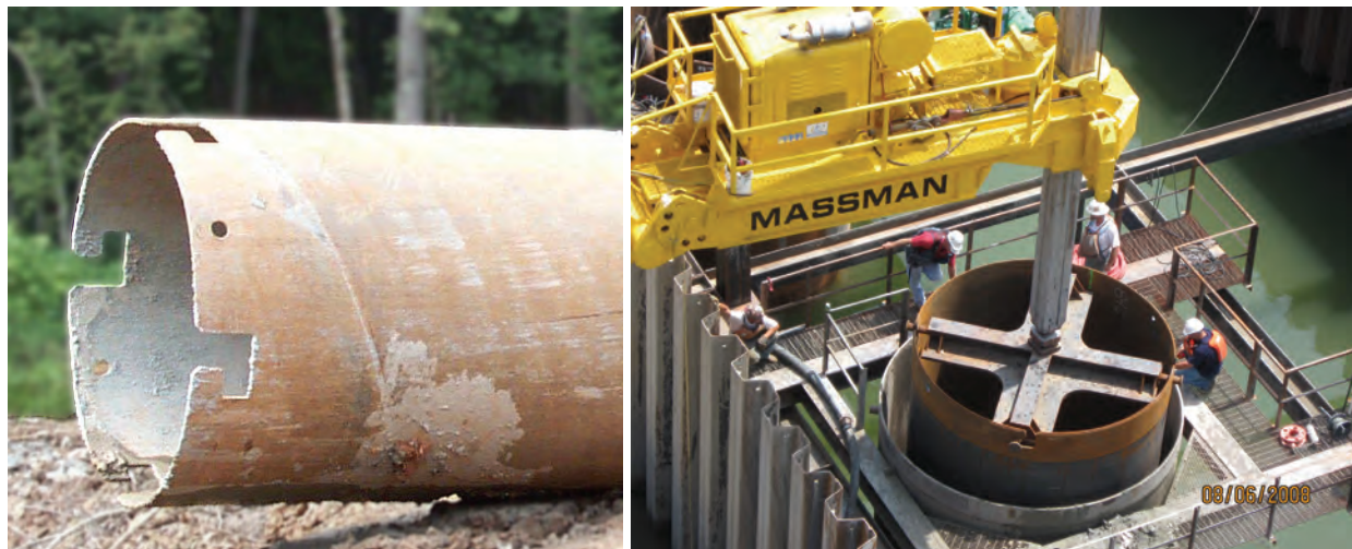
Figure 6-5 J Slots in Top of Casing for Use with Casing Twister
