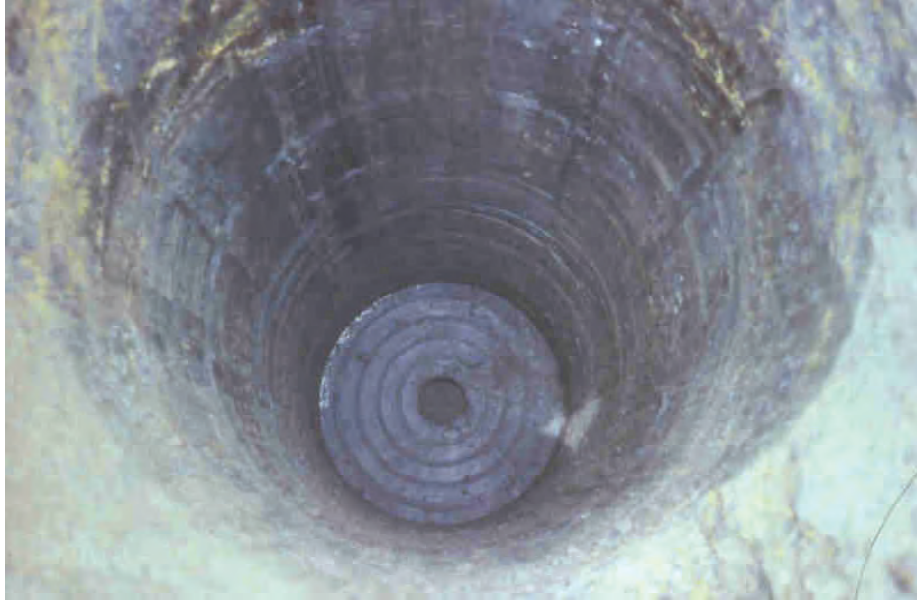
Figure 4-1 Dry Hole in Stable Soil
