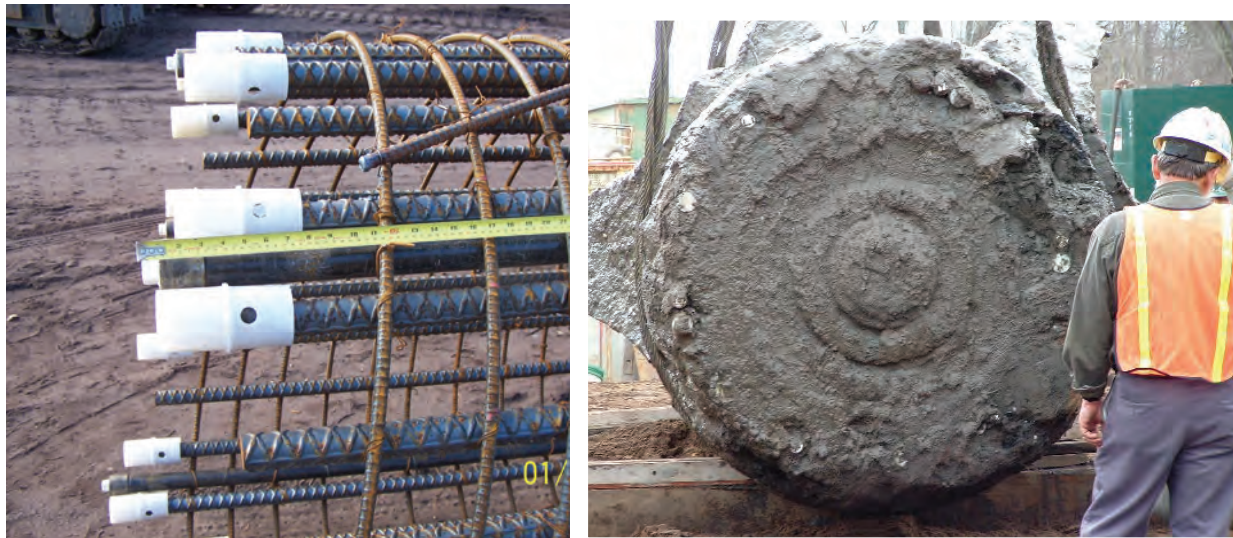
Figure 8-17 Chairs for Base of Reinforcing Cage
