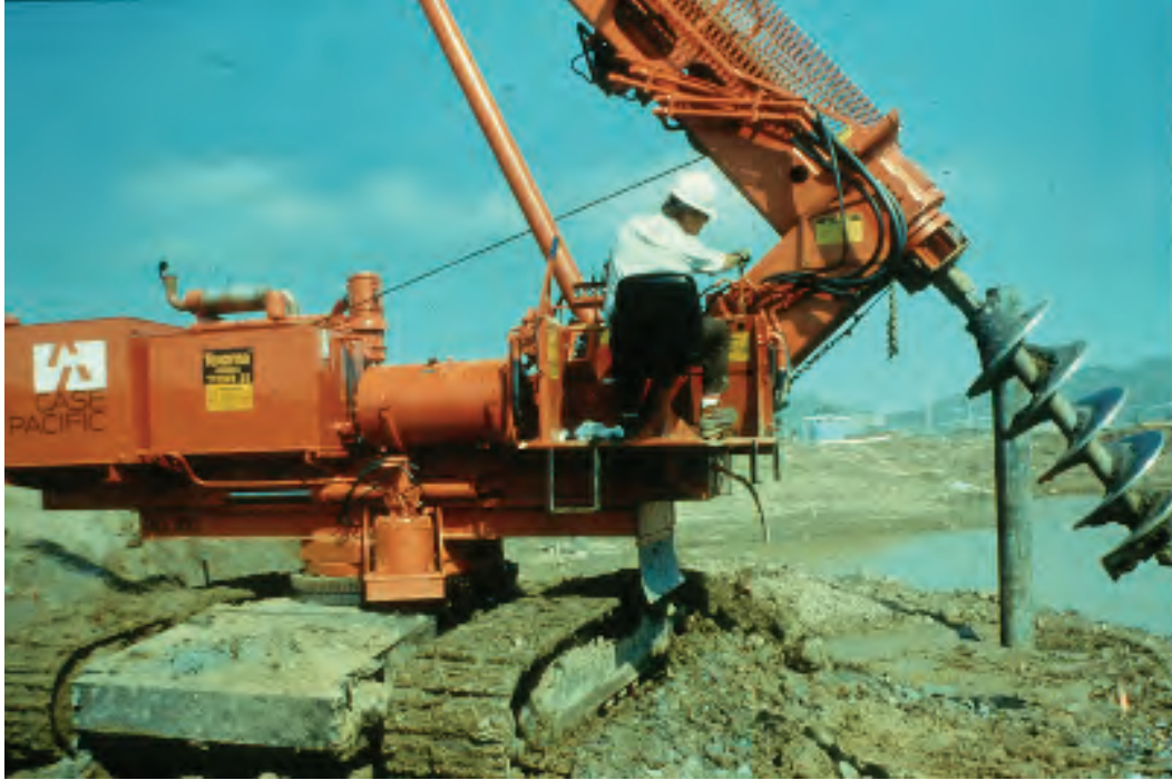
Figure 5-6 Crawler Mounted Drilling Rig
