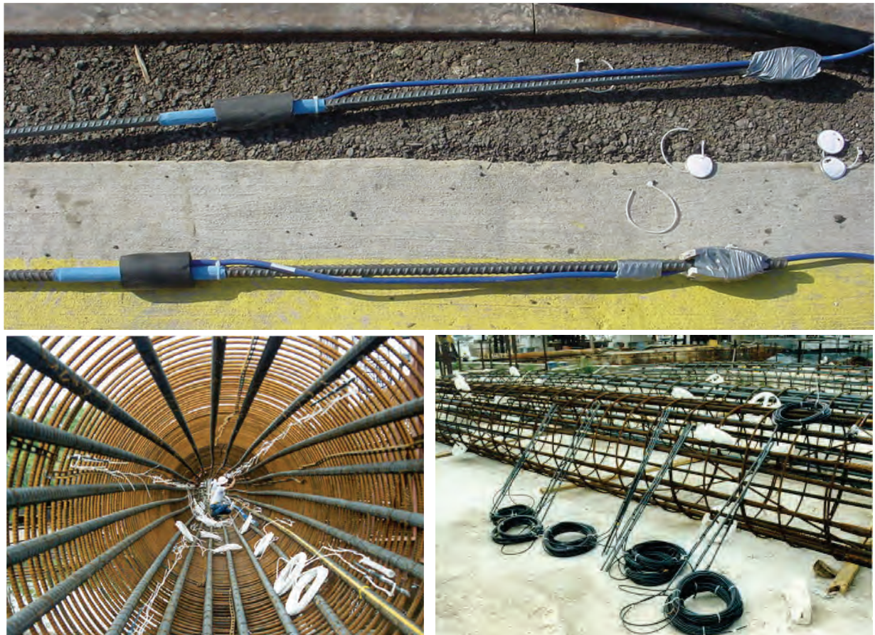
Figure 17-48 Sister-bar Mounted Strain Gauges Placed in Drilled Shaft Reinforcement
