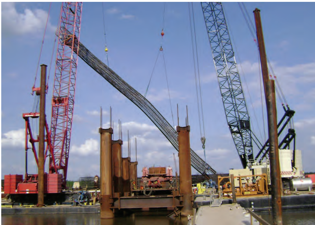
Figure 8-21 Photograph of Rebar Cage Being Lifted Properly
