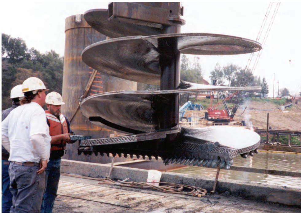
Figure 5-17 Large Diameter Auger with Double Cutting Edge
