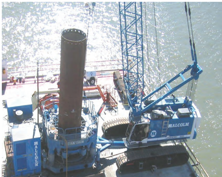
Figure 5-9 Rotator Machine
