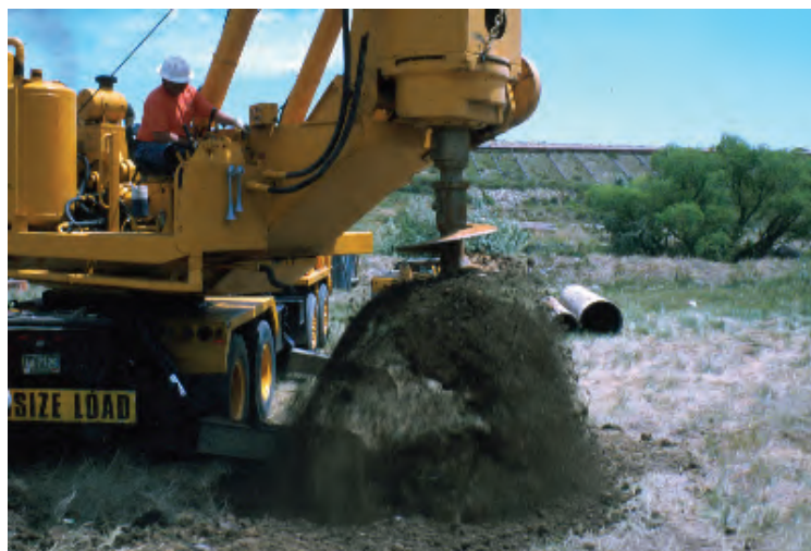
Figure 4-2 Cuttings from a Dry Hole Spun off the Auger
