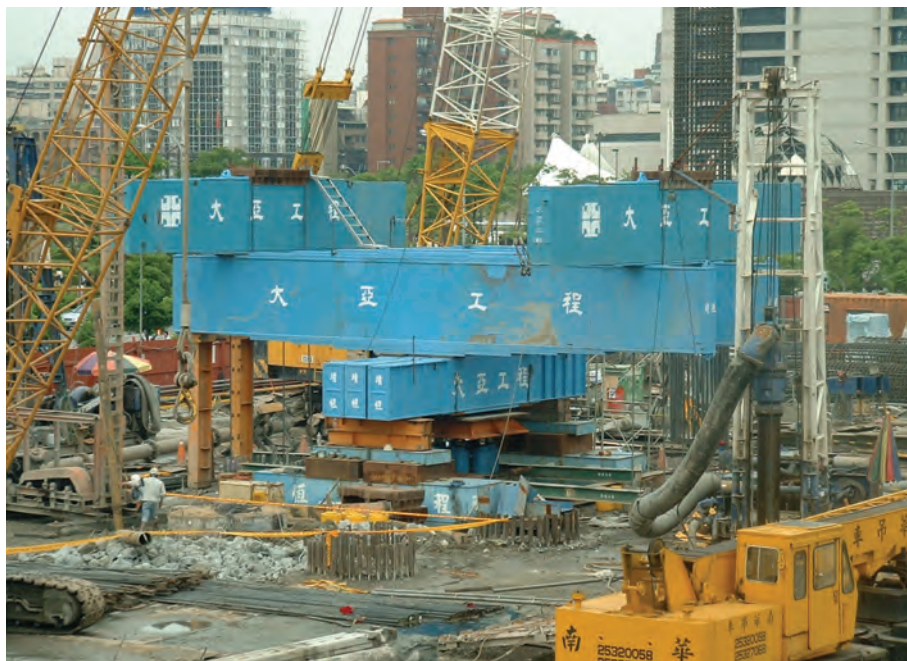
Figure 17-11 5,700 ton Capacity Load Test in Taiwan (photo courtesy Prof. San-Shyan “Sonny” Lin)
