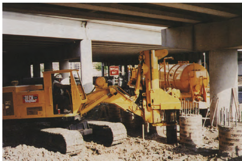
Figure 1-15 Drilled Shafts with Low Headroom
