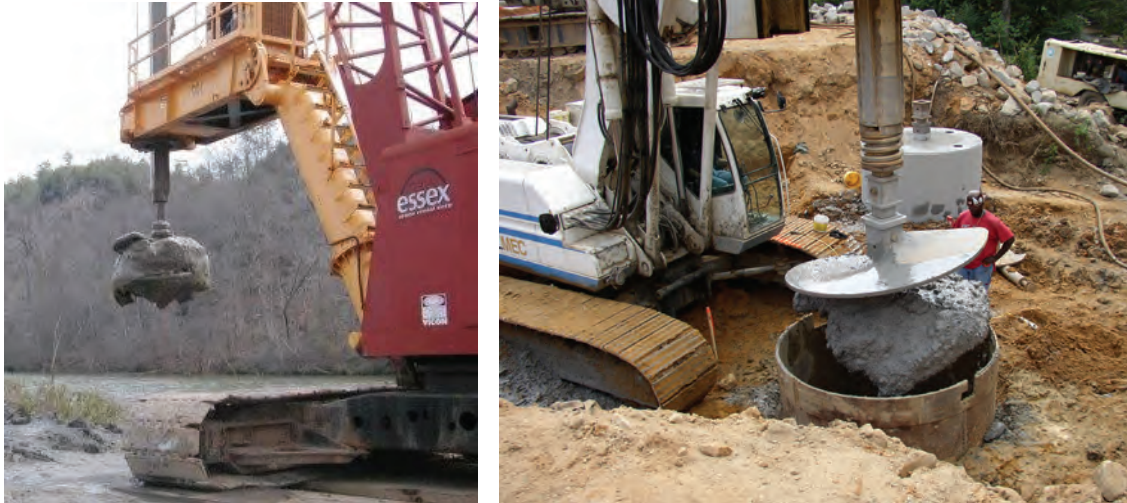
Figure 1-8 Typical Modern Drilled Shaft Rigs
