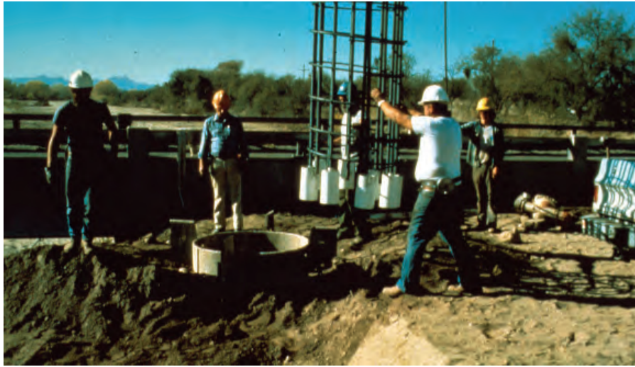
Figure 4-3 Placement of Reinforcing Cage into the Excavation
