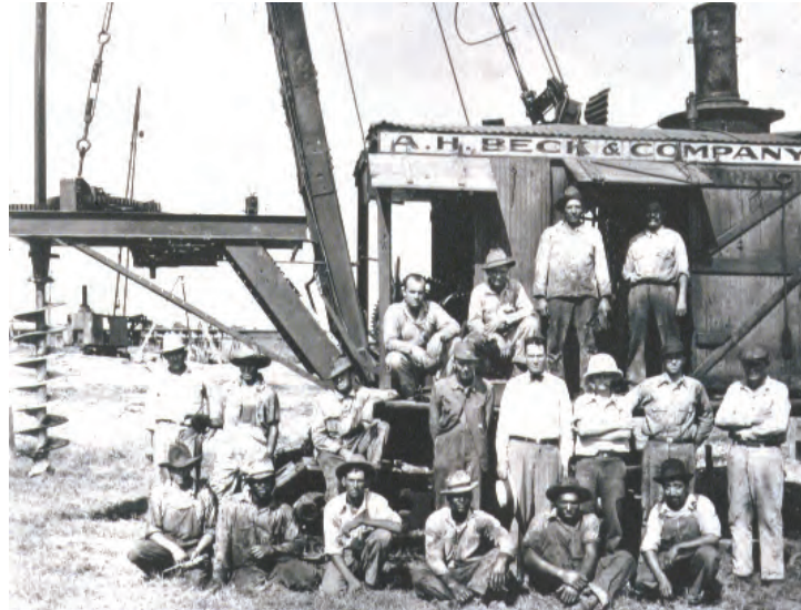
Figure 5-1 An Early Drilled Shaft Machine and Crew
