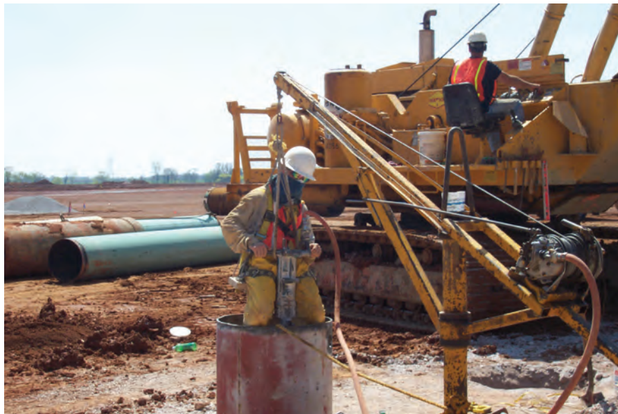
Figure 5-12 Manual Excavation in Rock
