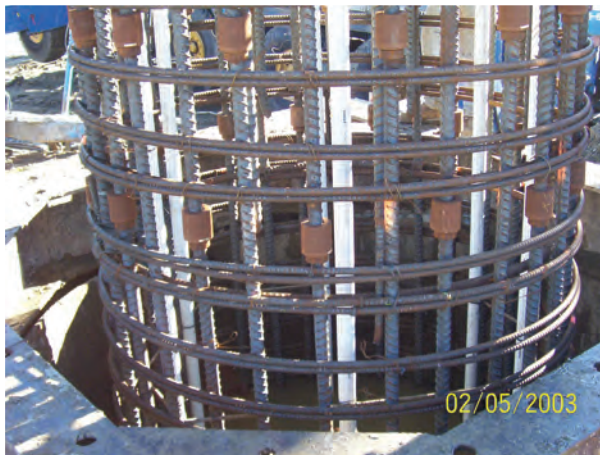
Figure 8-9 Bar Couplers Used to Construct Splices
