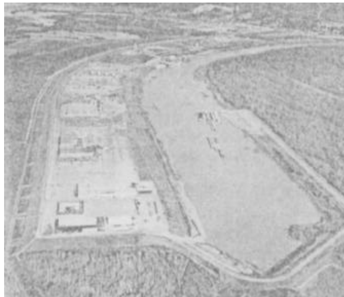
Figure 15-3. The port and industrial park at Vicksburg, Mississippi, which were built from dredged material from the Yazoo River
