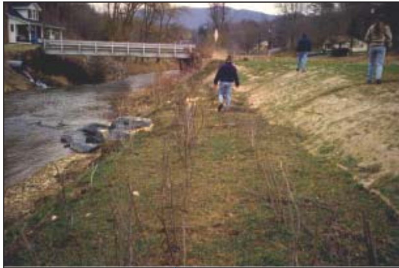
Figure 3.8 Bankfull bench on restoration site
