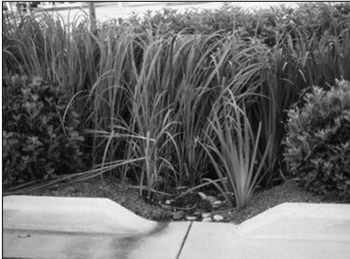
Figure 1.7: Bioretention Curb-cut Entrance
