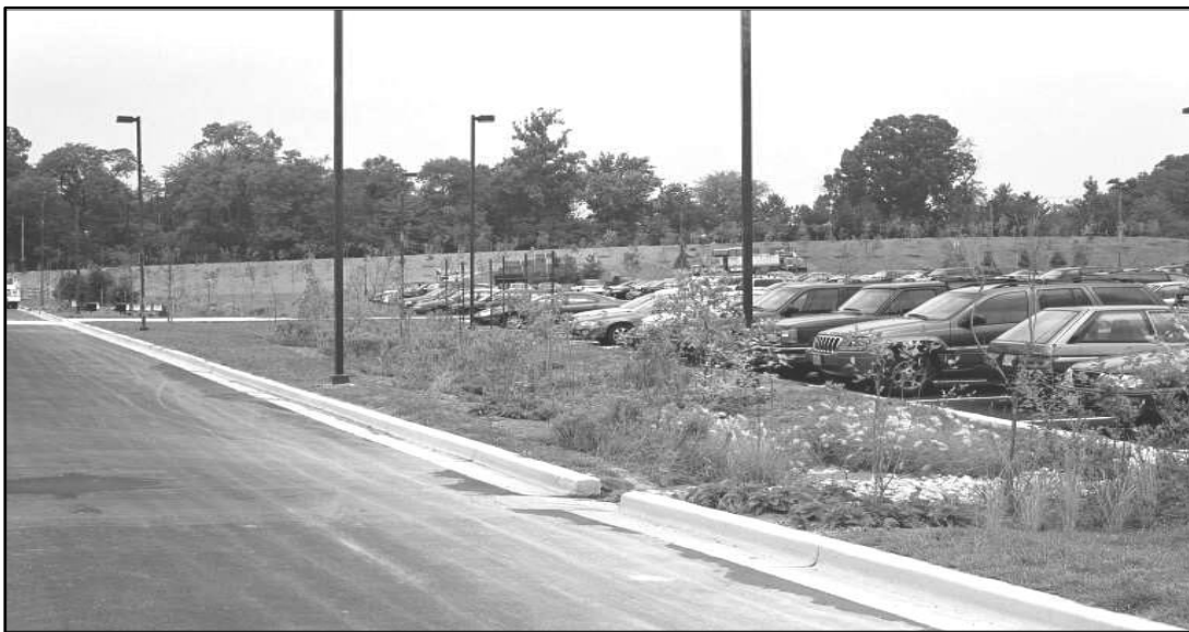
Figure 1.12: Curbed Parking Lot Island & Median Bioretention
