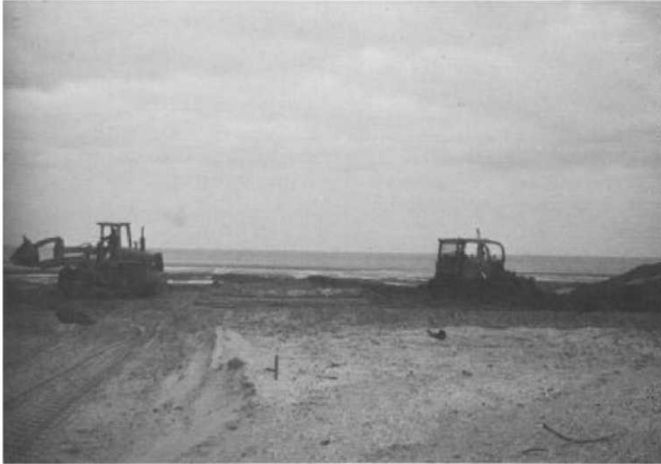
Figure 5-8. Heavy equipment was required to shave down sandy dredged material deposits to intertidal levels at Bolivar Peninsula, Texas, and at other man-made wetland sites
