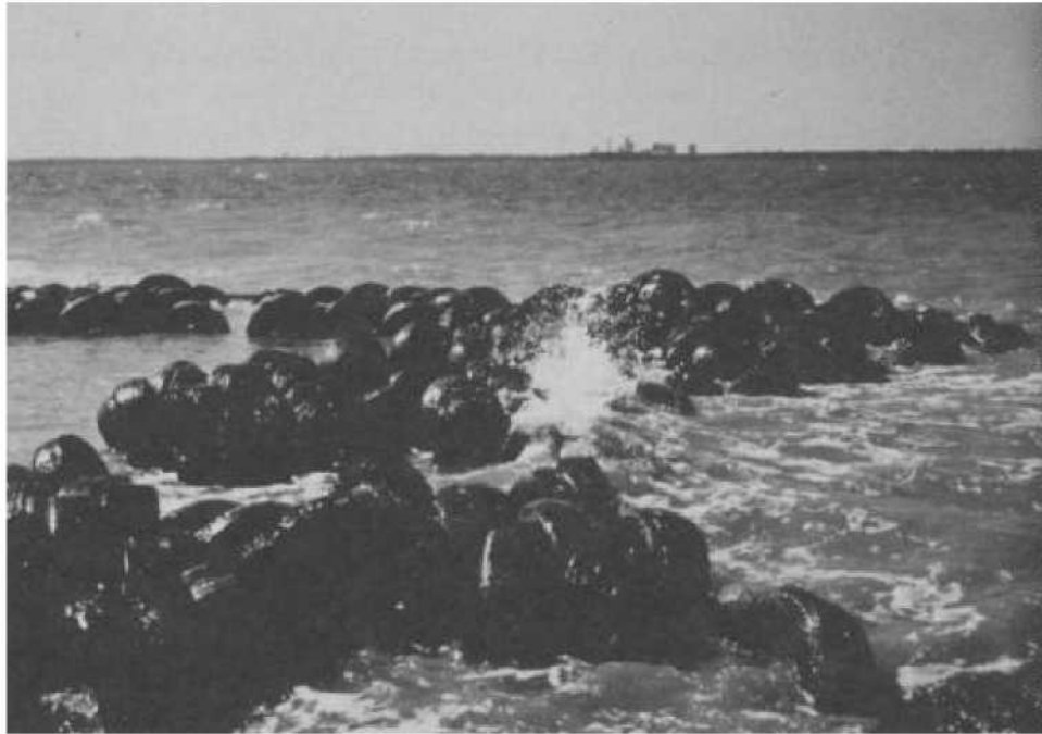
Figure 5-2. A floating tire breakwater installed at Gaillard Island, Alabama, to protect newly planted marsh from moderate wave energies
