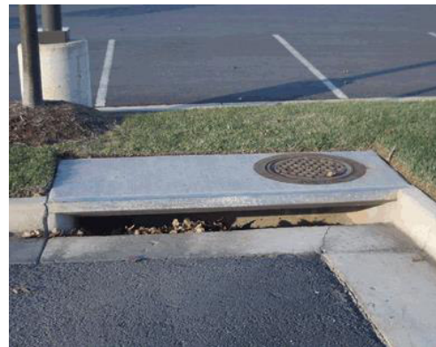
Figure 6 – A Curb-Opening Inlet
