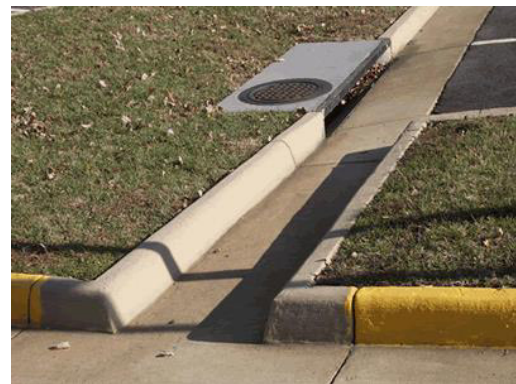
Terminating an Island next to a Curb
