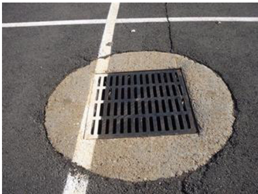
Figure 5 – A Grate Inlet
