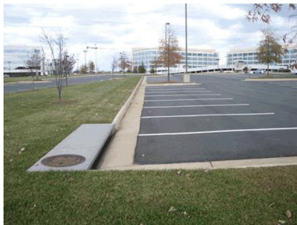
Concrete Curb/Gutter in a Parking Lot
