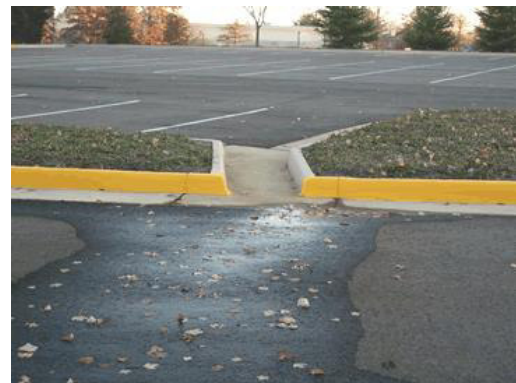
Splitting an Island for Water Passage
