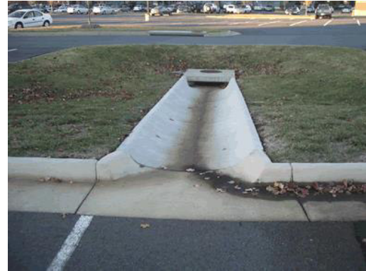
Connecting Two Drainage Systems
