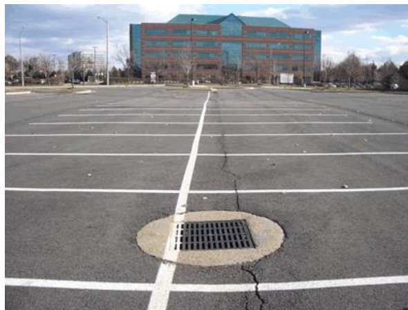
A Parking Lot with Grate Inlets
