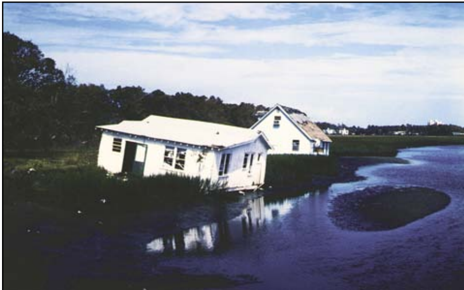
Figure 7-8 Hurricane Hugo (1989), Garden City, South Carolina. Intact houses were floated off their foundations and carried inland.
