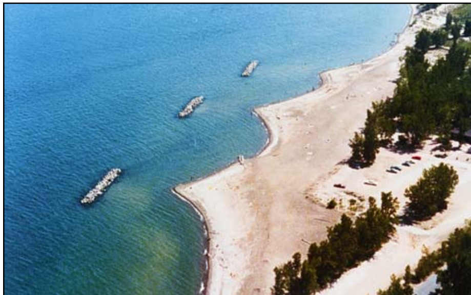
Figure 7-50 Trapping of littoral sediments behind offshore breakwaters, Presque Isle, Pennsylvania. Photograph courtesy of USACE.
