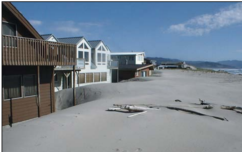
Figure 7-53 Windblown sand drifting against coastal residences in Pacific City, Oregon. Photograph by Jim Good.
