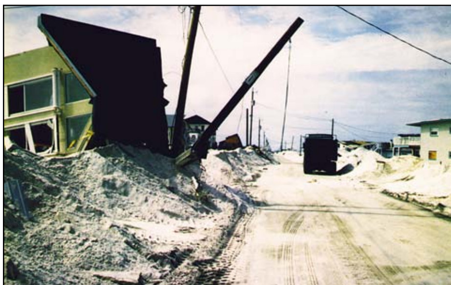
Figure 7-31 Removal of Hurricane Opal overwash from road at Pensacola Beach, Florida. Sand washed landward from the beach buried the road, adjacent lots, and some at-grade buildings to a depth of 3–4 feet.
