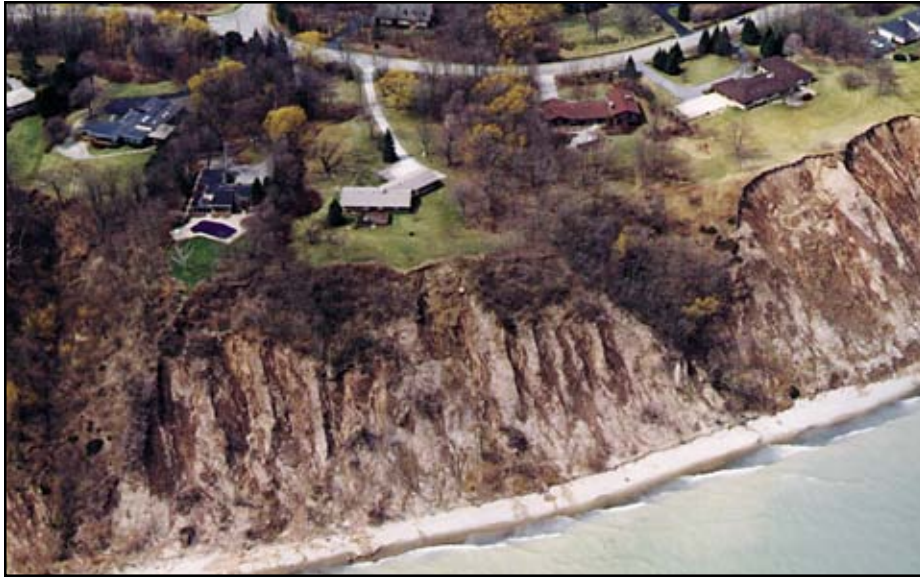
Figure 7-38 Long-term erosion along the Lake Michigan shoreline in Ozaukee County, Wisconsin, increases the threat to residential buildings outside the floodplain. 1996 photograph.
