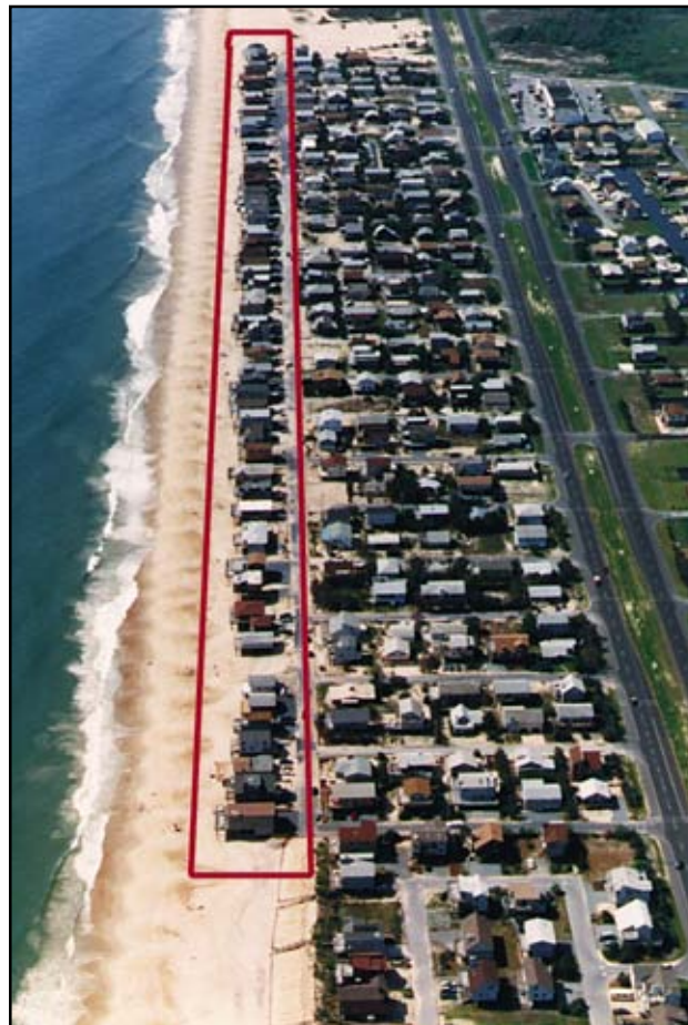
Figure 7-29 Long-term erosion at South Bethany Beach, Delaware, has lowered ground elevations beneath buildings and left them more vulnerable to storm damage. 1992 photograph.
