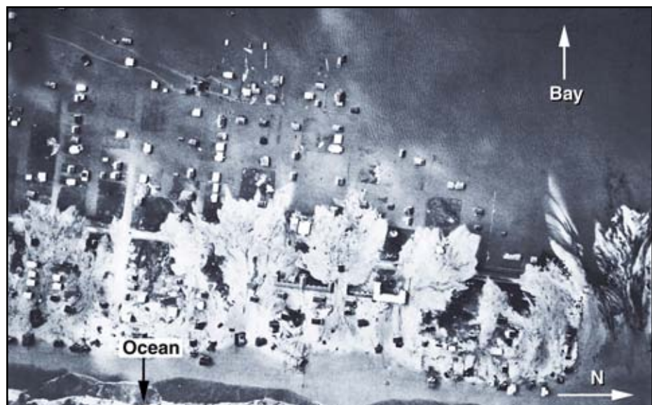
Figure 7-5 March 1962 northeaster. Flooding, erosion, and overwash at Fenwick Island, Delaware.
