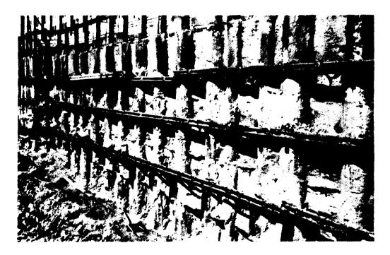
Figure A-2 - Drilled concrete shafts supported by three levels of tie-backs and walers.
