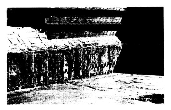
Figure A.4 — Upper wall of soldier piles and wooden lagging braced by two layers of tie-backs with steel walers.
