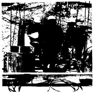
Figure A-10 — Stressing 54 strand tendon, Interstate Highway I-96 retaining wall, Detroit
