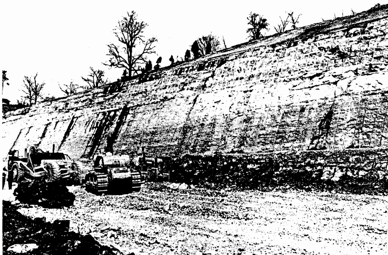
Figure 88.—Stable slope produced by controlled blasting. (Courtesy Austin Powder Co.)
