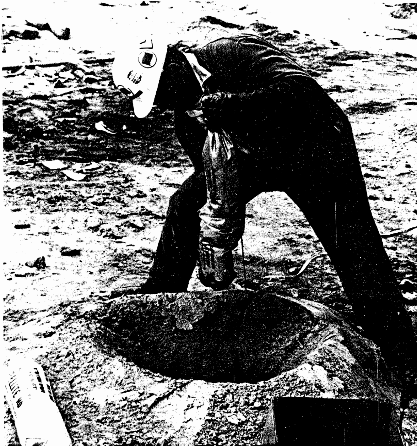
Figure 10.—Loading slurry-filled polyethylene bags. (Courtesy Atlas Powder Co.)
