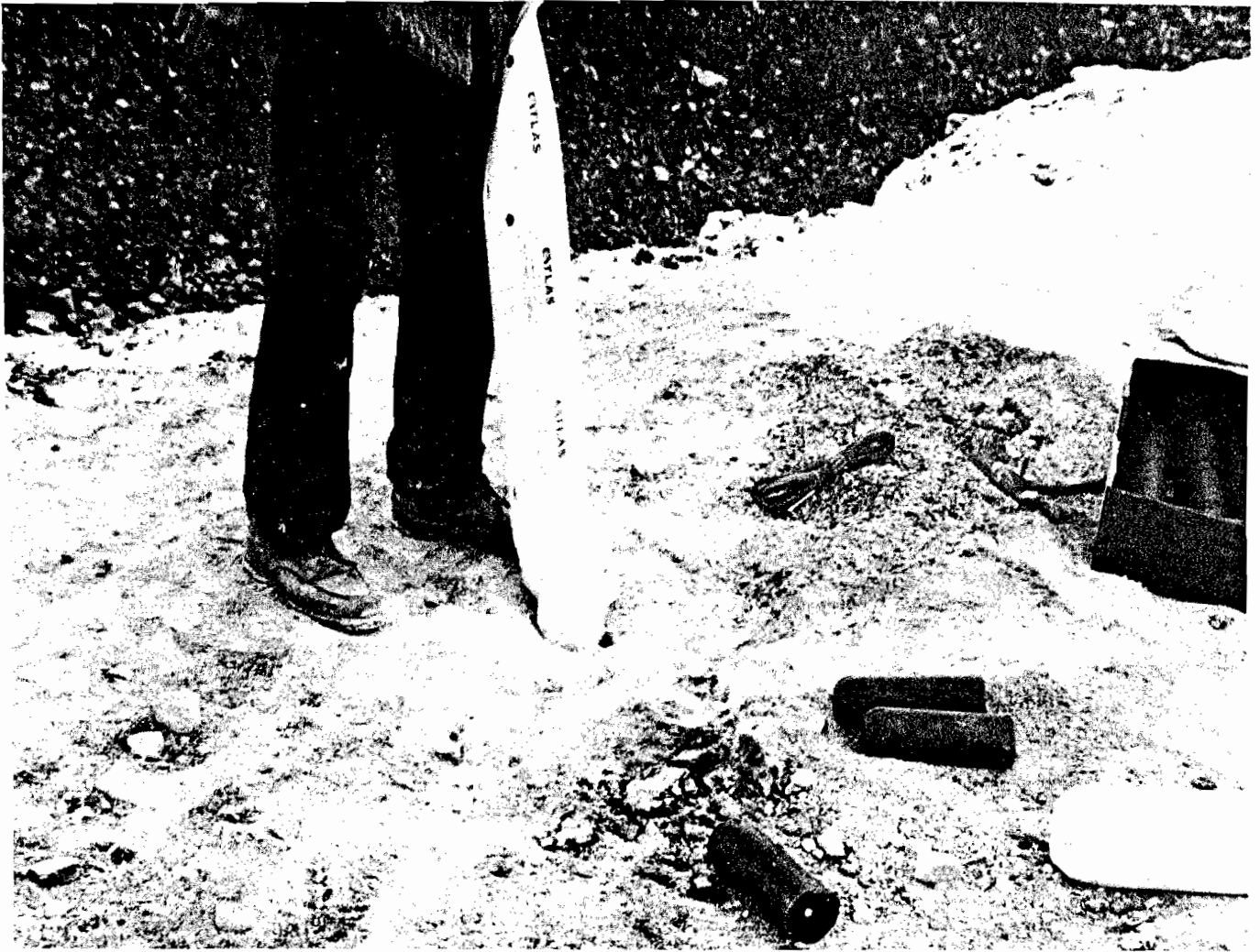
Figure 56.—Pouring slurry into small-diameter borehole. (Courtesy Atlas Powder Co.)
