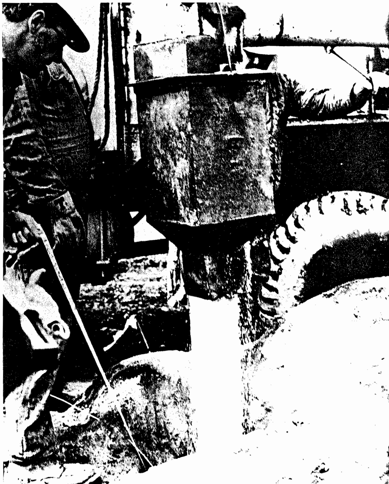
Figure 101.—Checking the rise of the AN-FO column with a weighted tape.
