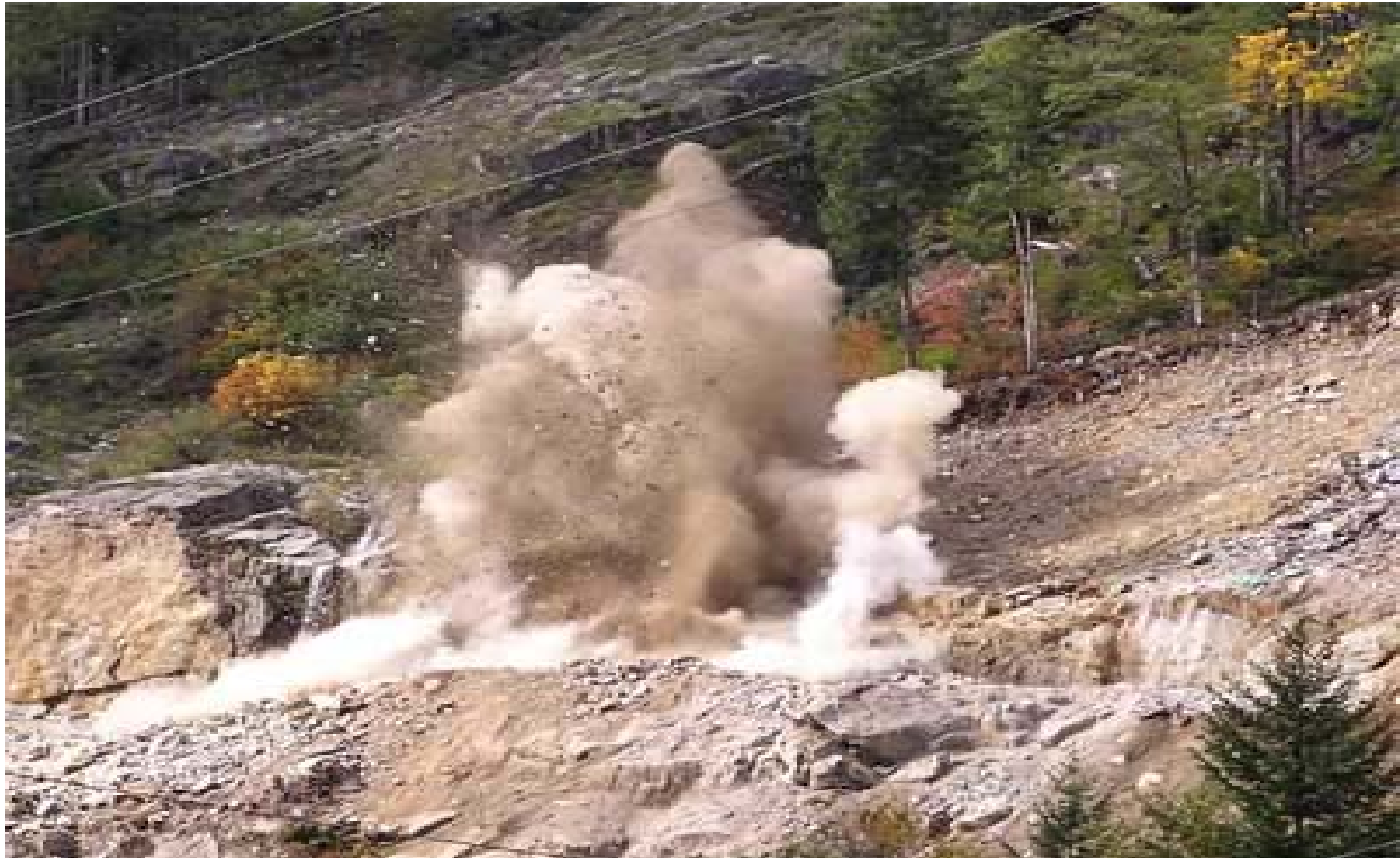
Blasting of a rock slope for a road cut
