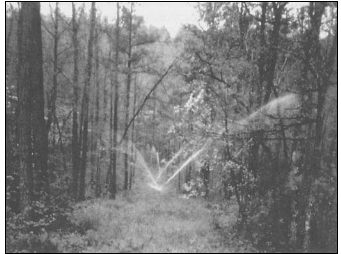
Figure 7-7. Forest Solid Set Sprinkler Irrigation at Clayton County.
