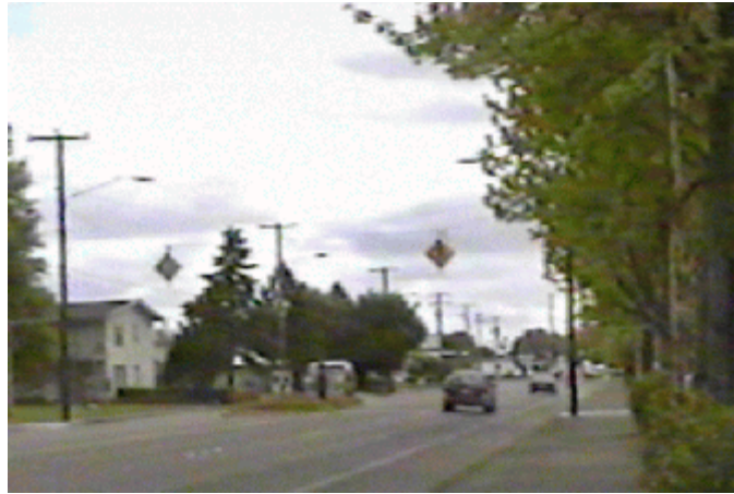
Figure 9. Refuge island, Circle Boulevard, Corvallis, Oregon.
