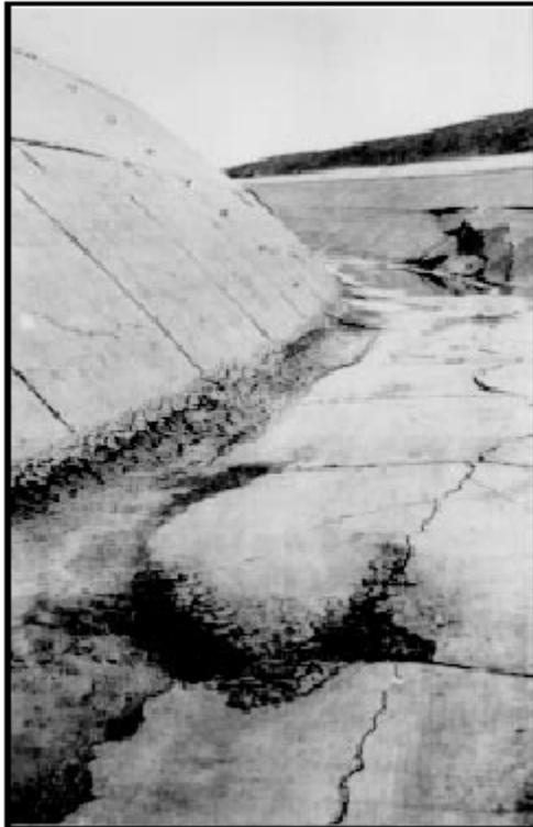
Figure-30.—Heaving of canal bottom (about 300 mm at center), Mohawk Canal, Arizona.
