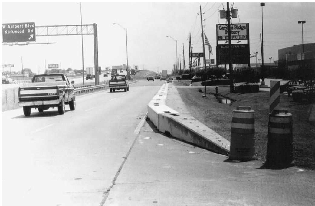
FIGURE 2 LPB, construction zone.
