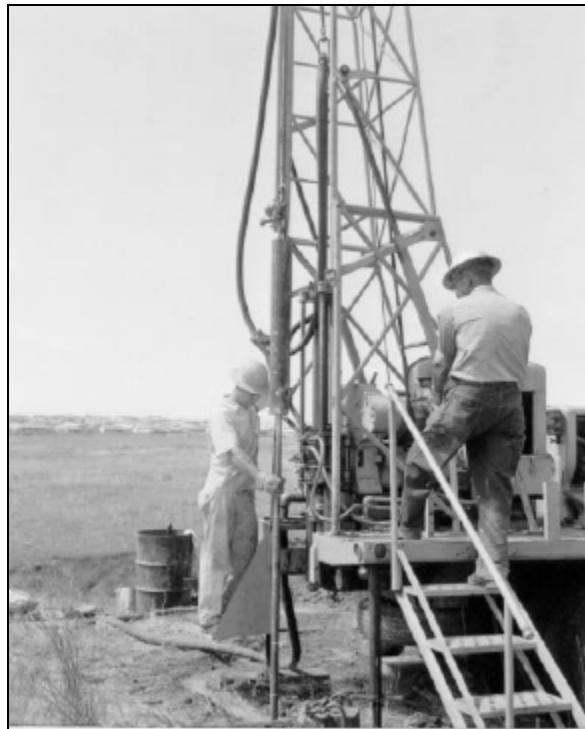
Figure 51. Standard drilling equipment used to perform penetration tests.
