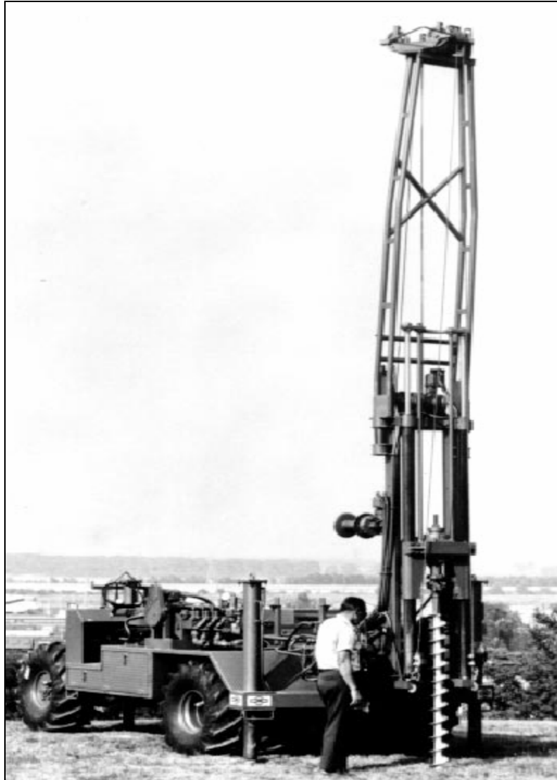
Figure 22. Continuous-flight auger mounted on an all-terrain carrier.
