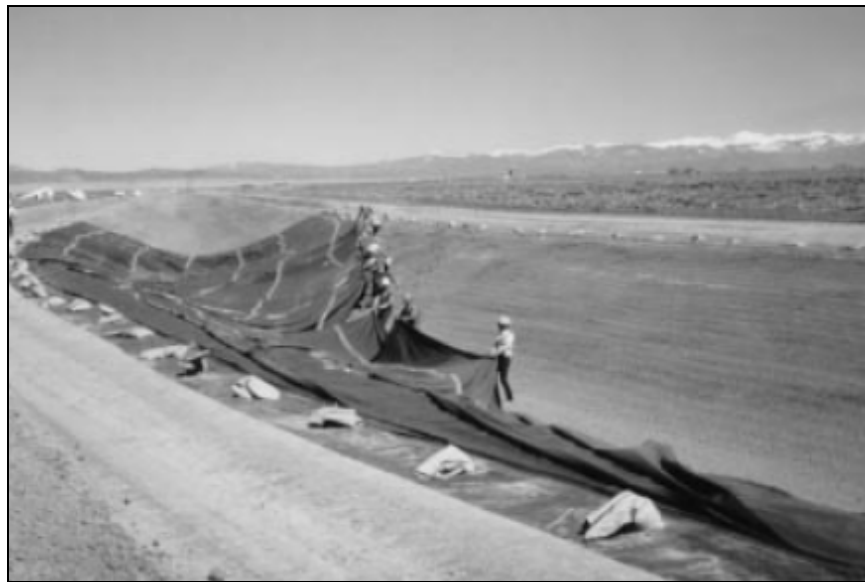
Figure 35, Geomembrane being placed over prepared subgrade.
