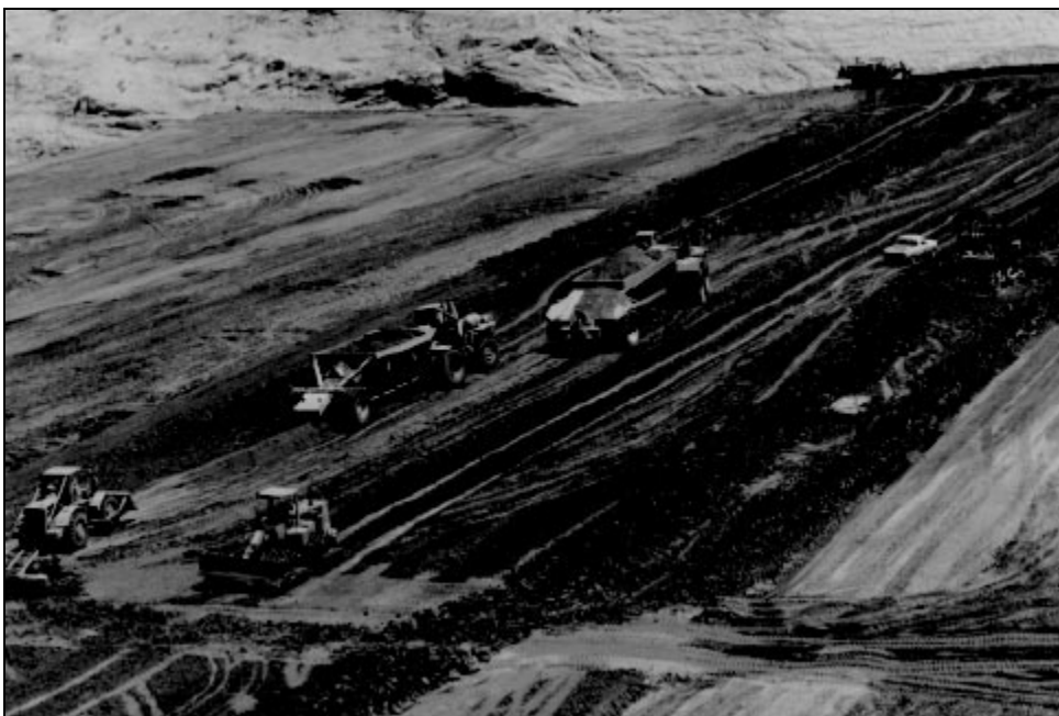
Figure 20, Earth fill operation on an impervious zone
