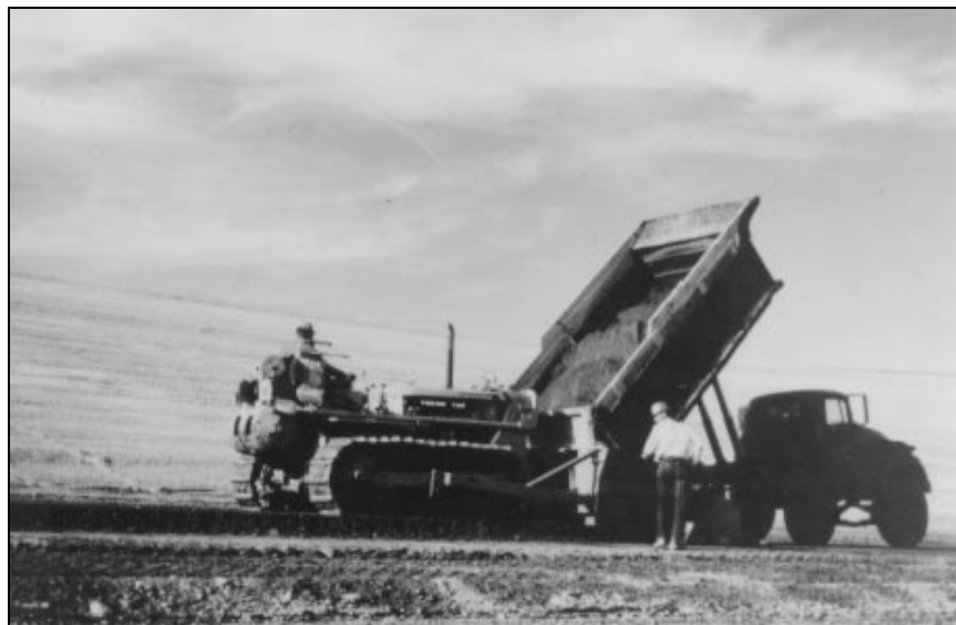
Figure 43, Soil-cement placement with Tractor and Spreader Box.
