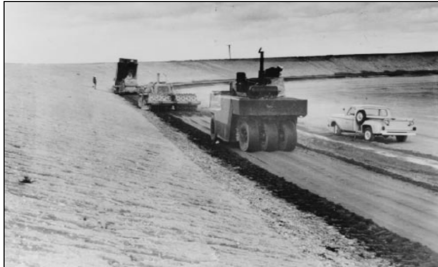
Figure 44, Compaction of soil-cement.
