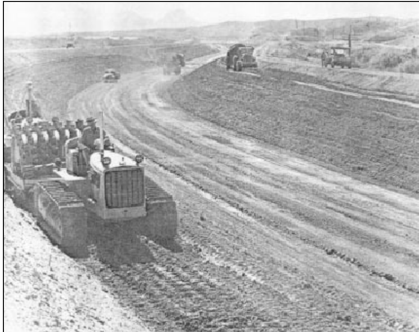
Figure 33, Placing and compacting a thick earth lining.
