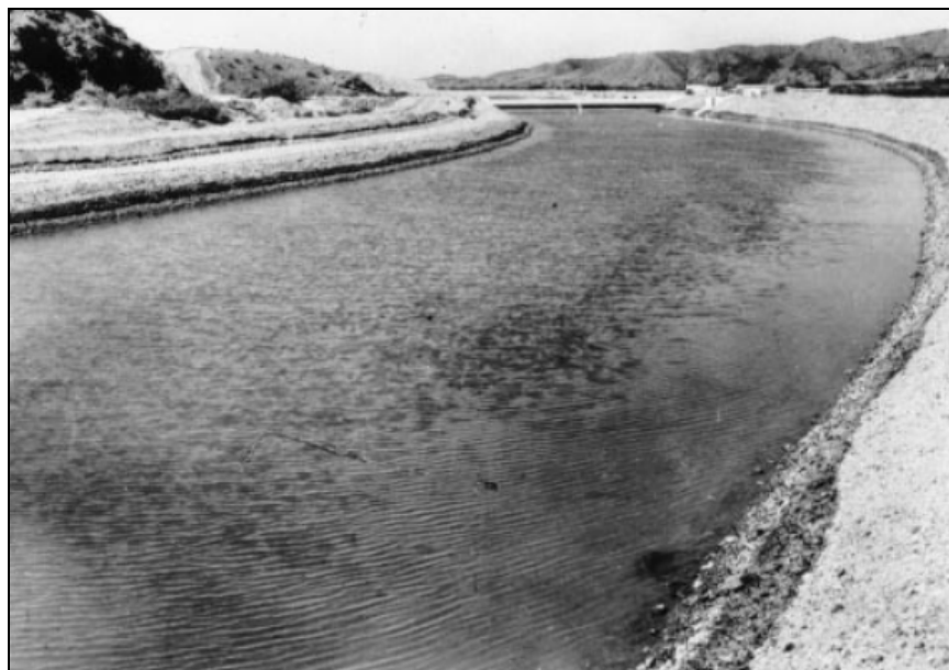
Figure 34, A Completed thick earth lining.
