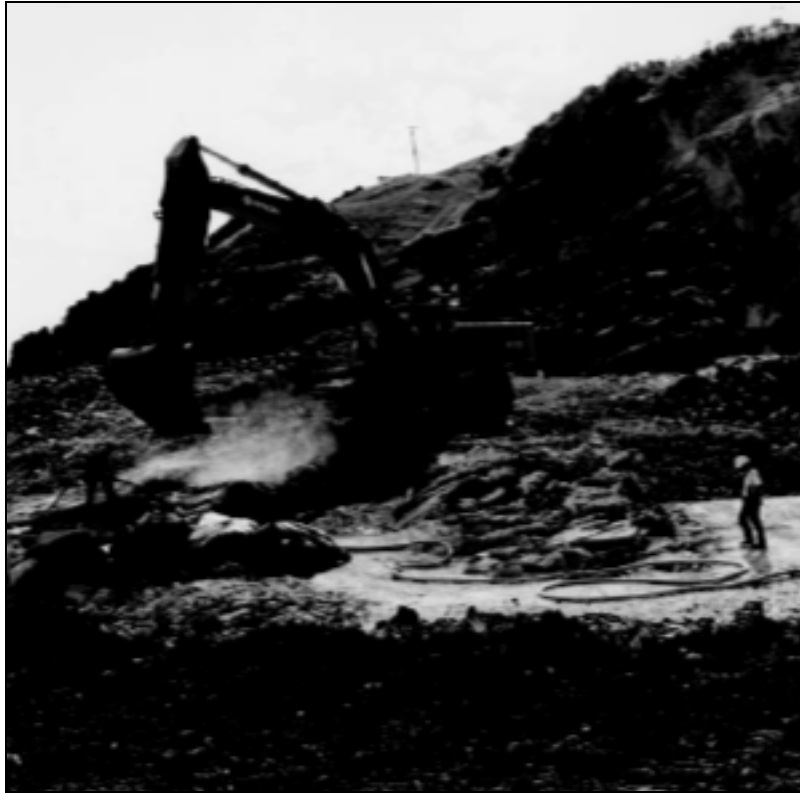
Figure 17, Foundation preparation for the impervious (zone 1) foundation.
