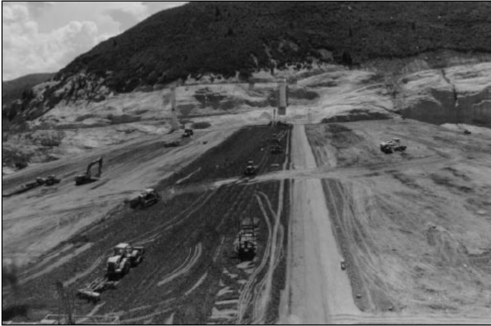
Figure 21, View of a Dam under construction.
