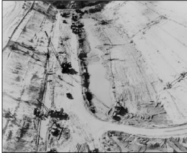
Figure 5, Cutoff trench at a dam in Arizona.
