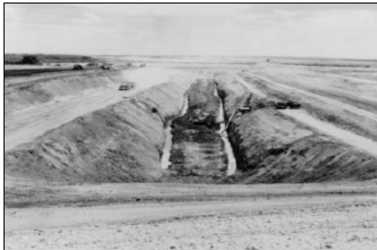
Figure 6, Cutoff trench at a dam in Texas.
