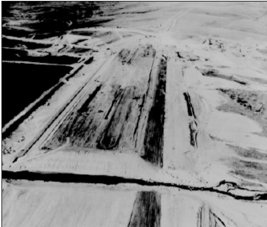
Figure 16, Temporary diversion channel through A Dam.
