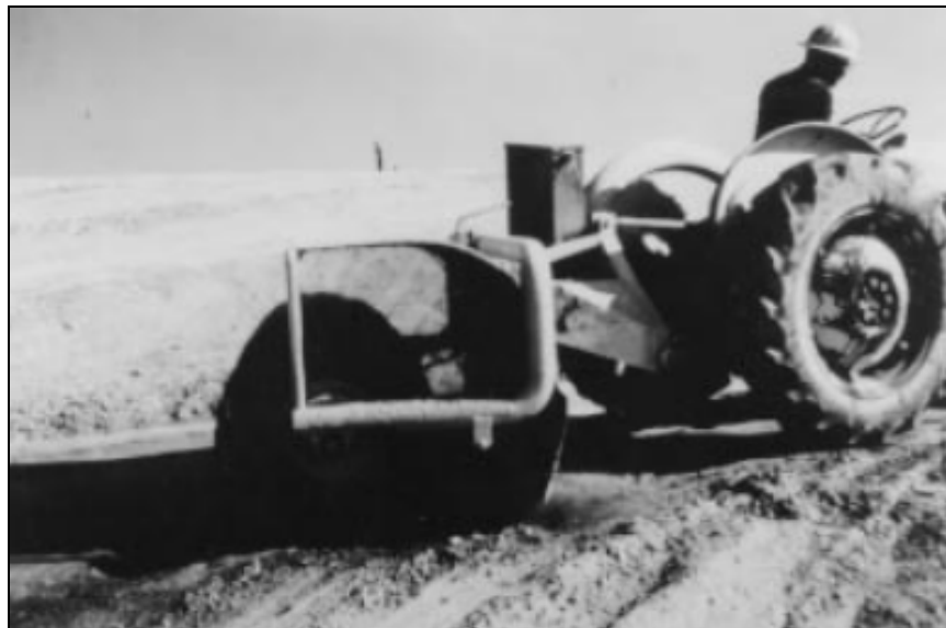
Figure 45, Power brooming of surface prior to placement of the next lift.
