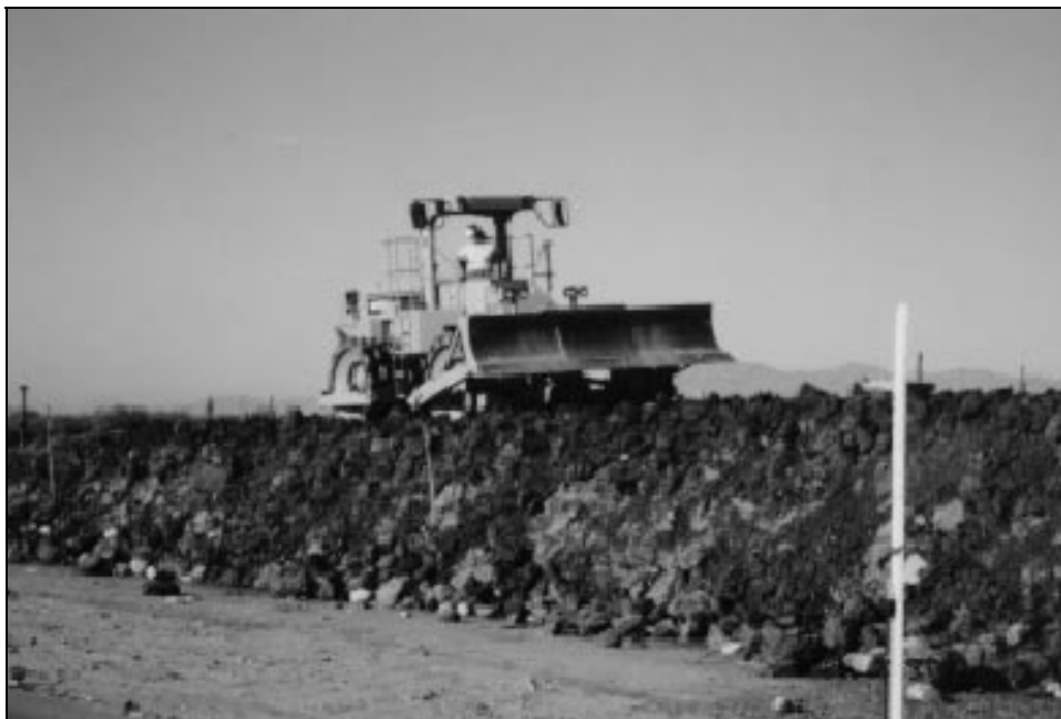
Figure 22, Pad foot roller on a test fill of zone 1 material
