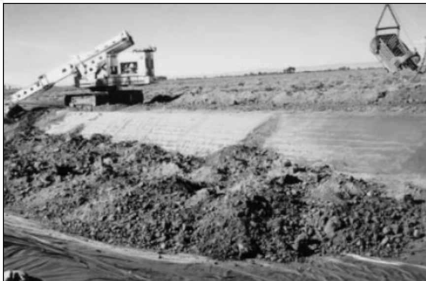
Figure 36, Placement of a protective earth cover over a geomembrane.
