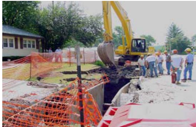
Figure 5-6 Open Cut Installation of Sewer Pipe
