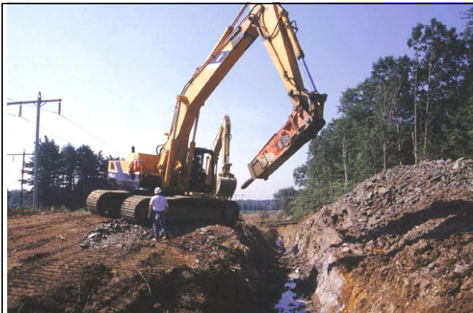
Figure 17: Backhoe with Hydraulically Operated Jackhammer for Rock Breaking
