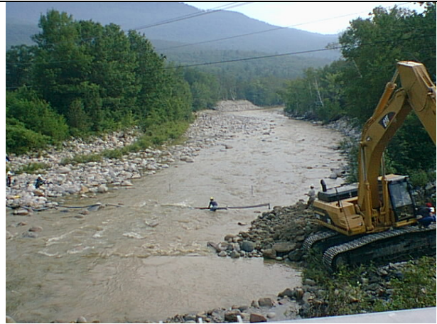
Figure 33: Open-Cut Waterbody Crossing - Backhoe Transferring Material in Relay
