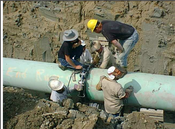
Figure 23: Lining Up Two Pipe Joints for "Tie-In Weld" Using Clamps
