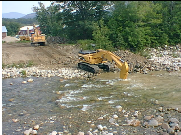
Figure 32: Open-Cut Waterbody Crossing - Backhoe Excavating River Bed
