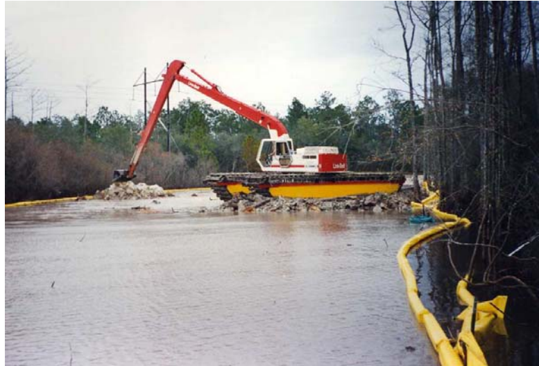
Figure 16: Floatable "Swamp-Hoe" Ditching within Wetland
