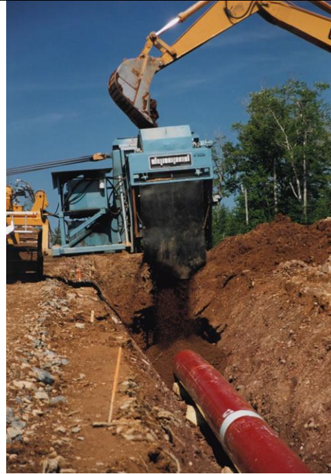
Figure 30: “Dyndopad” Type Padding Machine is Manually Fed by Backhoe
