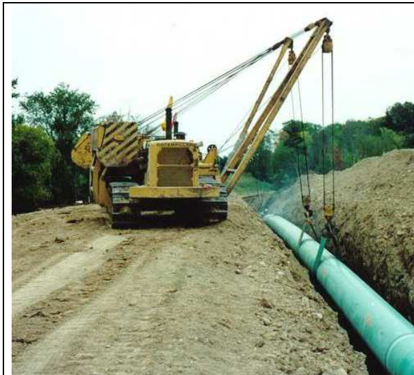
Figure 27: Sidebooms Lowering-In Pipeline
