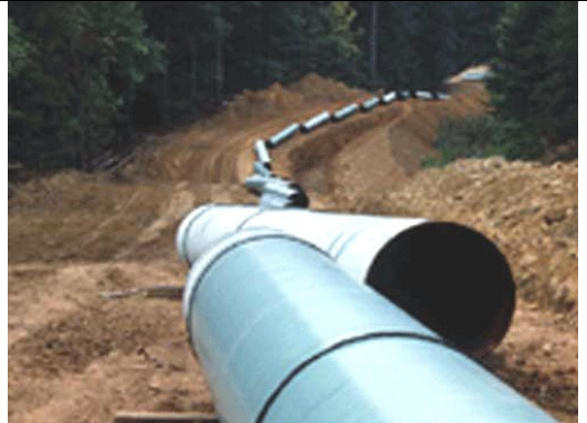
Figure 20: Pipe Strung Along the Ditchline
