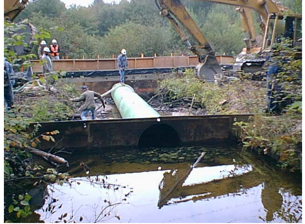
Figure 35: Custom Flumed Dry-Cut Waterbody Crossing with Excavation Ready to Begin
