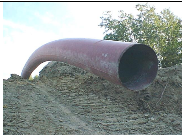
Figure 22: "Over-bend" Pipe
