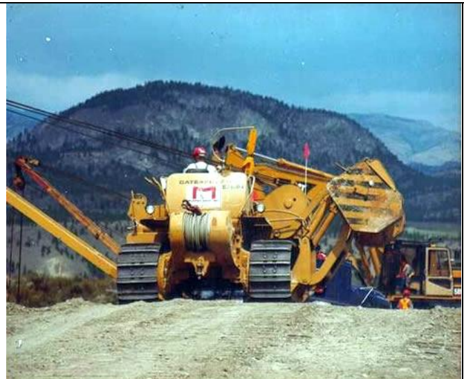
Figure 28: Sidebooms with Counter-Weights Fully Extended Holding a Heavy Load
