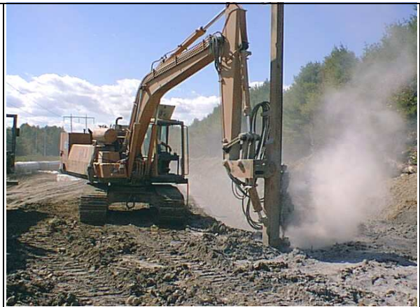
Figure 18: "John Henry" Drilling Holes for the Insertion of Blast Explosives
