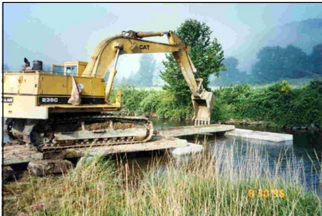
Figure 11: Waterbody Bridge Installation
