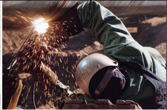
Figure 24: Mainline Welder at Work
