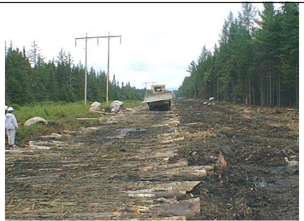
Figure 12: Equipment Support “Rip-Rap” Log Corduroy Road Through Wetland
