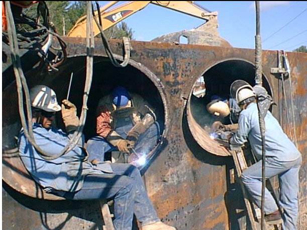
Figure 36: Fabrication of Dual Flume Assembly
