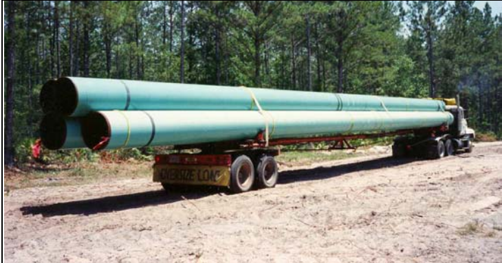
Figure 19: Stringing Truck Delivering Pipe
