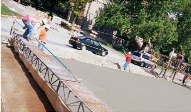
Figure 3-5. Fly ash concrete finishing
