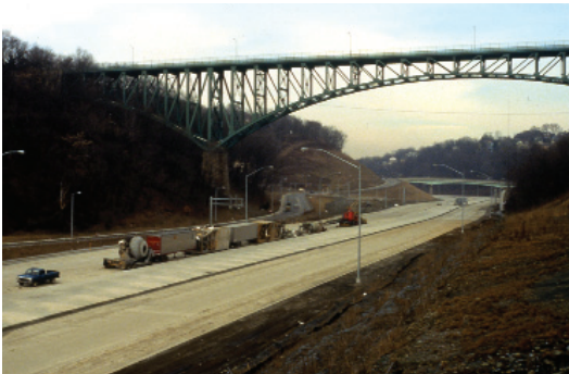
Figure 6-1. Highway embankment with fly ash structural fill.
