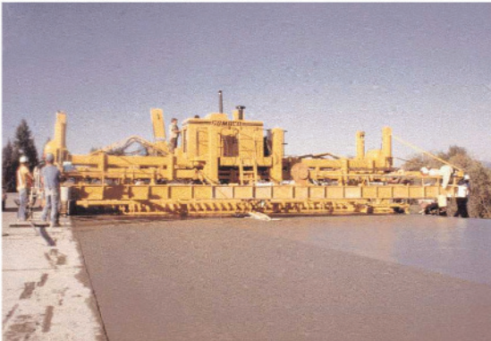
Figure 3-1. Fly ash improves workability for pavement concrete.
