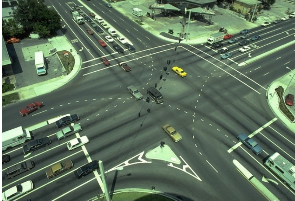
Figure 11. Pavement markings can be used to delineate travel lanes within wide intersections as shown in the photograph.
