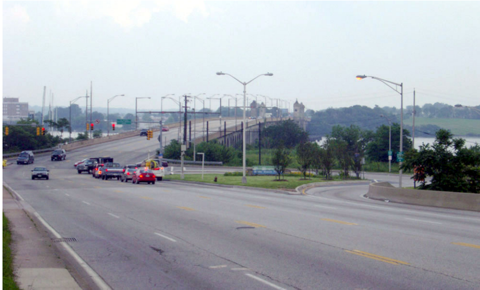
Figure 78. Example of a jughandle intersection.
