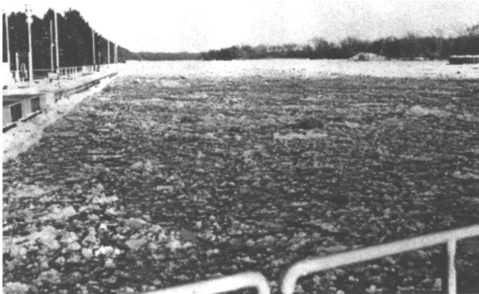
Figure 14-2. Ice accumulation in the upper lock approach area
