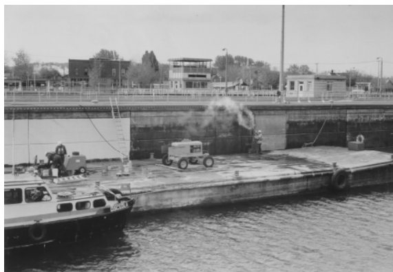
Figure 18-20. Application of copolymer coating.
