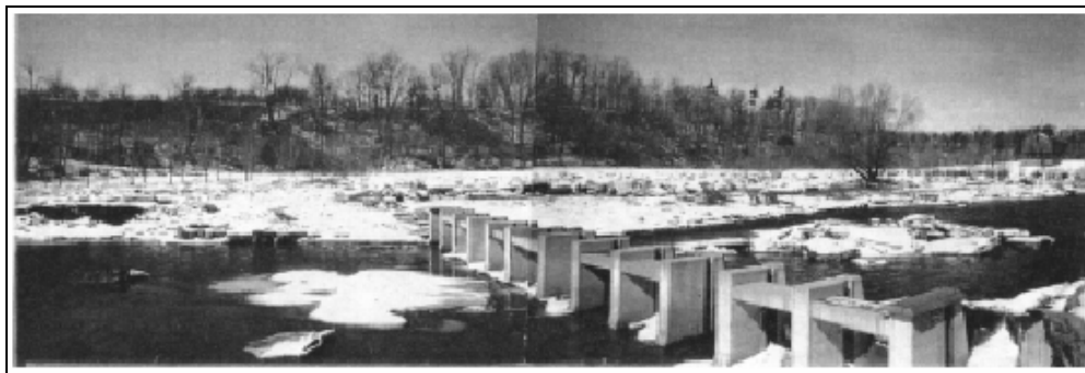
Figure 3-33. Credit River ice control structure following breakup, March 1994. Note the ice stored on the right flood plain. (Photos courtesy of Harold Belore.)
