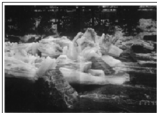
Figure 3-34. Cut granite block ice control structure in Hardwick, Vermont, following breakup, March 1995.
