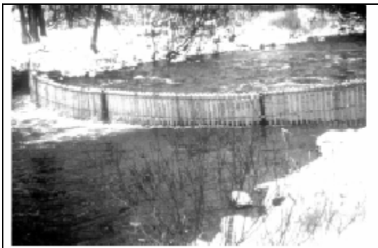
a. Installed condition.
