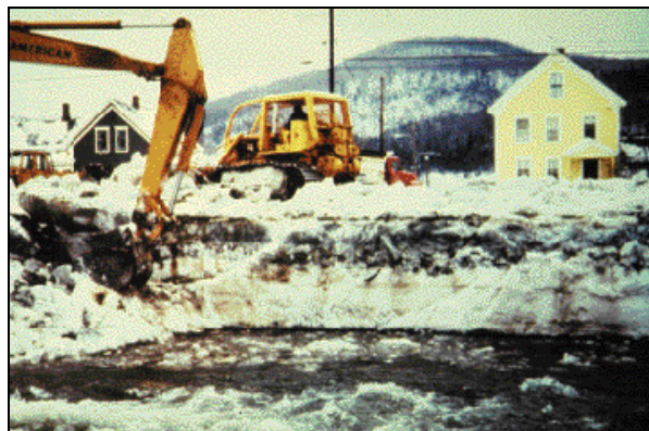
Figure 3-18. Breaching an ice jam in Hardwick, Vermont, using excavation equipment working from the shore and a bridge (bridge is not shown, but is just beyond the left edge of the photograph).
