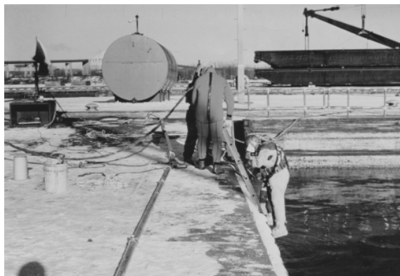
Figure 18-13. Diver working to install air screen system.
