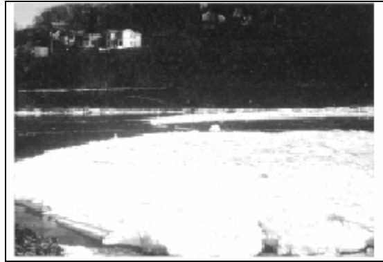
Figure 3-25. Allegheny River ice boom.
