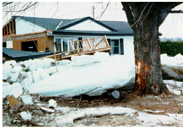
Figure 10-4. Damage from January 1996 breakup jam, Saranac River near Plattsburgh, New York.
