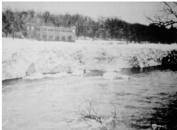
Figure 10-7. Jam immediately downstream of power plant, Fox River, near Ottawa, Illinois.
