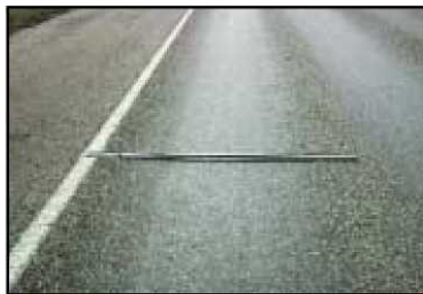
FIGURE 32 Distress Type ACP 9—Rutting
