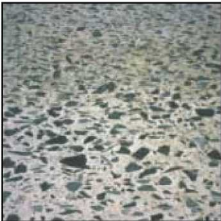
FIGURE 72 Distress Type JCP 9—Polished Aggregate
