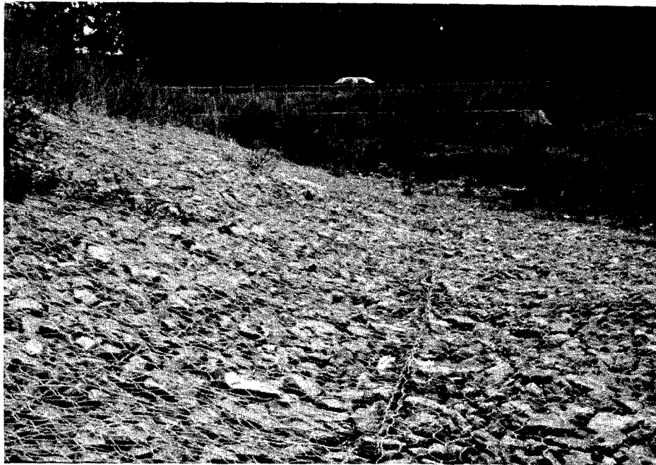
Figure 9. Rock and wire mattress revetment.
