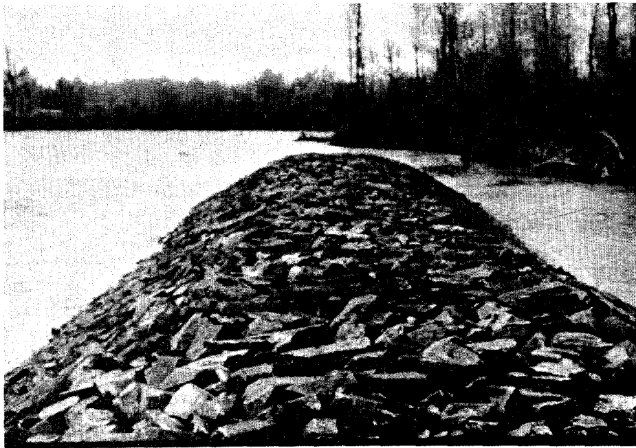
Figure 7. Plated or keyed riprap.
