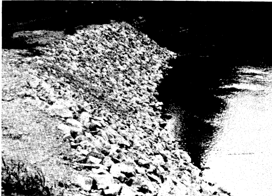
Figure 6. Hand-placed riprap.
