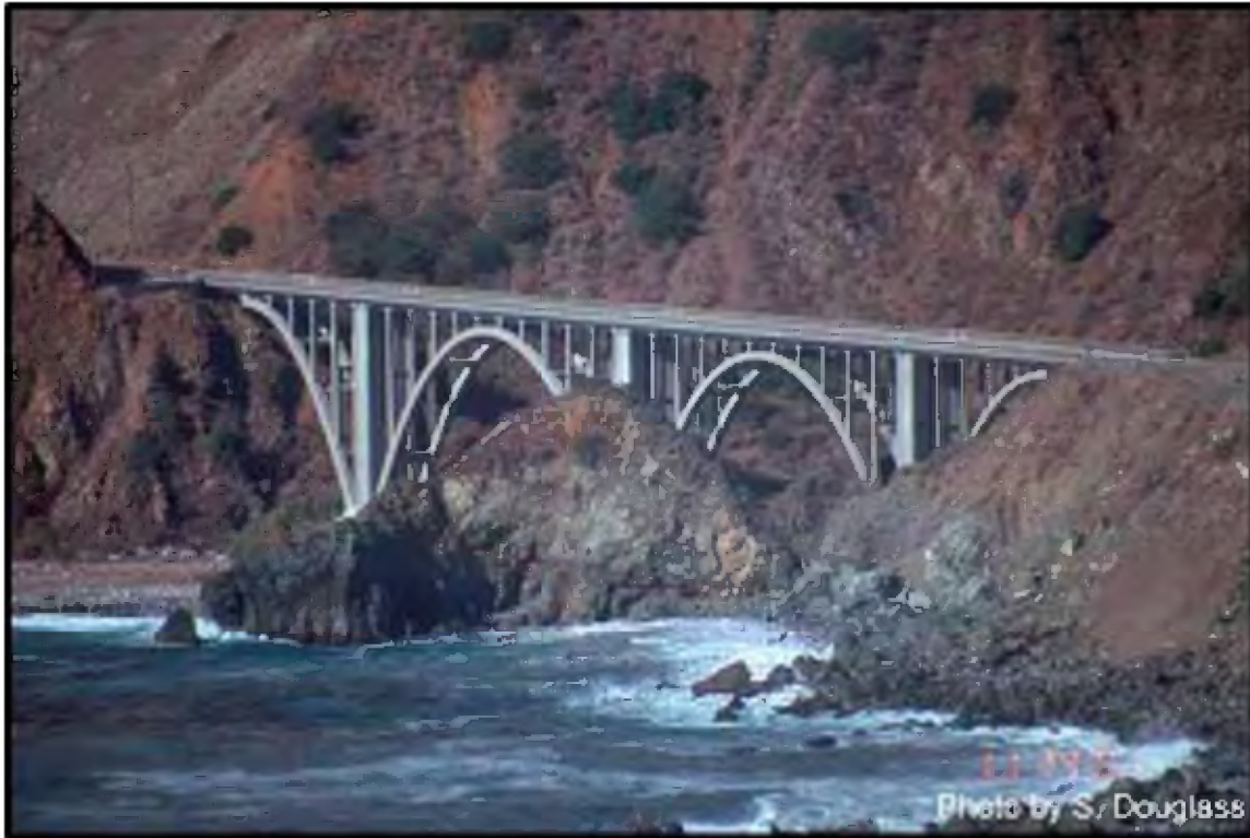
Figure 2.2. Bridge on the Pacific Coast Highway (California Route 1).
