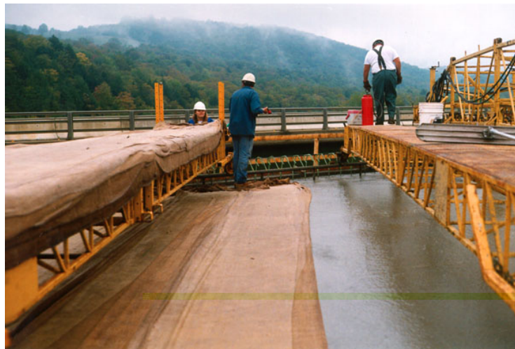
Figure 8.6.3-1 Note the proximity of the burlap to the finishing machine
