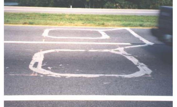
They consist of a loop of wire buried in the pavement that, when connected to an inductive loop detector unit, senses the presence of a vehicle by detecting changes in inductance caused by the vehicle's presence. They are capable of providing both presence detection and motion detection.
