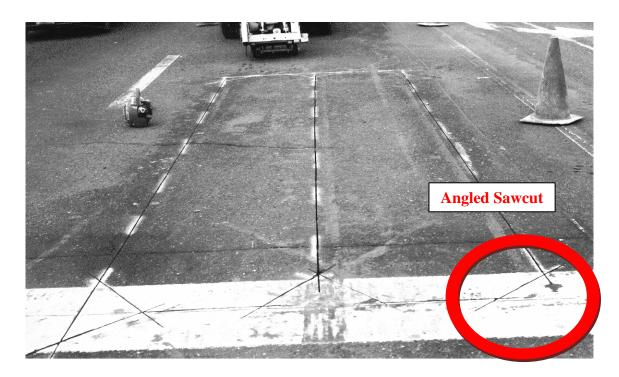
The use of preformed loops has gained popularity in recent years. These loops are typically used where new pavement construction is occurring. The loops are fabricated at a central location, transported to the site, and then installed between pavement layers. With a bit more difficulty, preformed loops can be sawcut into existing pavement. The primary advantage of preformed loops is the consistent quality of their construction.
