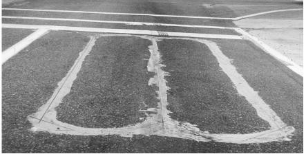
• Use power heads, which provide additional turns of wire at the front end of the loop, thus increasing loop sensitivity in this area.
