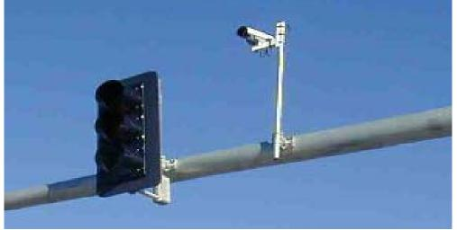
These systems are quite sophisticated, using machine vision and complex computer algorithms to evaluate changes in the video image which indicate the presence of a vehicle. Accurate detection requires that the system be able to operate successfully in all kinds of weather and under a variety of ambient light conditions.
