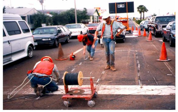
Inductance loops are typically constructed using number 14 or number 12 AWG (American Wire Gauge) XHHW cross-linked polyethylene wire rated for 600 volts. The depth of the sawcut depends on the number of turns of loop and wire size. As a general rule, a sawcut depth that provides 1 inch of cover is used for concrete pavements and a sawcut depth that provides 2 inches of cover is used for asphalt pavements.
