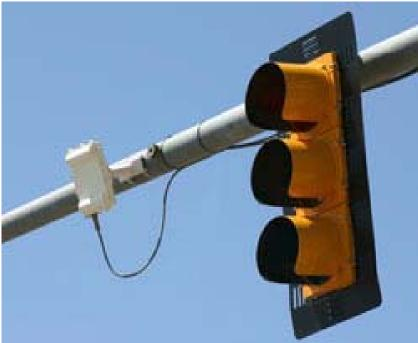
As is the case with underground detection, there are a number of different nonvideo technologies that can be used in overhead applications to provide vehicle detection inputs for actuated signal control:
