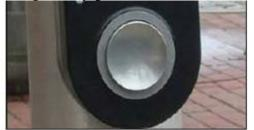
When a pedestrian pushes the button, a call for pedestrian service is registered with the controller for the corresponding pedestrian phase. The pedestrian call is then is serviced (the WALK indication is displayed) at the appropriate time in the signal cycle.
