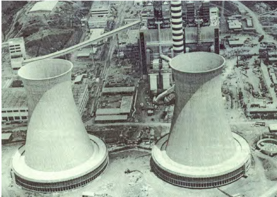
Figure 4-5. Hyperbolic Natural-Draft Cooling Towers
