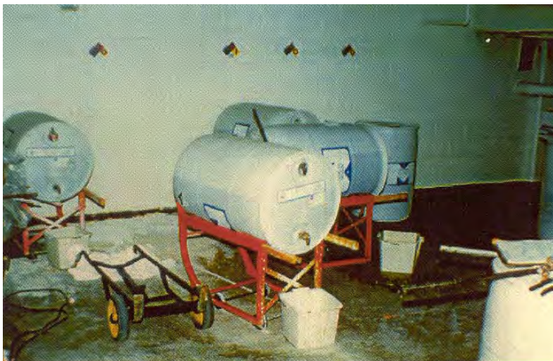
Figure 7-2. Manual Chemical Feed System
