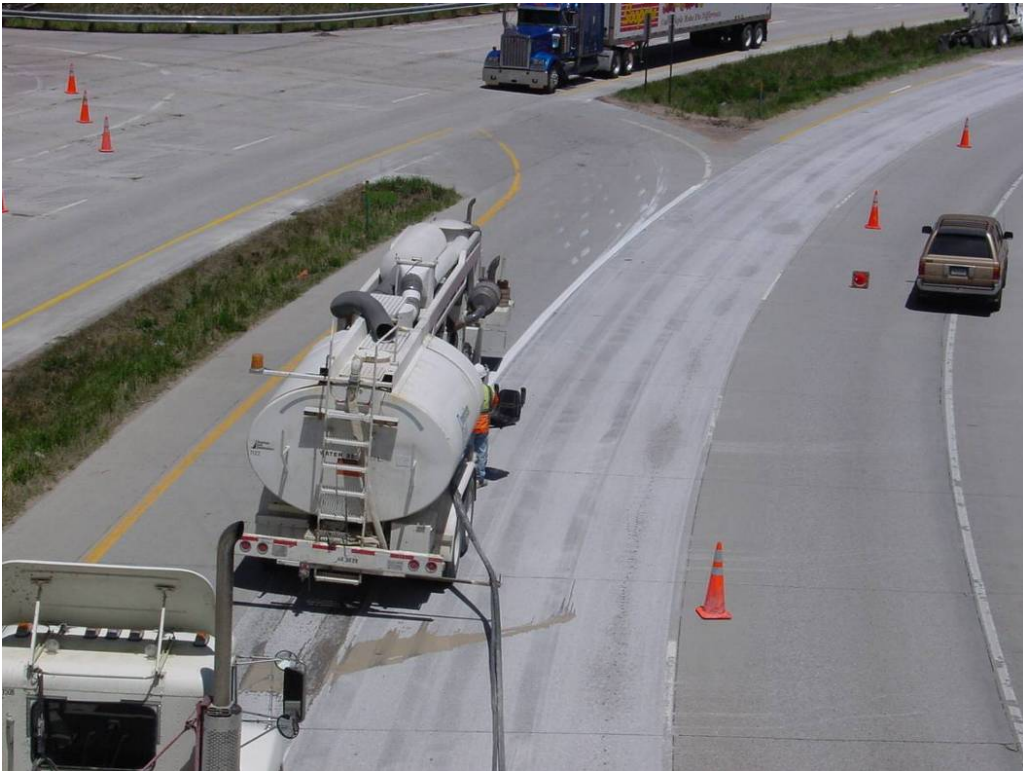
Figure 5-9 Grinding process (Courtesy of Caltrans)
