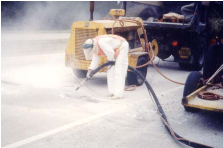
Figure 7-4 Cleaning the repair area with sandblasting equipment (FHWA, 2006)
