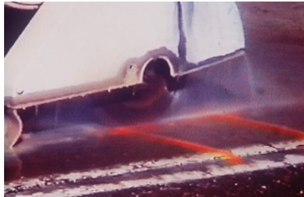
Figure 7-2 Concrete removal using the saw and patch methodology (FHWA, 2006)
