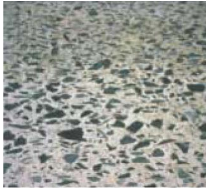
Figure 1-14 Example of surface polish/polished aggregate (FHWA, 2003)
