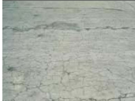
Figure 1-12 Map-cracking (FHWA, 2003)
