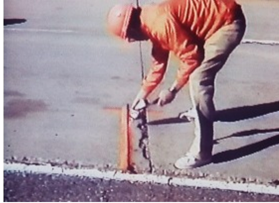
Figure 7-1 Marking damage area for removal (FHWA, 2006)
