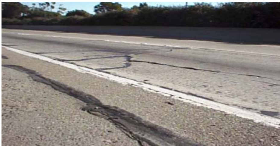
Figure 1-20 Settlement (Caltrans, 2004b)
