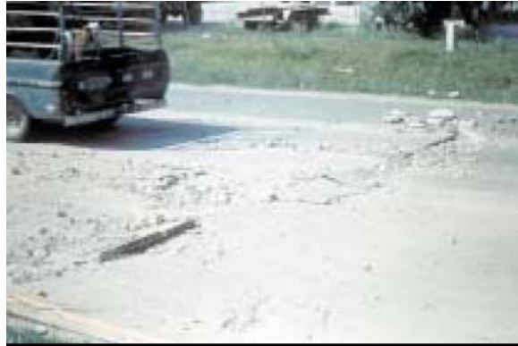
Figure 1-17 Example of blow-ups (FHWA, 2003)
