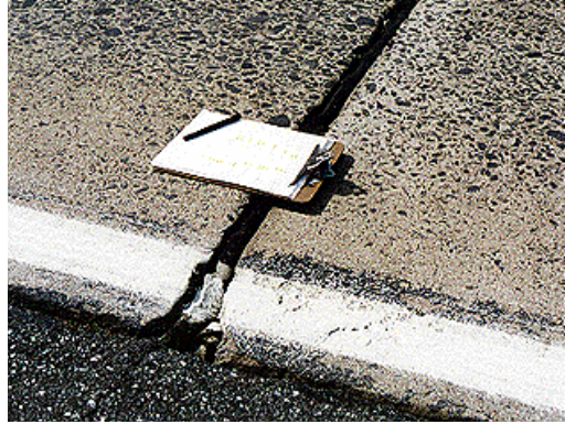
Figure 1-5 Faulting (FHWA, 2003)
