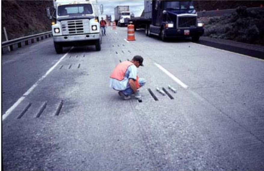
Figure 6-12 Placing dowel-chair assembly (Caltrans, 2006a)
