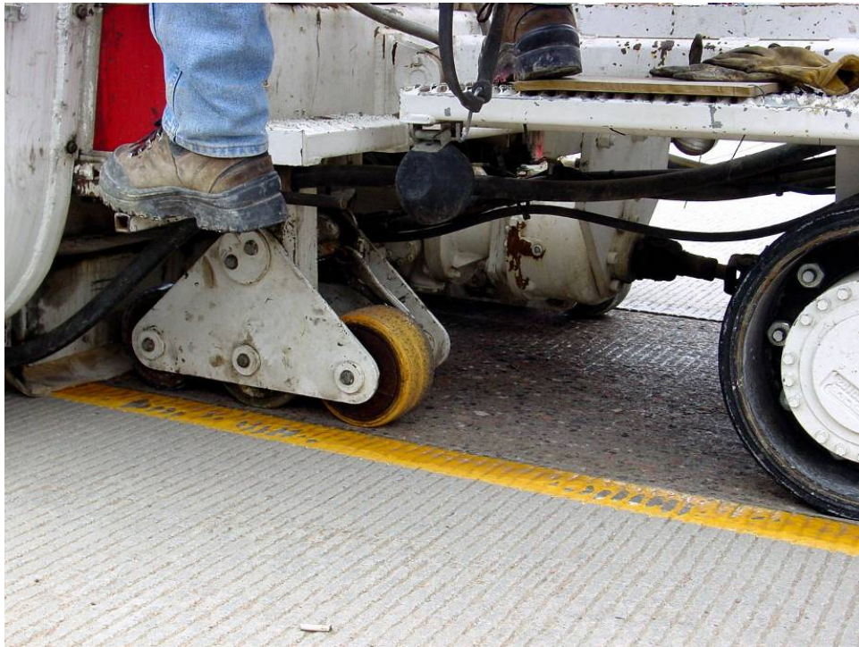
Figure 5-13 Pavement surface texture behind grinding head (Courtesy of Caltrans)
