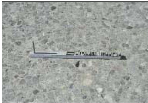
Figure 1-16 Example of popouts (FHWA, 2003)
