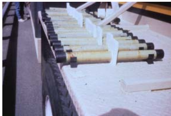
Figure 6-2 Photo of dowels with chair, end caps, and foam core inserts in place (Caltrans, 2006a)
