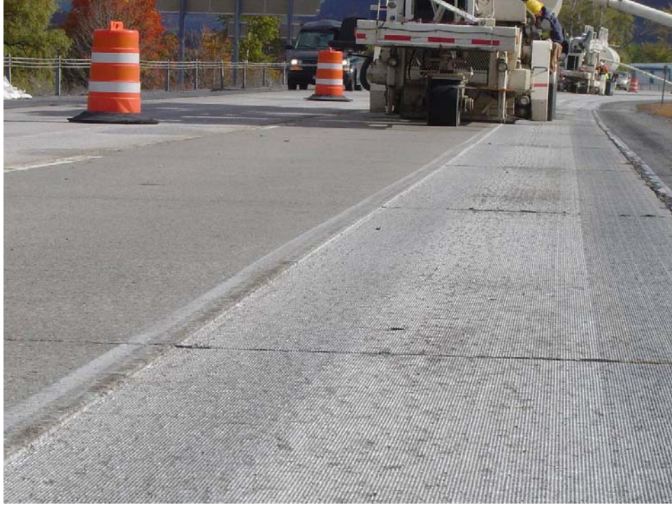
Figure 5-12 Pavement surface after diamond grinding (Courtesy of IGGA)
