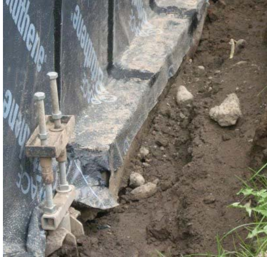
Figure 3: Underpinning Application with Lifting Bracket
