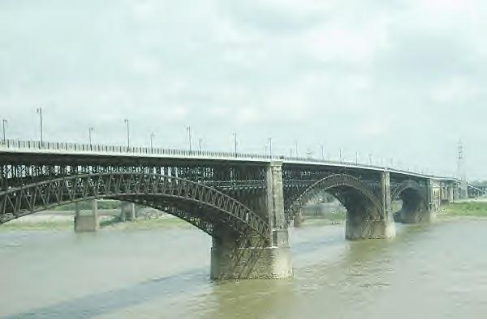
St. Louis Bridge (a.k.a. Eads Bridge )
