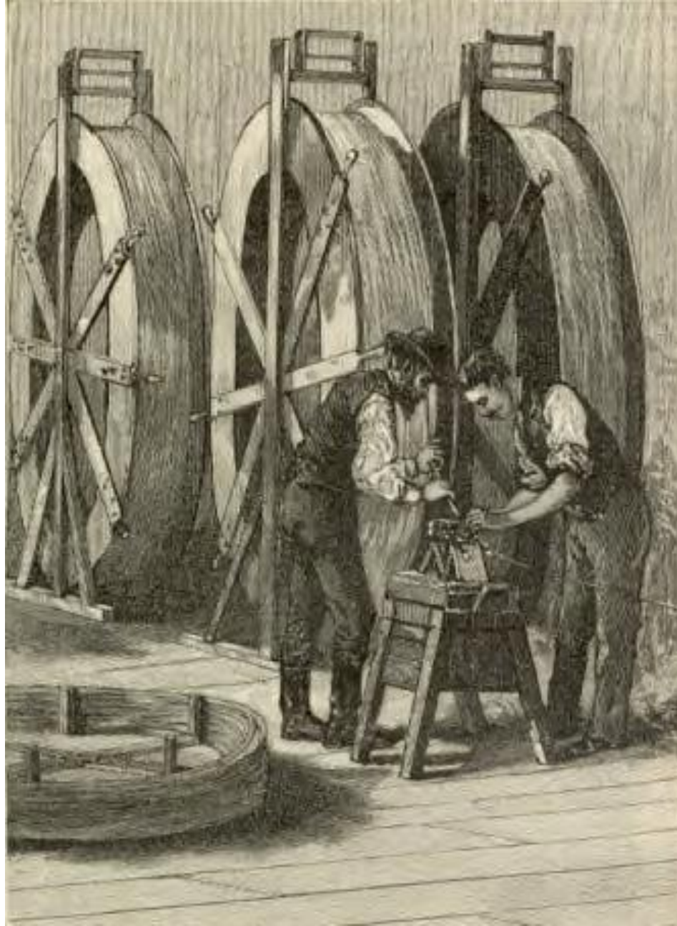
Splicing the wire (in Ferrule) off the wooden coils
