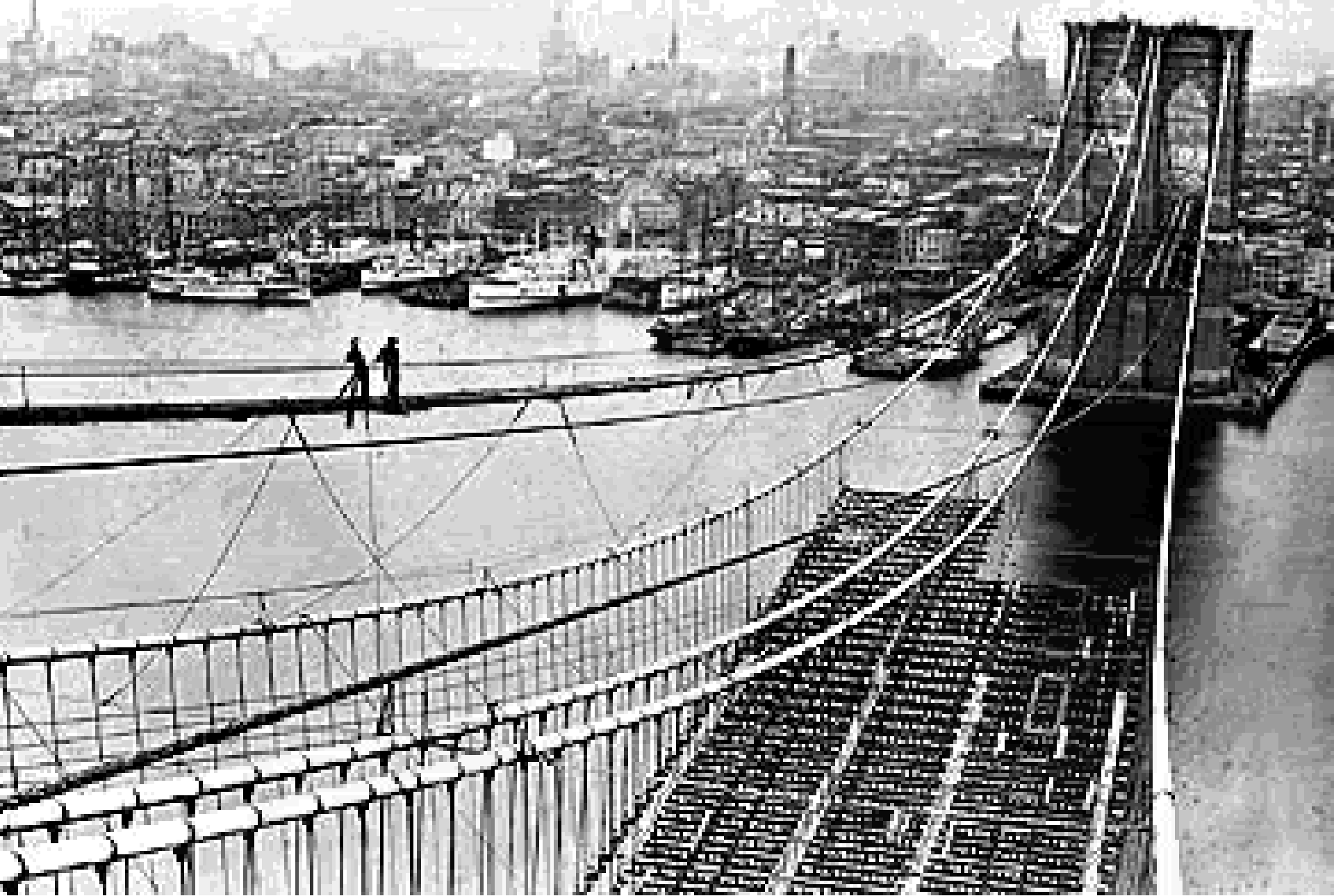
Deck trusses nearing mid-span
