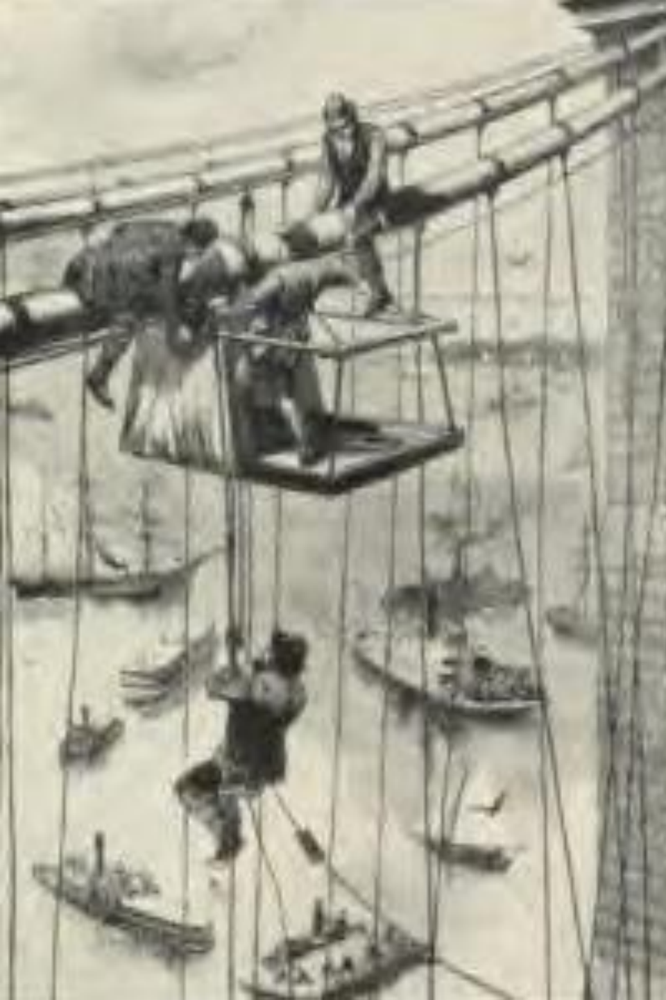
Newspaper drawing depicting workers installing the suspender cables (1880)
