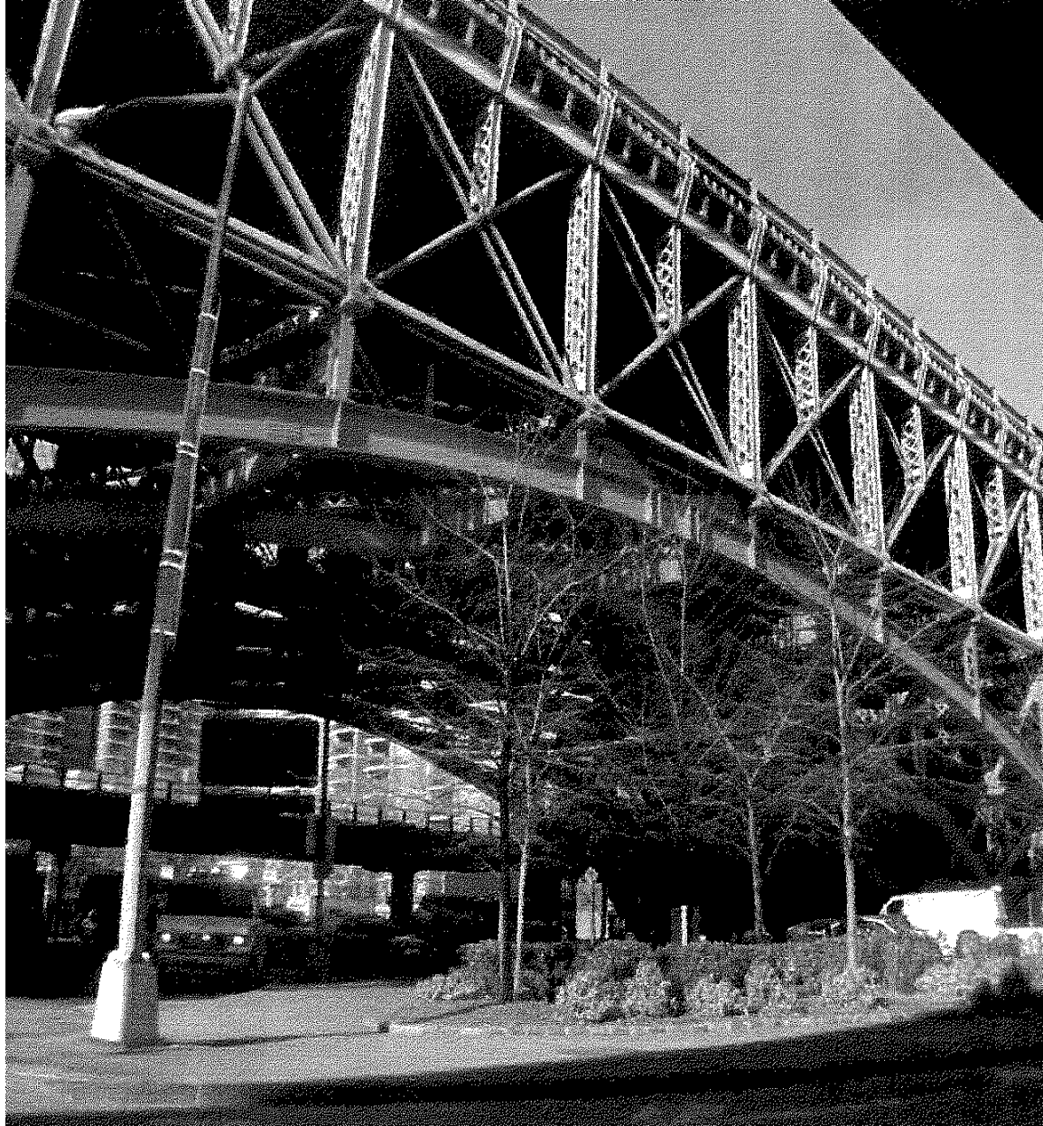
North William Street Bridge (replacement with steel arch - present day)
