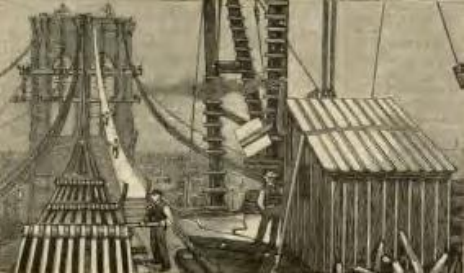
Eye-Bar Chain (connecting to cable strands)
