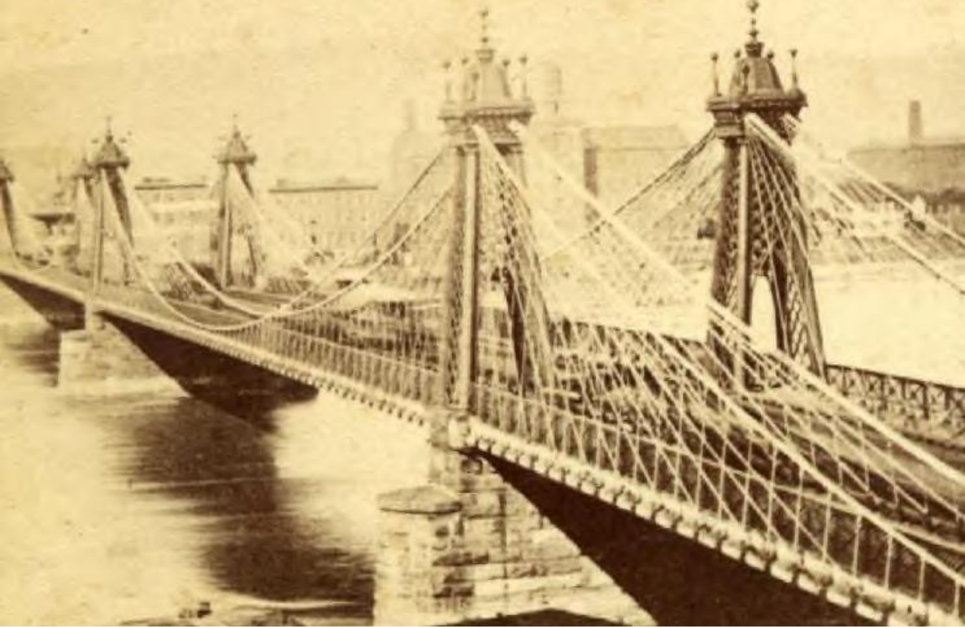
Allegheny River Bridge, 1857 by JAR Pittsburgh, PA
