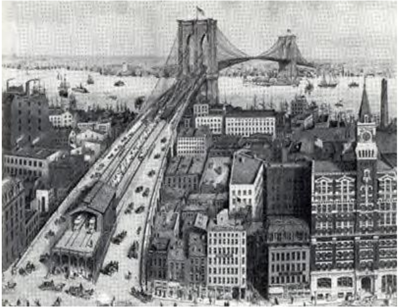
NY Terminal (left) and Tribune Tower (right), ca. 1883 (Pulitzer's World Building was completed in 1890)
