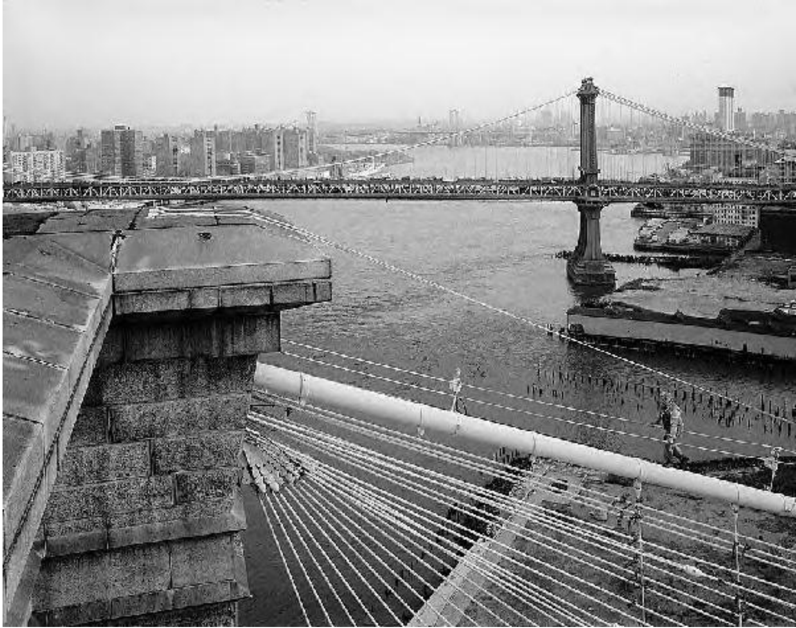
Radiating cable stays off Brooklyn Tower (foreground) Manhattan Bridge (background)
