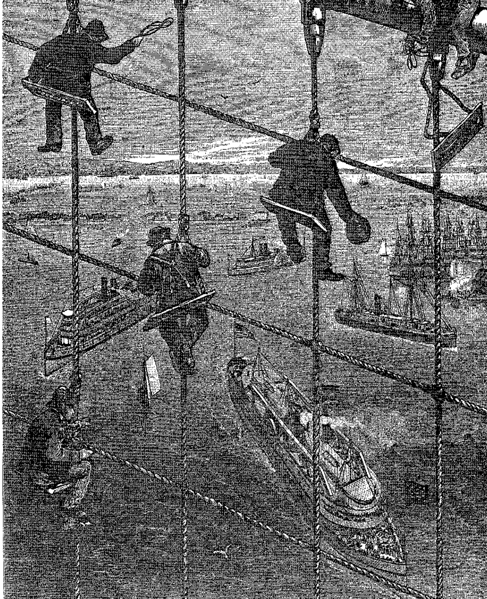
JAR's trademark cable stays (being tied to the suspender cables)
