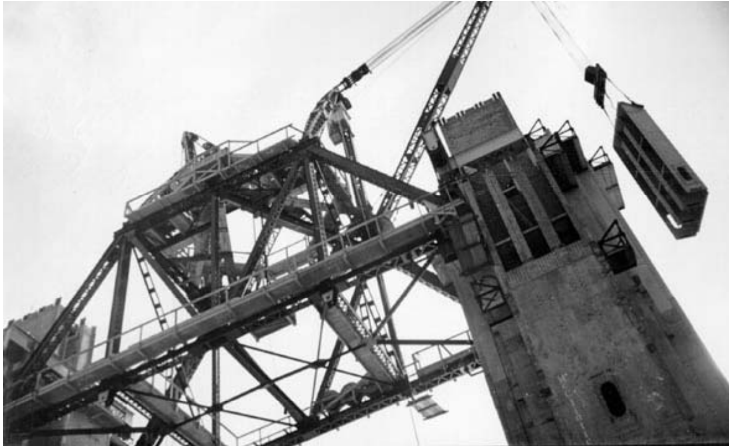
Creeper Crane (lifting steel sections into position)
