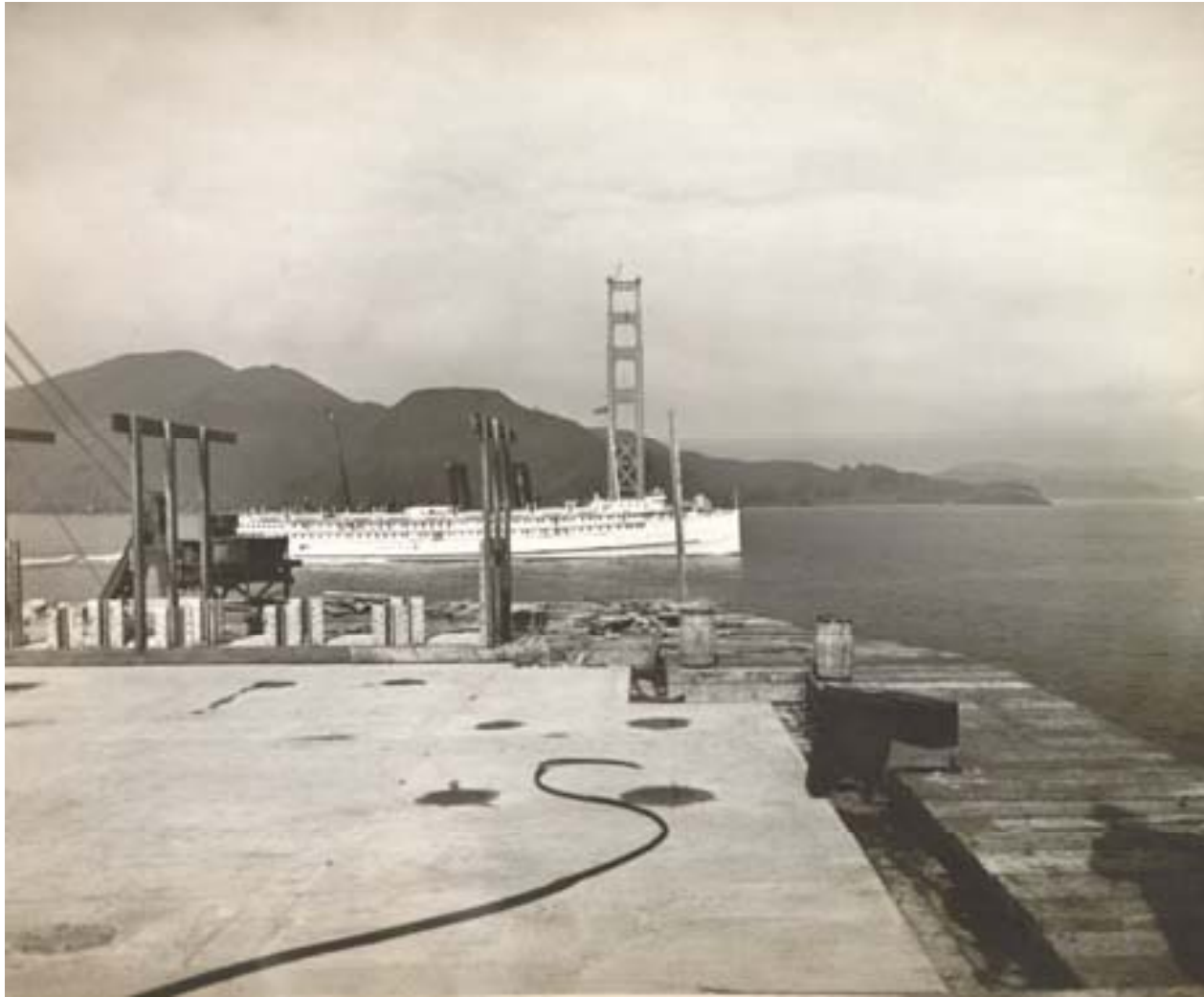
Atop the completed pier
