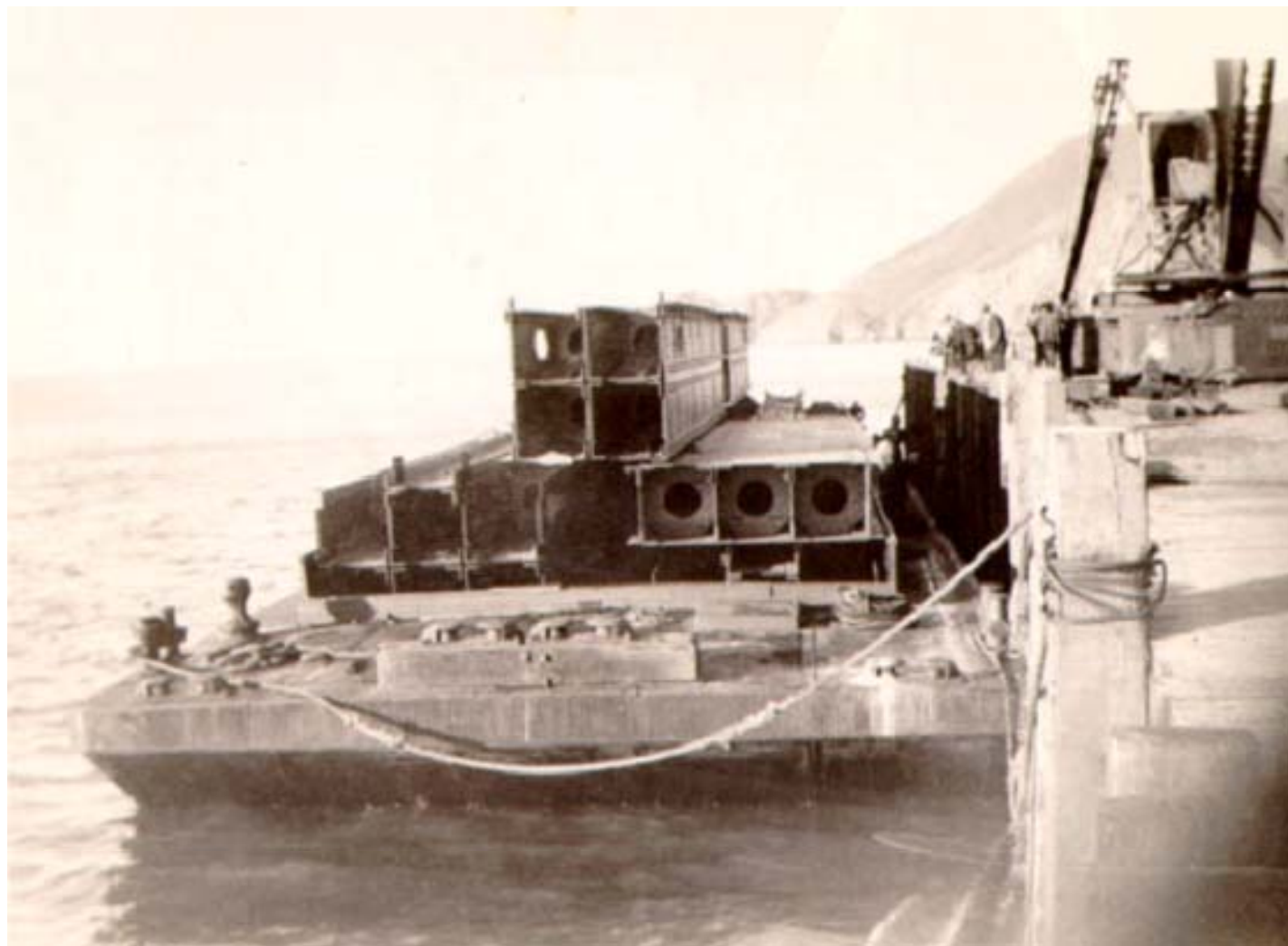
Barge with Steel Sections (adjoining pier)
