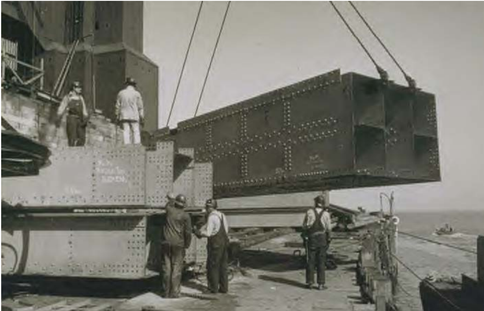
Tower Section on Pier (being lifted into position by creeper crane)
