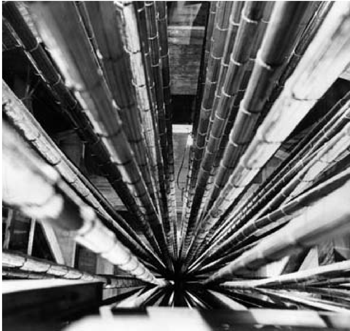
Individual Cable Strands (distributing to eye-bars within anchorage)
