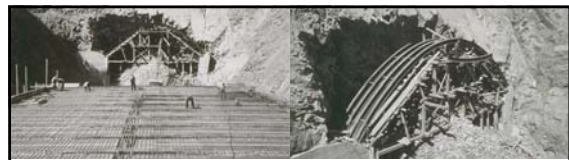
East Tunnel Portal May 1935
