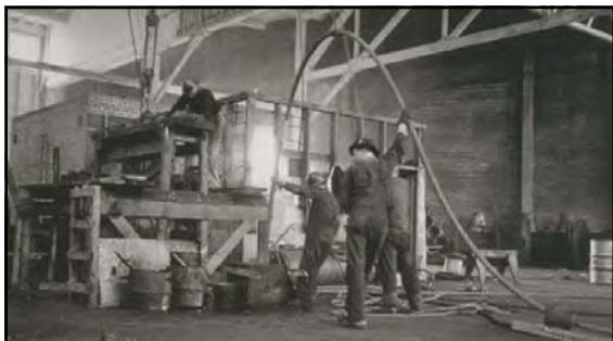
January 1936 Wire rope suspender "Pickling" process
