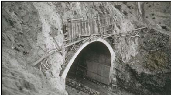
West Tunnel Portal December 1935
