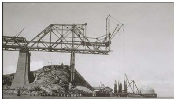
Pier E-1 (far left) / Pier E-2 (far right) May 1935
