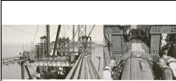
Central Anchorage North and South Cables (left) North Cable (right) October 1935
