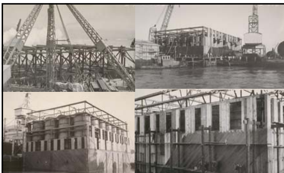
As the caisson descends, the sidewalls and cylinders are built-up
