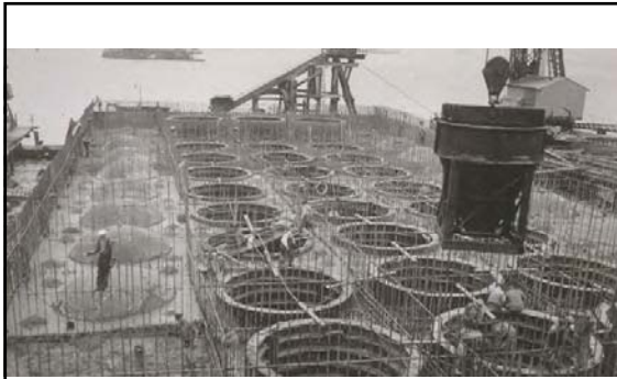
Pier W-4 August 1934
