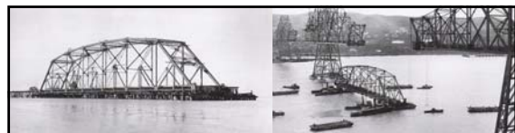
Carquinez-Strait Bridge Suspended Span
