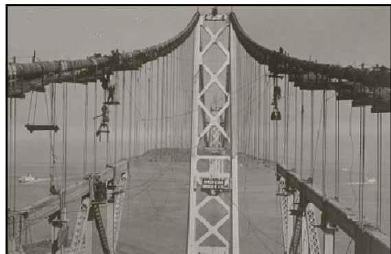
February 1936 Stiffening Truss extending from Pier W-1 towards Tower No.2 342
