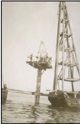
Preliminary Test Borings (1931)
