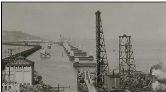
Piers E-22 thru E-14 (Oakland Approach) June 1934
