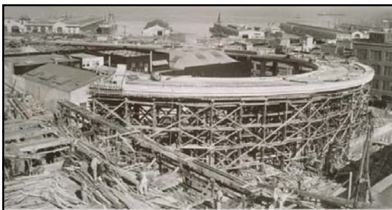
San Francisco Approach On Ramp (Span Nos. 38 thru 111 – Contract No. 15) April 1936
