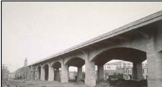
San Francisco Approach – Span Nos. 7 thru 18 The approach spans (and on an/off ramps) were built under Contract No. 15 (not Contract No. 3) November 1935
