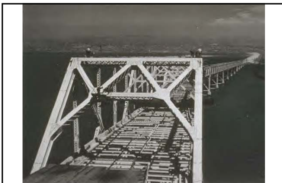
Span E-7 (Through Truss) – deck support in-place April 1935
