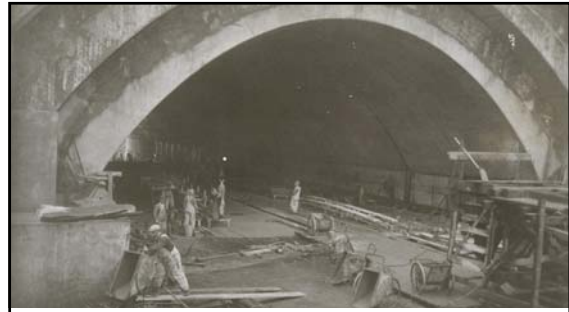
Tunnel Upper Deck (at West Portal) January 1936
