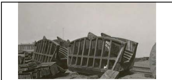
The two main cables were secured in-place by a pair of saddles (north and south) at Pier W-1's Cable Bent/s, Tower Nos. 2, 3, 5 and 6 and the Cable Bent/s at the Yerba Buena anchorage (pictured above). Each saddle was cast at a U.S. Steel subsidiary (in New Jersey) and weighed approximately 46-tons. At the time the Bay Bridge was built, the steel castings for the saddles were the largest ever made for a bridge project.
