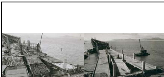
Lower Deck Concrete Girder Spans November 1934 (left) / January 1935 (right)
