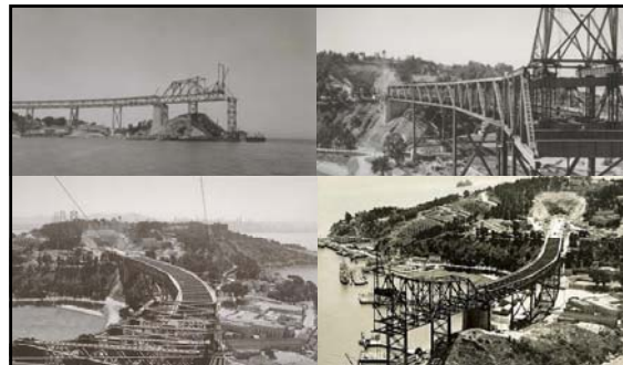
Yerba Buena Steel Viaduct (Deck Trusses) June/July 1935
