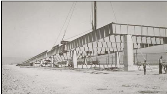
Plate Girder Spans (on Oakland shore) June 1935
