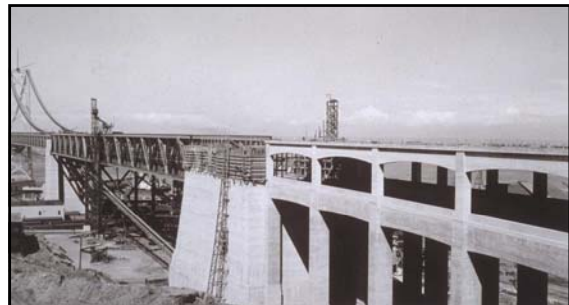
July 1936 Left to right: west suspension span / Pier W-1 / Steel Viaduct Spans / San Francisco Anchorage / Concrete Approach Viaduct
