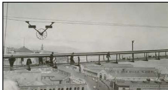
North cable traveler wheel in action The wheel had a cow bell attached to alert workmen of its approach August 1935
