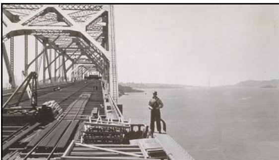
Through-Deck Truss Transition (atop Pier E-9) April 1935
