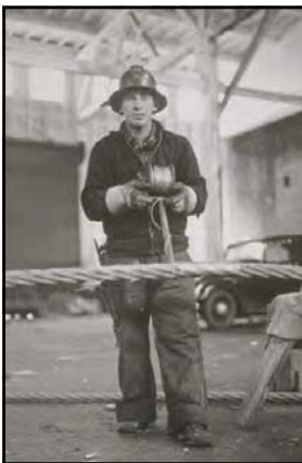
January 1936 Wrapping protective seizing around wire rope suspender. Rather than using a pair of suspender ropes (typical), the shortest suspenders of the four side-spans consist of short, fabricated steel shapes able to resist both compressive and tensile forces (the suspender ropes can only resist tensile forces). Under an unbalanced live load and due to the length of the side-span/s (1,160-feet), a stress reversal can occur requiring compression resistance at these locations.
