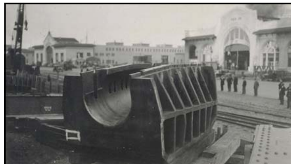
Cable Bent Saddle
