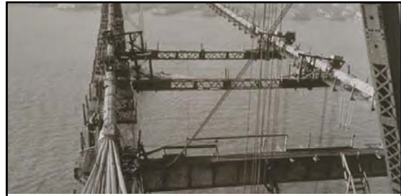
Lifting Struts (near the Central Anchorage) December 1935
