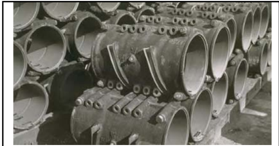
A cable band is a steel clamp consisting of two semi-circular halves bolted together around the main cable/s in corresponding positions. Welded to each half are slots; to secure the pair of suspender ropes which would be looped around each cable band for support of the suspended structure. There are a total of 612 cable bands.
