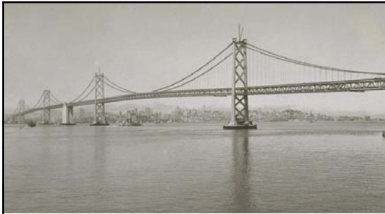
July 1936 All Stiffening Truss sections in-place
