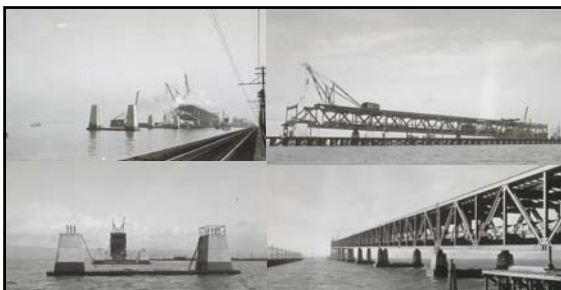
Direct (Pier) Supported Deck Truss Spans October/November 1934
