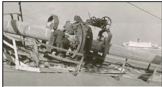
North Cable Compacting (between Central Anchorage and Tower No. 3) October 1935
