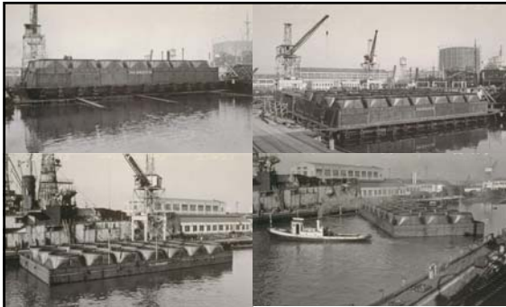
Caissons (at Dry Dock)
