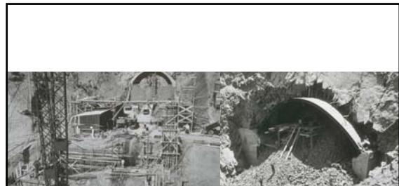
Yerba Buena Tunnel West Portal (left) / East Portal (right) September 1935
