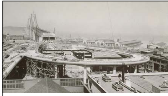
San Francisco On Ramp (Contract No. 15) June 1936
