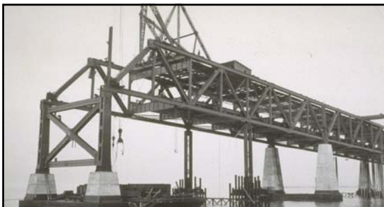
Deck Truss Span E-16 November 1934
