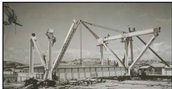
Unit No. 144 being assembled (at Islais Creek ) April 1936
