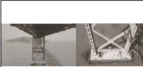
Pier E-5 with X-Braced Steel Tower August 1935
