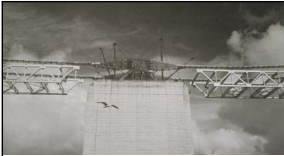
Central Anchorage March 1936
