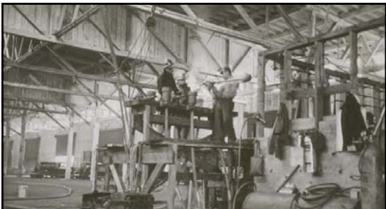
January 1936 Pouring zinc socket/s for wire rope suspender end/s
