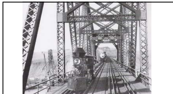
Southern Pacific's vintage C.P. Huntington, No. 1 , becomes the first train to cross the new $12 million lift bridge across Suisun Bay. Close behind is the first modern locomotive to cross the bridge.
