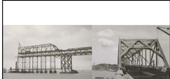
Through Truss Span E-8 (Pier E-9 - upper left) March/April 1935
