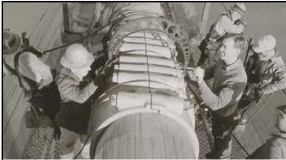
Checking strain in cable band bolts December 1935
