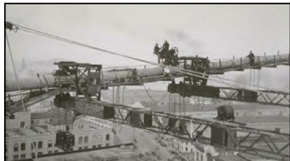
January 1936 Lifting struts (between Pier W-1 and Tower No. 2)
