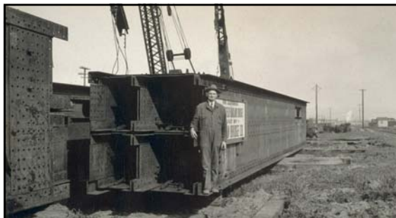
Tower No. 2 “Cells” February 1934
