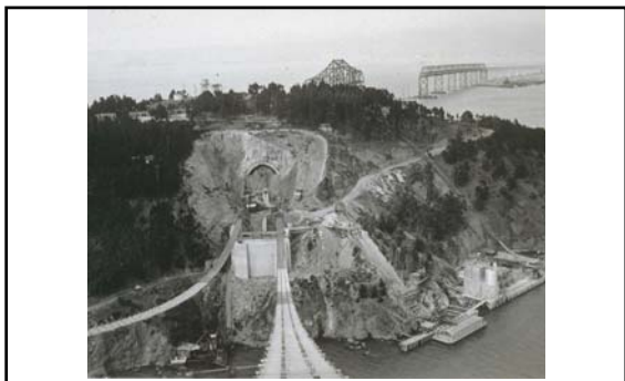
West Tunnel Portal (as seen from the south footbridge – concrete plant at lower right) September 1935 460
