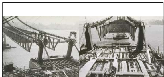
April/May 1936 Trusses extending from Y-B anchorage towards Tower No. 6
