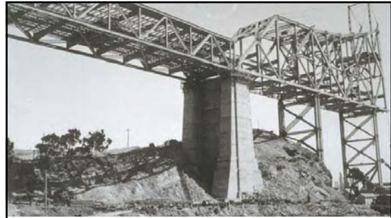
Pier E-1 July 1935
