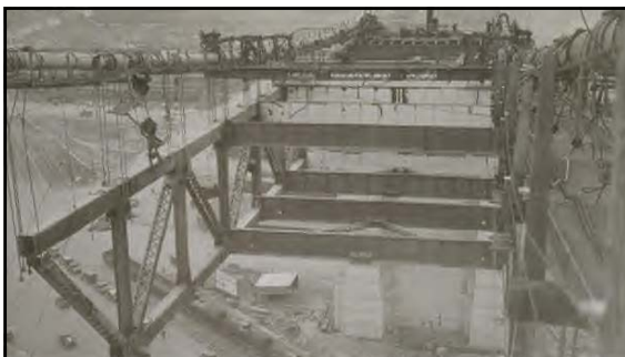
January 1936 Stiffening Trusses extending from Pier W-1 towards Tower No. 2 341
