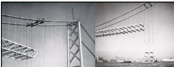
Lifting Struts (in action)
