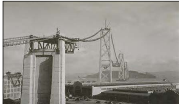
January 1936 Stiffening Trusses extending from Pier W-1 towards Tower No. 2 338
