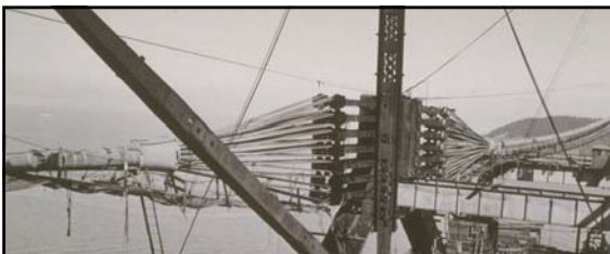
North Cable – Central Anchorage February 1936
