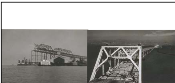
Through Truss Span E-7 March/April 1935
