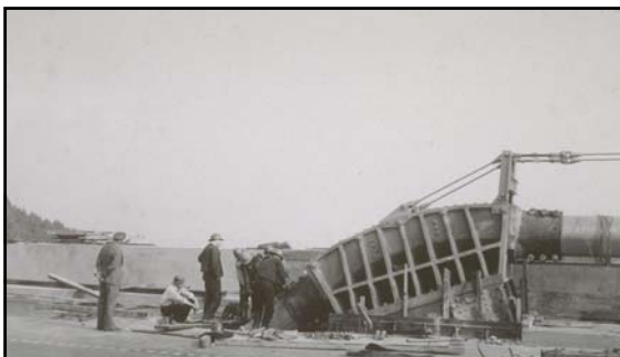
South Cable/Saddle – Yerba Buena Bent September 1936
