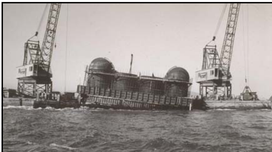
Pier W-6 (listing towards Yerba Buena Island) January 14 th 1934
