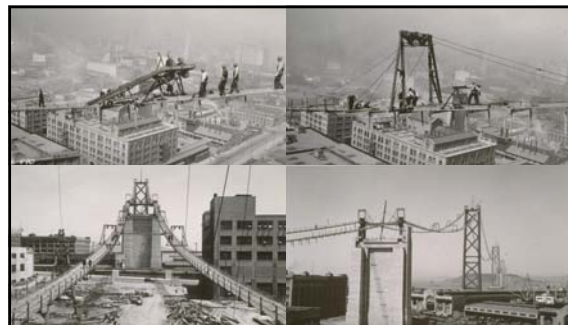
“Gallows” atop Footbridge/s (for support of the moving cable/traveler wheel) June 1935
