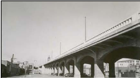
San Francisco Approach (Contract No. 15) September 1936
