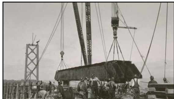
Central Anchorage A-Frame Section March 1935
