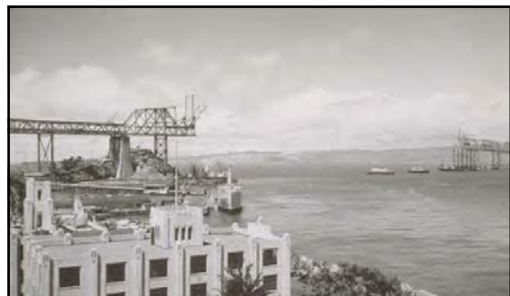
Piers E-1 thru E-5 (left to right) May 1935
