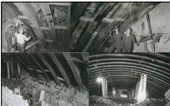
Steel Framing for Tunnel Vault April 1935 (top L&R) / June 1935 (bottom L&R)
