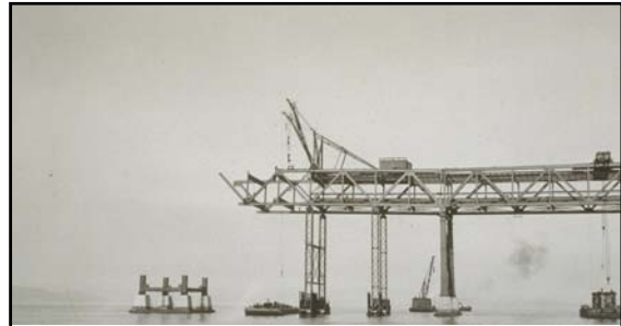
Deck Truss Span E-9 January 1935
