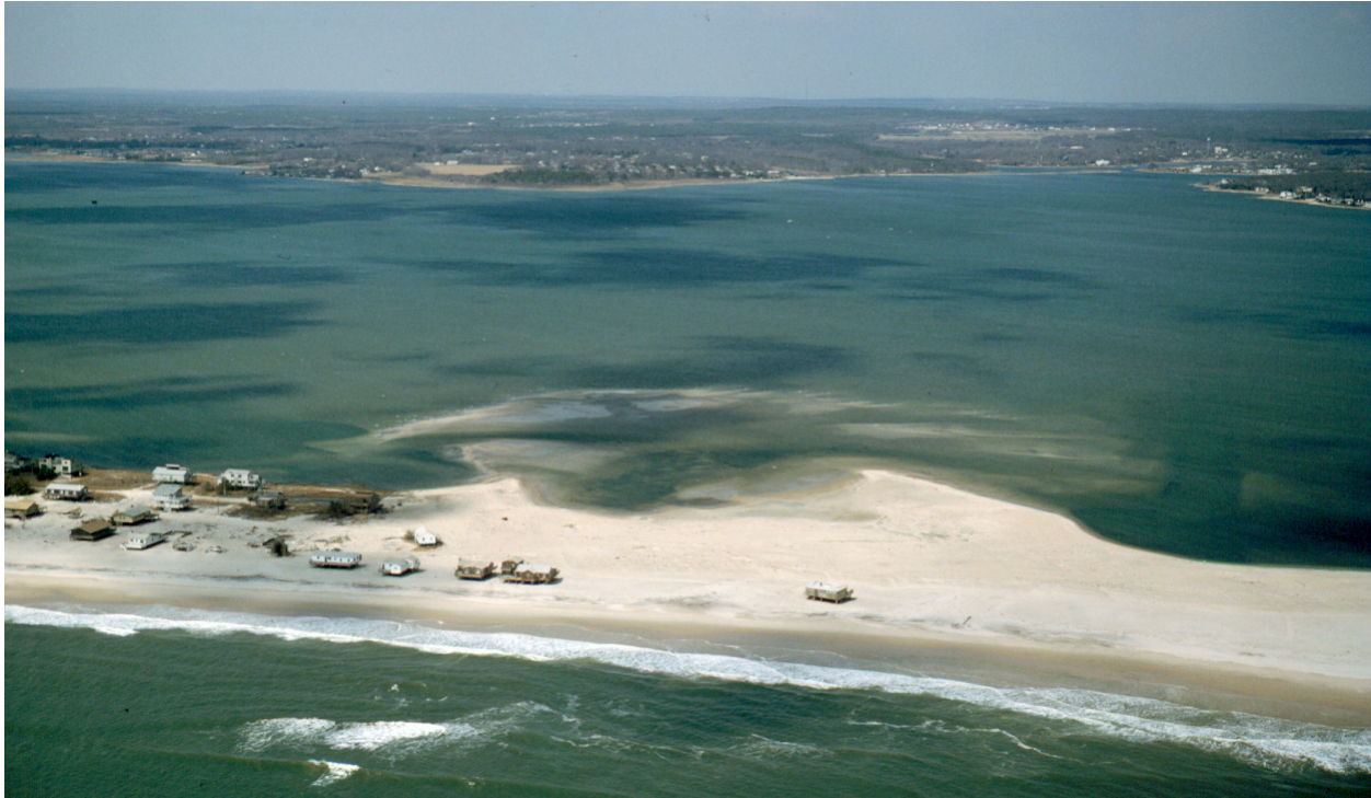
Figure IV-2-30. Westhampton Beach, Long Island, New York (March 1994 - view looking north towards Moriches Bay). In December 1992, the barrier island breached here during a northeaster, and 60 houses were destroyed. A large overwash fan can be seen in the bay, and to the left are houses that survived the storm. This is an example of the rollover mechanism, when sand from the ocean-facing shoreface is carried over the barrier and deposited in the back bay. The breach was repaired by the Corps of Engineers during 1993 using sand dredged from offshore. This low stretch of the barrier is particularly vulnerable, with several earlier breaches on record. In summer 1998, new homes were again being built here
