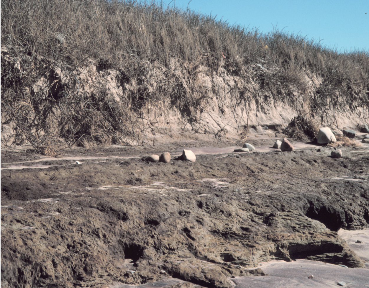
Figure IV-2-35. Peat horizon exposed on the shoreface, Ditch Plains, Long Island, New York (March 1998). The peat is in-situ, indicating that lagoonal sediments accumulated here before the barrier beach retreated over the marsh. The peat layer was about 1 m above the ocean water level at the time the photograph was taken. The dune resting on the peat is about 2 m thick
