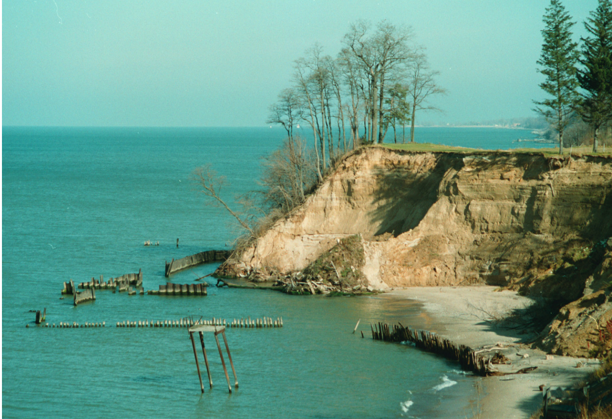
Figure IV-2-22. Lake Michigan shore south of St. Joseph, Michigan (November 1993). A triangle-shaped wedge of the bluff has recently slumped. The bluffs in this area have suffered rapid retreat, and many homes have been destroyed. At least three factors account for the erosion: (a) offshore downcutting of the till lake bottom; (b) wave attack on the bluffs; (c) ice expansion and lubrication of bedding planes caused by groundwater
