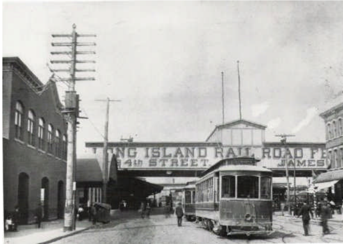
Ferry Terminal – Borden Avenue (now the entrance to the Queens Midtown Tunnel )
