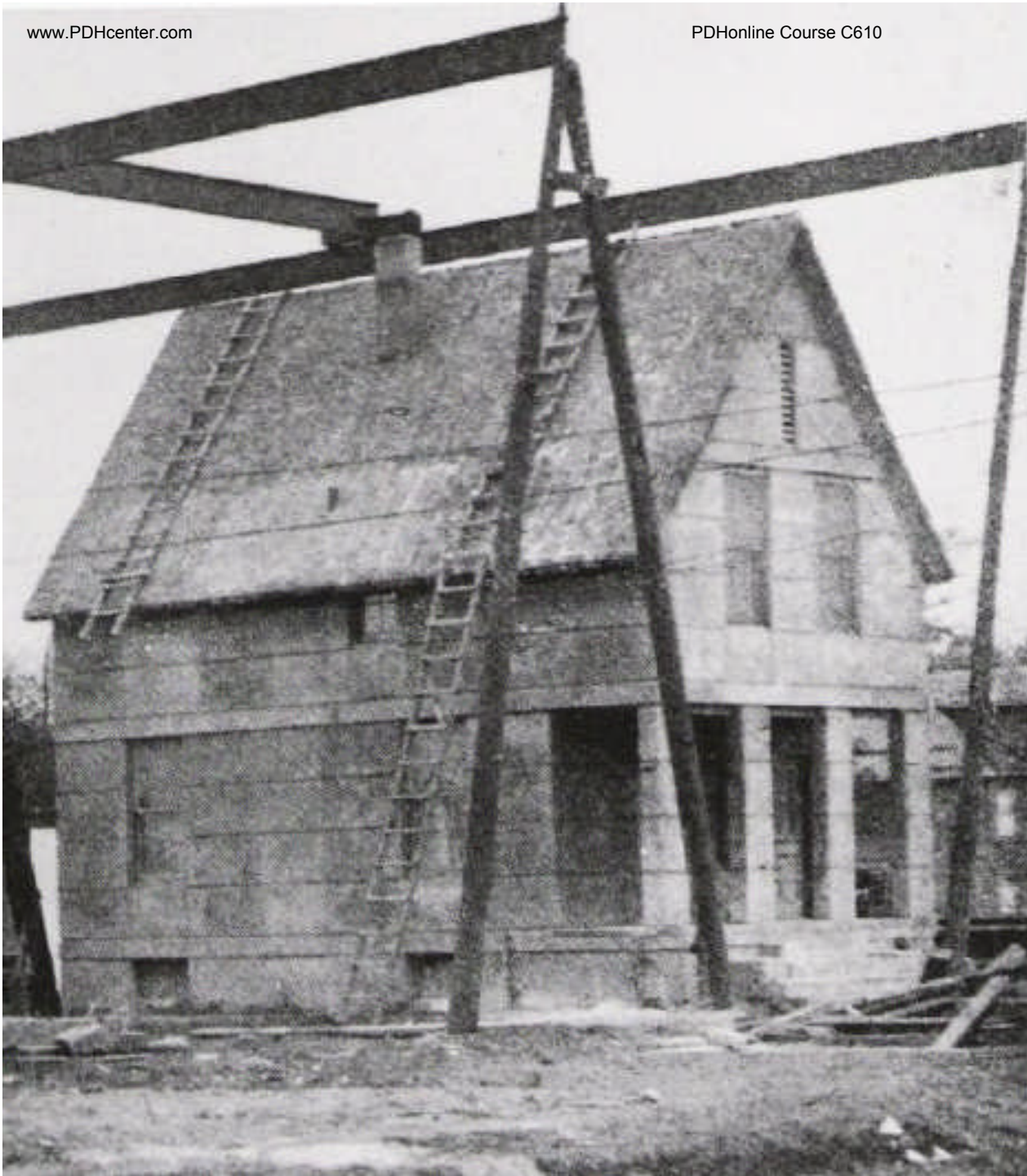
House under construction ca. 1911
