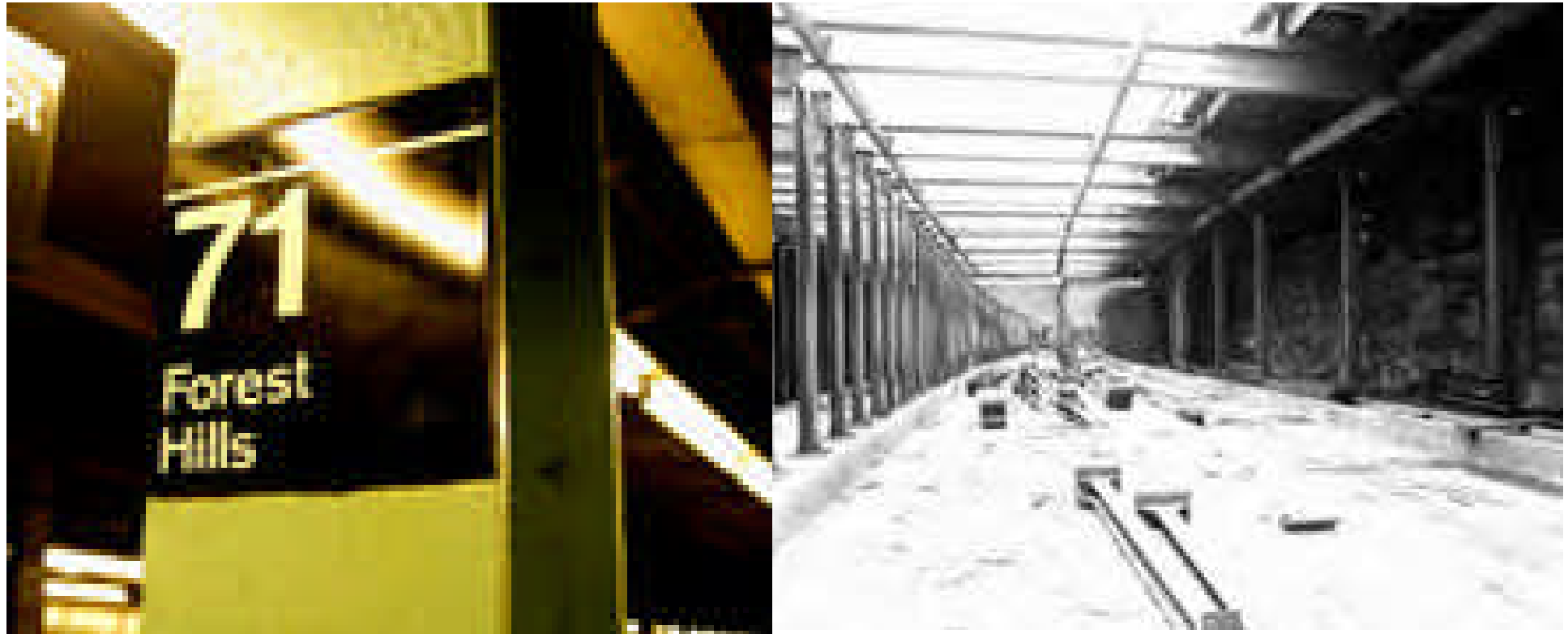
Subway line to Forest Hills & Jamaica under construction, mid-1930s
