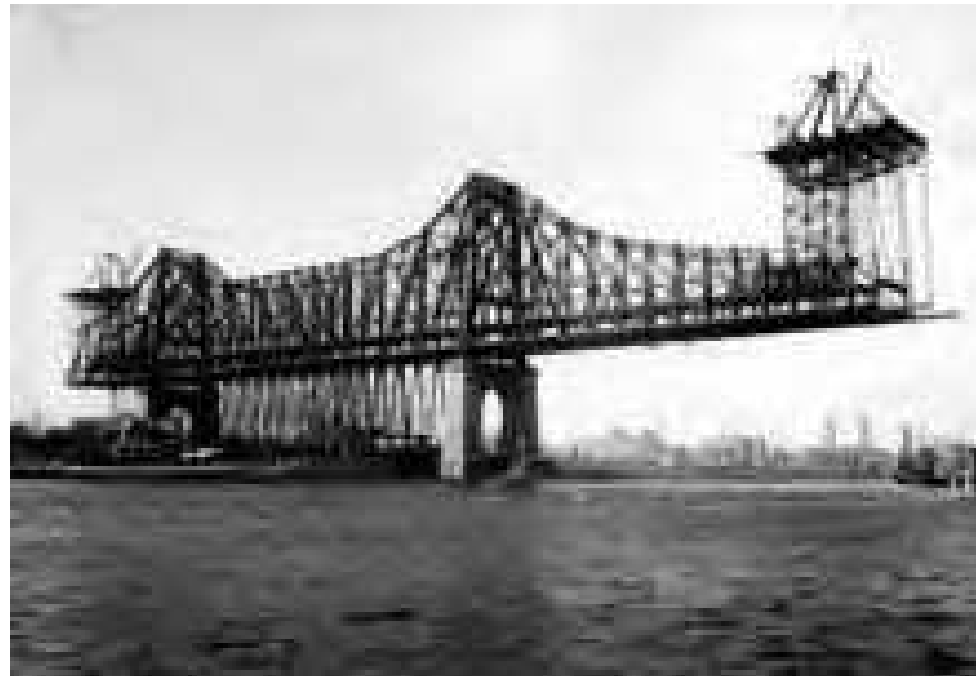
Queensboro Bridge under construction ca. 1908
