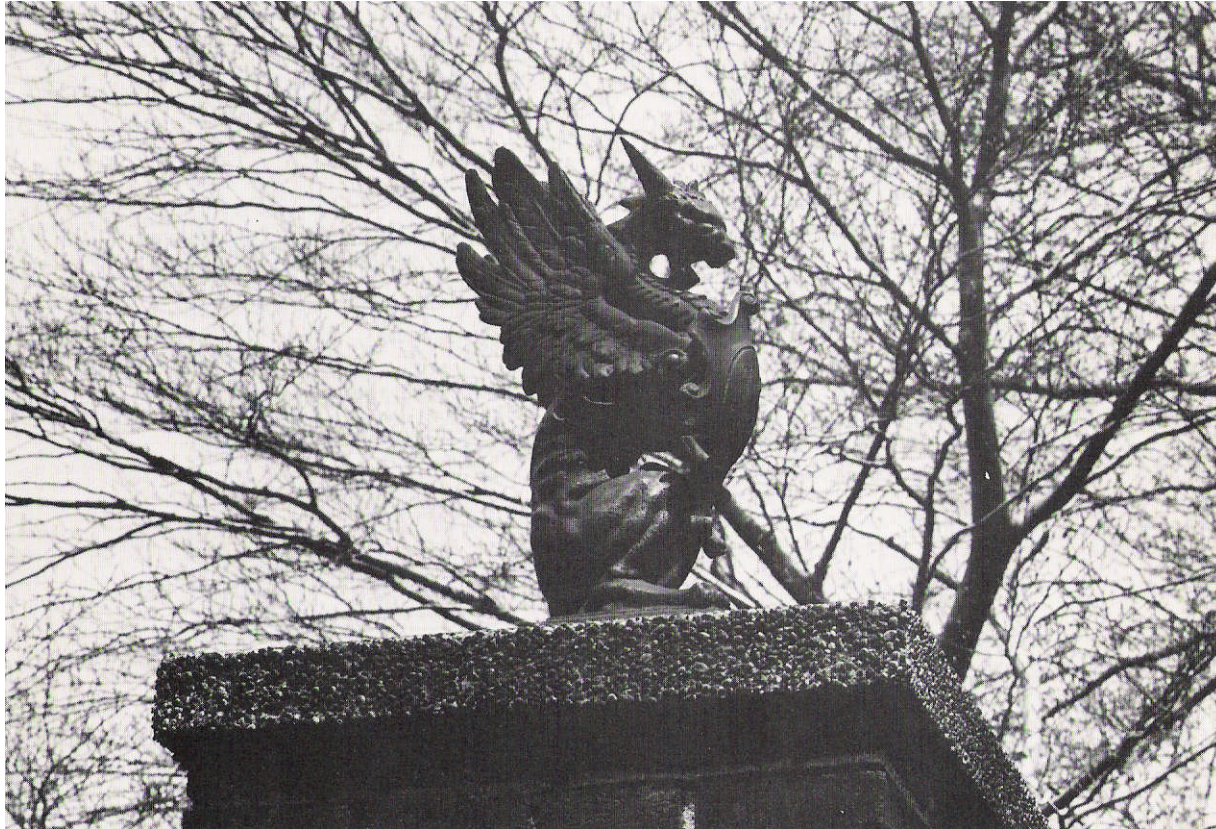
“Grotesque” atop masonry pier (Rockrose Place - Upper Gardens)
