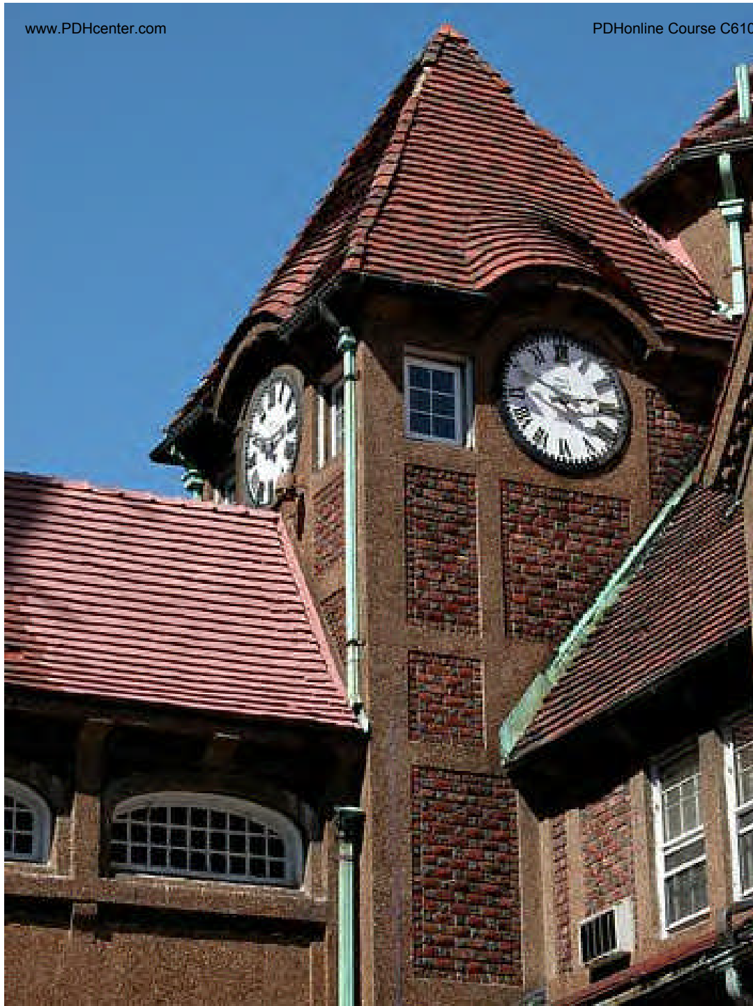
Pebbledash “half-timbering” (on pre-cast panels) Clock Tower - 10 Station Square
