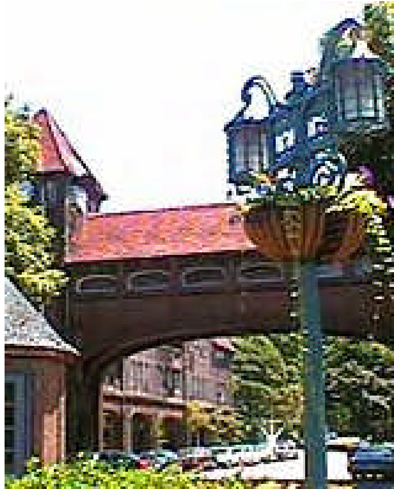
High Bridge portal (to Greenway Terrace) and adjacent Clock Tower (as seen from island in the middle of Station Square - east kiosk at lower left)
