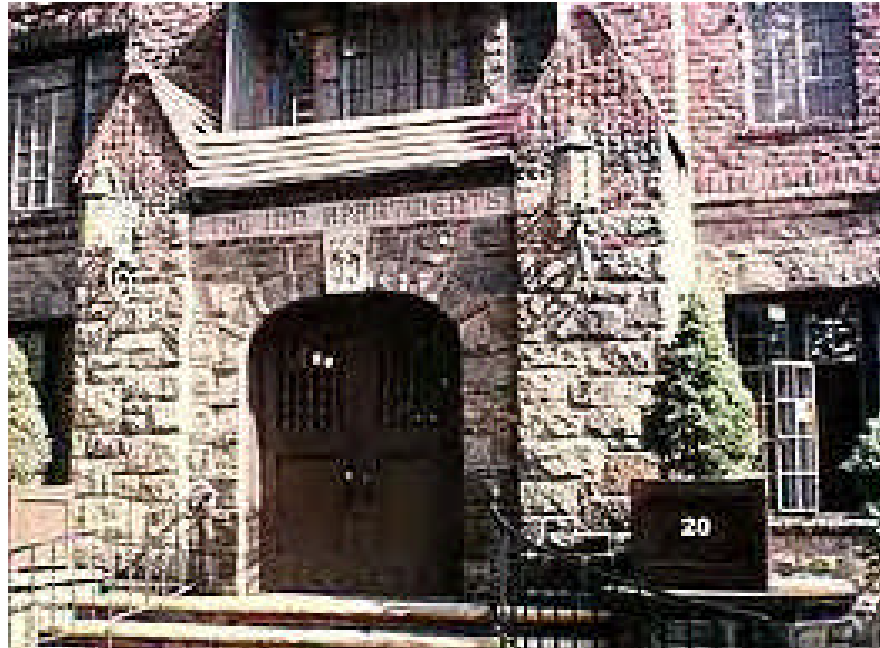
20 Continental Avenue Lobby Entry
