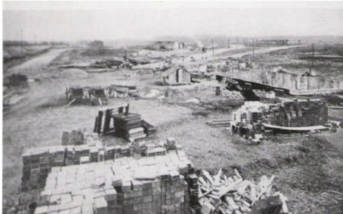
Station Square under construction (ca. 1911)
