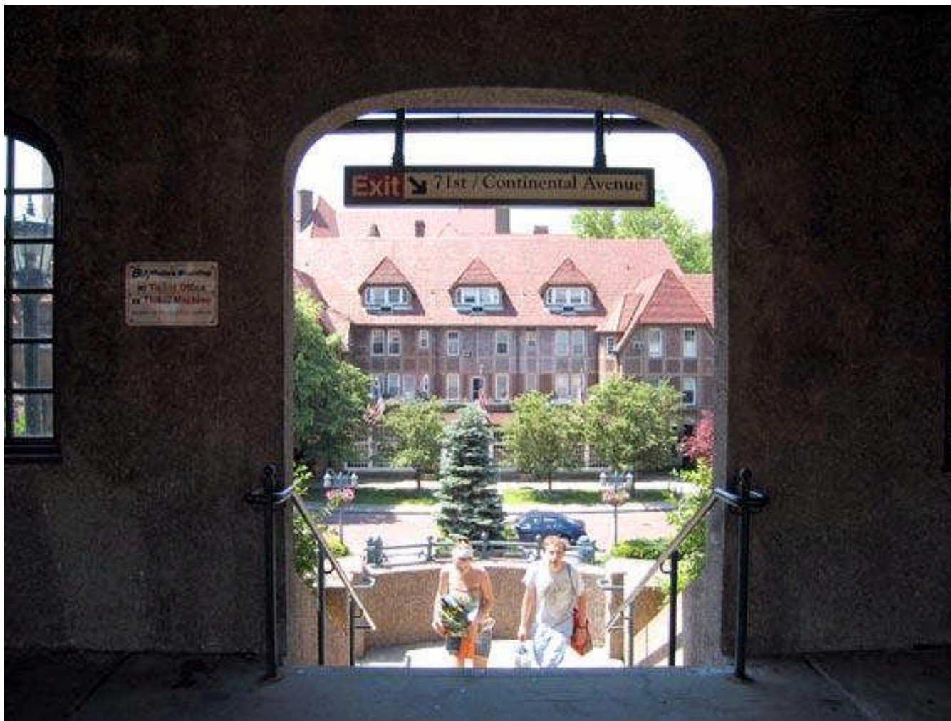
Station Square and the station's balcony – as seen from the LIRR's east-bound platform
