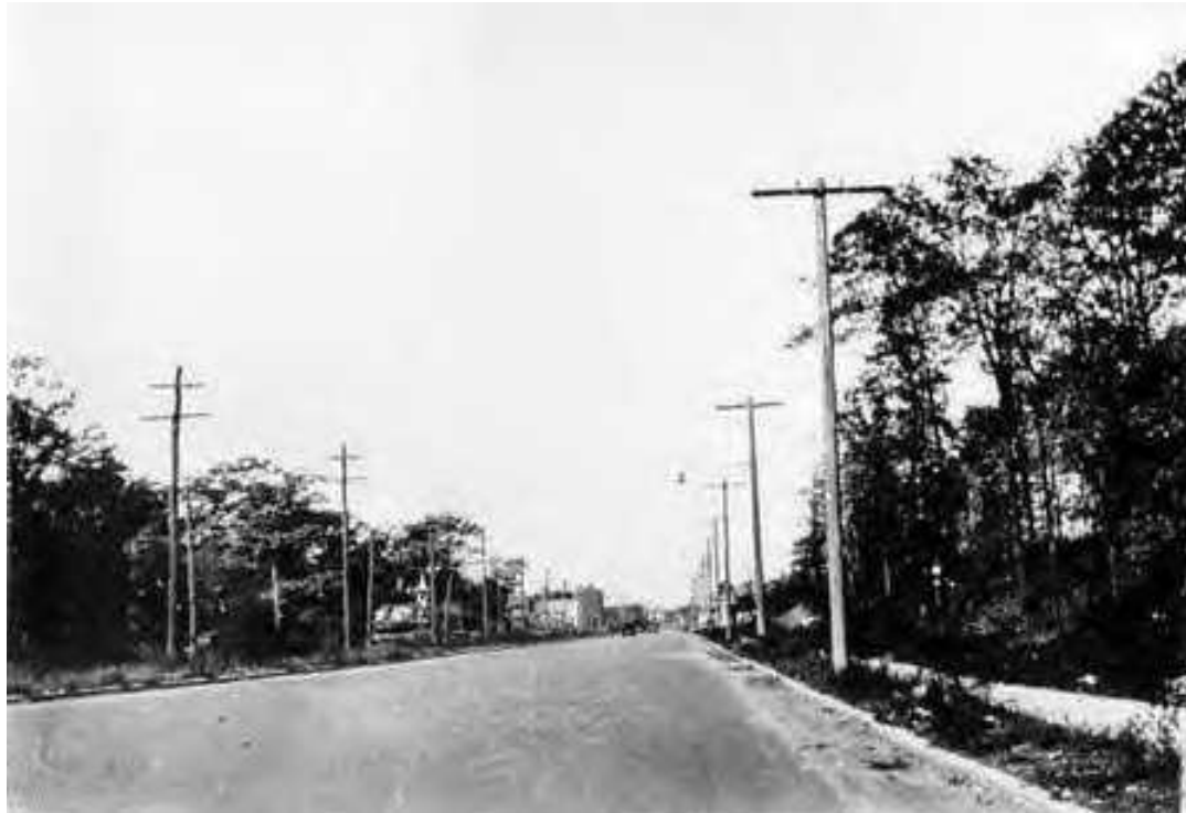
Queens Boulevard (before widening)
