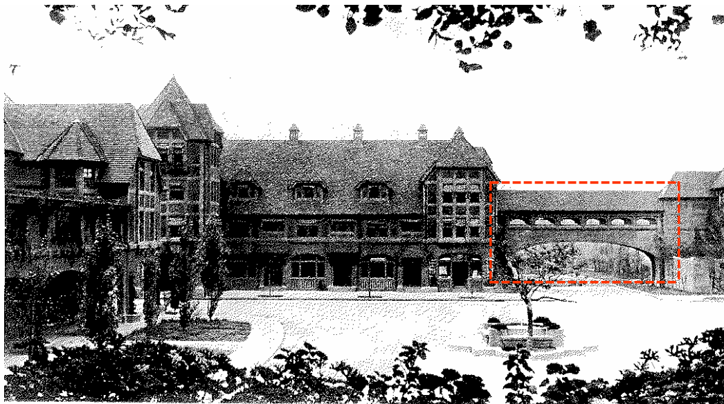
View looking west towards 2 Dartmouth Street and Burns Street/LIRR bridge
