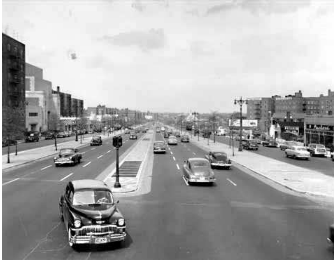
Queens Blvd. ca. 1950 (Rego Park)
