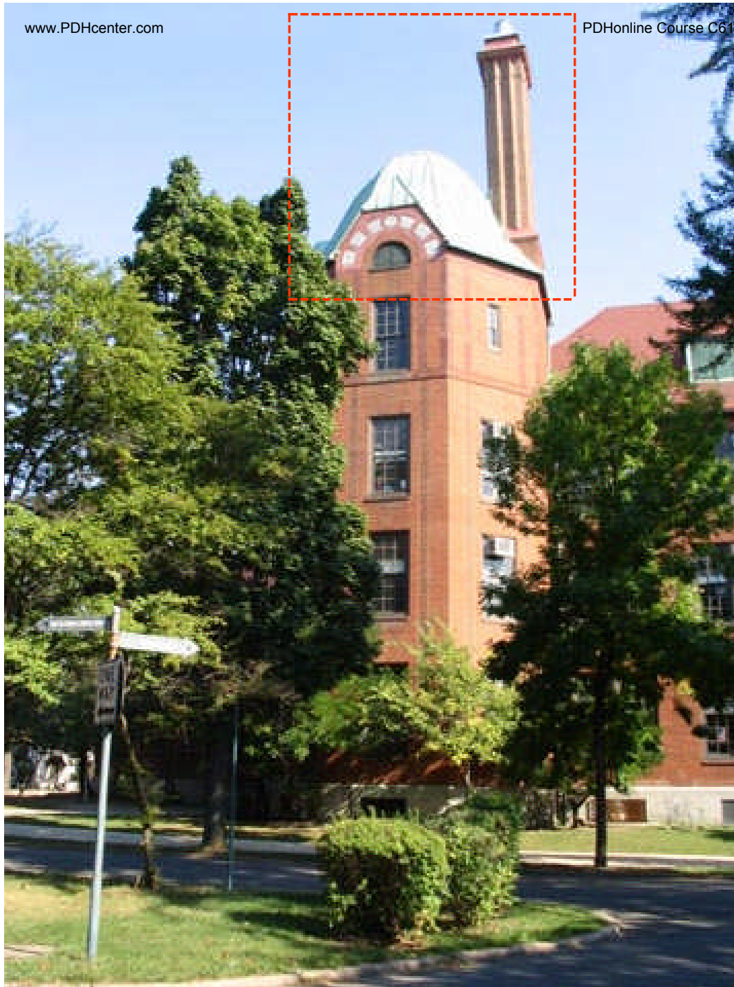
Four-story tower with copper-clad turret roof and prominent chimney
