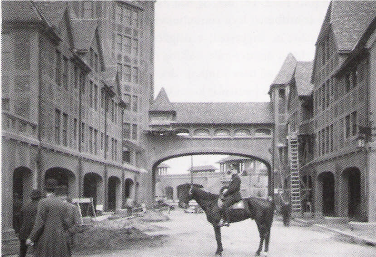
One Station Square (left) & Ten Station Square (right) under construction ca. 1911
