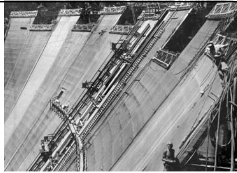
Looking across the downstream face of the dam at top of forms (toward Nevada side). Cooling system header pipes seen in middle (July 1934).
