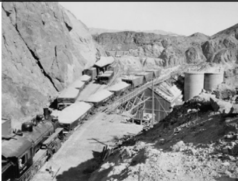
Train at concrete mixing plant
