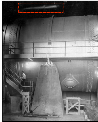
View of the 25-foot pipe in the upper Arizona Penstock header tunnel from the construction adit. The ventilating pipe can be seen in the upper portion of photo (July 1937)
