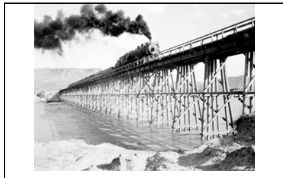
Gravel train crossing a trestle on the way to BCP site (May 1932)
