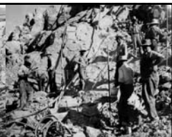
Left: blasting in power plant location/s (in dam foundation excavation and on canyon walls above power plant location). This was the last of the major blasts prior to the beginning of actual concreting operation in the dam structure proper (May 1933).
