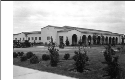
The Annex Building (of the Main Administration Building) in Boulder City
