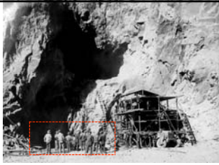
Drilling the first round in enlarging upper portal of Diversion Tunnel No. 2. The welded steel "Jumbo" mounted on the truck has twenty five air drills on it (the swing shift crew is waiting to go to work in the lower left of the photo; November 1931). Holes for explosives were bored into the rock using pneumatic drills. Five hundred pneumatic drills, hoses and compressors were purchased from Ingersoll Rand for the BCP. Compressor plants were installed just below the outlet portals and upstream near the inlet portals. Compressed air was taken to the work sites through a network of pipes two to six inches in diameter. 273
