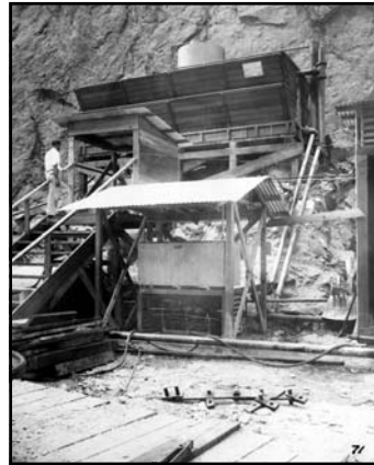
Frigidaire drinking water and water cooling plant (at compressor No. 2, Arizona side; August 1931)
