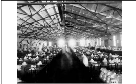
Anderson Mess Hall, Boulder City - North Wing Dining Room (seating capacity was five-hundred in each wing; September 1931) 229
