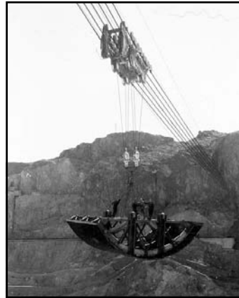
The 150-ton cableway transporting Penstock header tunnel lining forms into canyon (September 1933)
