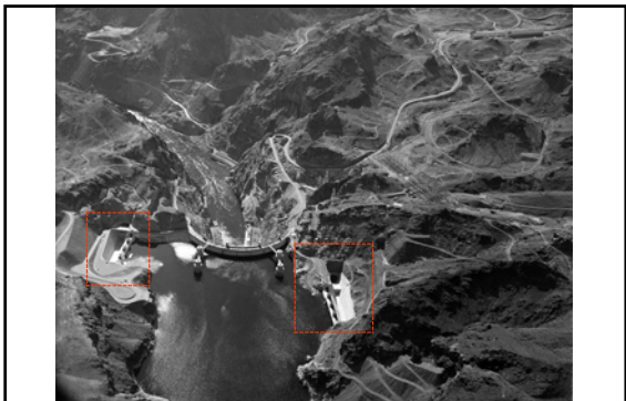
Aerial view of Hoover Dam showing Intake Towers, Spillways and roadways (October 1947)
