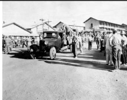
Workmen loading-out for the canyon on the day shift (in front of the Six Companies' Mess Hall, Dormitories in background)
