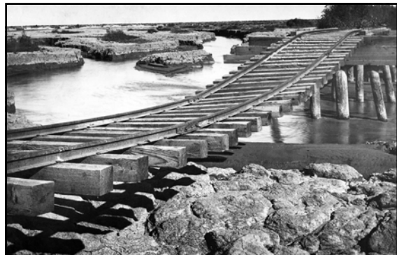
View shows where the Southern Pacific railroad tracks were cut into and washed out (September 1906)
