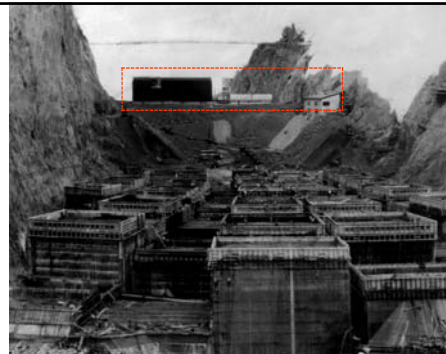
Cooling Tower and Refrigeration Plant (atop crest of the downstream cofferdam; September 1933)
