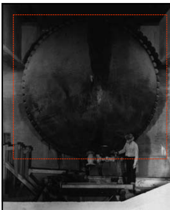
Temporary bulkhead (on the thirteen-foot penstock for Generator No. 5; December 1941) in the Arizona powerhouse. The bulkhead was placed on the Penstock at the time of its construction.
