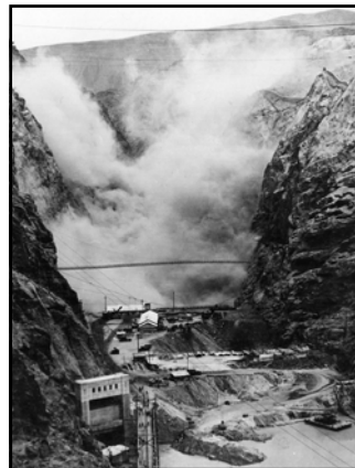
Left: blasting in power plant location/s (in dam foundation excavation and on canyon walls above power plant location). This was the last of the major blasts prior to the beginning of actual concreting operation in the dam structure proper (May 1933).
