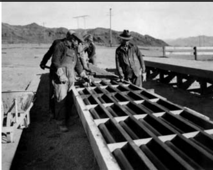
Yard for manufacturing porous drain tiles for the Spillways (January 1933)
