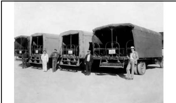
“Covered Wagons” (each having a capacity of forty-eight men) were used to transport workmen from Boulder City to Black Canyon. The trucks’ canvas-covered side curtains could be raised during hot weather. 97
