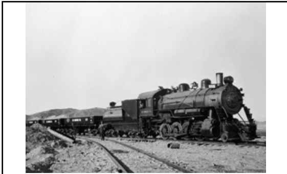
First train load of gravel arriving at screening plant (January 9 th 1932)
