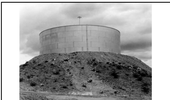
Boulder City water supply tank (May 1932)
