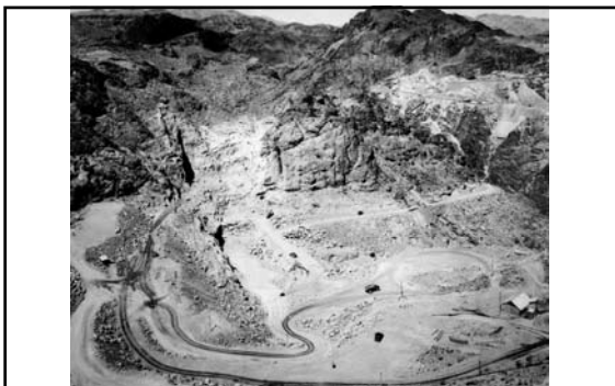
Six Companies constructed muck roads and spoil dumps (June 1932)
