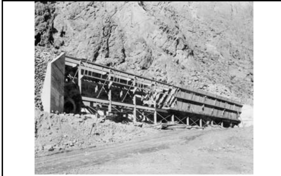
Aggregate bins at Six Companies' Low-Level concrete mixing plant. Conveyor to mixing plant operates from end (at left; Dec. 1931) 577
