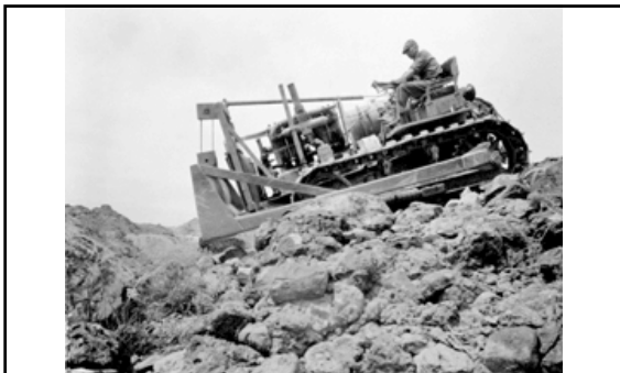
Caterpillar tractor at work (March 1932). Caterpillar introduced its first diesel powered tractor; the "Diesel Sixty," in 1931 (shown above). It was used extensively on-site at the BCP. 251
