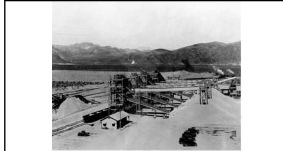
Since gravel (aggregate) and sand were the only materials not provided by the federal government, Six Companies had to provide these key ingredients for the concrete mix. Thus, an aggregate washing, classification and storage plant was established (at Hemenway Wash). Aggregate up to nine-inches in diameter was used in BCP concrete. 572
