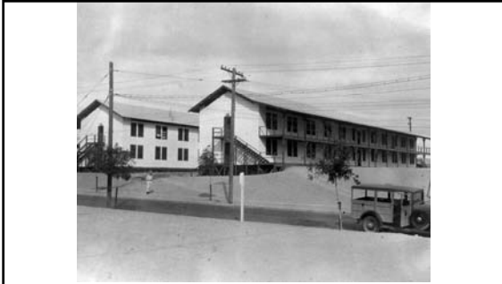
Typical dormitory housing employees of Six Companies. Each dormitory of this type (of which there were eight) housed 172 men in separate rooms, all of which were equipped with an air cooling system (October 1933). 223
