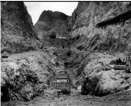
First forms for Hoover Dam (looking downstream; June 1933) 633
