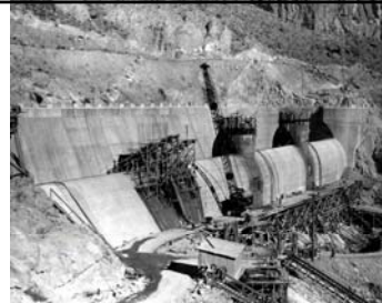
Nevada spillway (view from the construction trestle over the Nevada Intake Towers (November 1933). Each Spillway consisted of a concrete-lined open channel approximately 650-feet long, 150-feet wide, and 170-feet deep on each canyon wall. More than 600K cubic yards of rock were excavated for the Spillways. The Spillway walls were lined with eighteen-inches of concrete and the floors with twenty-four inches. A total of 127K cubic yards of concrete were placed for the Spillways.
