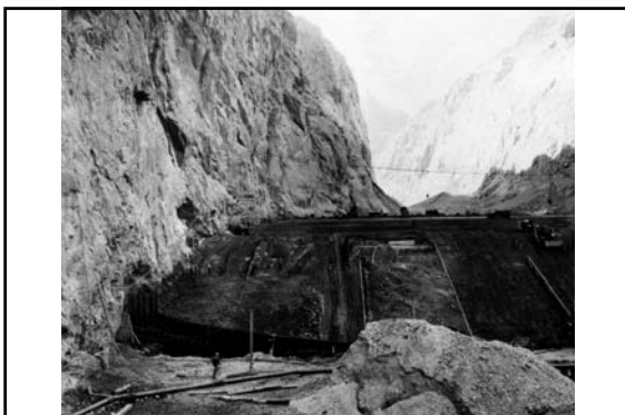
Upstream Cofferdam (looking downstream; Dec. 1932)
