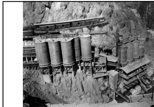
Hi-Mix and cement blending plants (with unloading track and aggregate bins above; April 1934) 580
