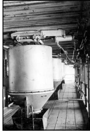
Sand and coarse aggregate batchers on upper batching deck at Six Companies' Low-Level concrete mixing plant (April 1932)
