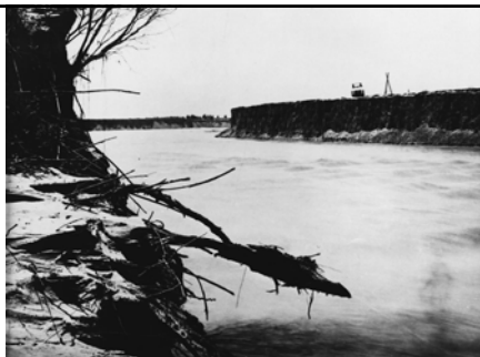
Cut banks in the new river canyon (at the ferry four miles northeast of Brawley, California). The photo above shows the Colorado River when it was out of it's banks and flowing across Imperial Valley to form the Salton Sea (August 1906)
