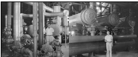
Left : pump units for cooling system (Compressor House; July 1935) Right : exchange units for cooling system (Compressor House; July 1935)
