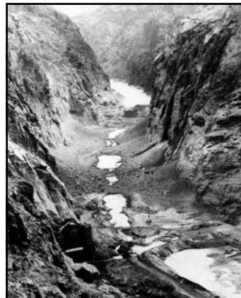
Looking upstream in Black Canyon (from lower portals) showing Lower Cofferdam site and general conditions after diversion of the Colorado River (November 1932)
