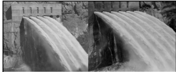
Left: 9Kcfs pouring from the Arizona Outlet Works 180-feet to river below (October 25 th 1936) Right: Six valves in Arizona valve house discharging 23Kcfs (valves were 100% open; April 12 th 1937)
