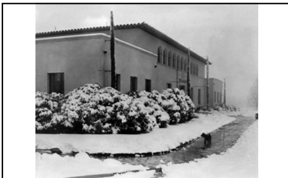
Rear view of the Administration Building covered with a four-inch blanket of snow (February 1939) 99
