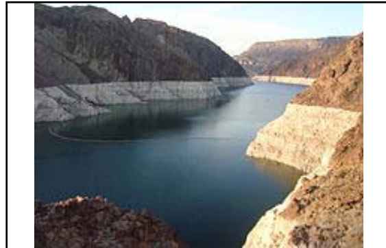
View upstream from Hoover Dam (July 2009) shows that the water level has decreased drastically 890
