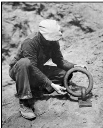
Old Ring Bolt anchored in rocks on the Arizona shore of the Colorado River (near Jumbo Wash, below Hoover Dam). These rings were used by early navigators as cable anchors to assist the boats through swift waters. The bolt was probably set shortly after the end of the Civil War. 105
