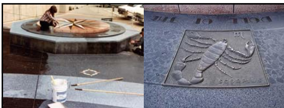
Left: crew applying a coat of sealer to the Star Map's raised Compass and surrounding Zodiac (on octagonal platform; February 1982) Right: Scorpio plaque on Zodiac
