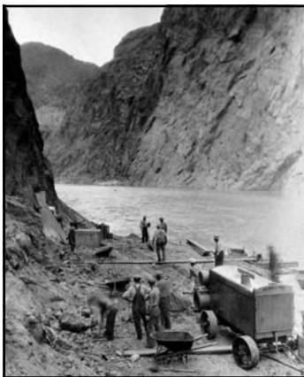
Leveling bar at Arizona abutment (for compressor plant) to drill Adits to Diversion Tunnel/s (April 1931)
