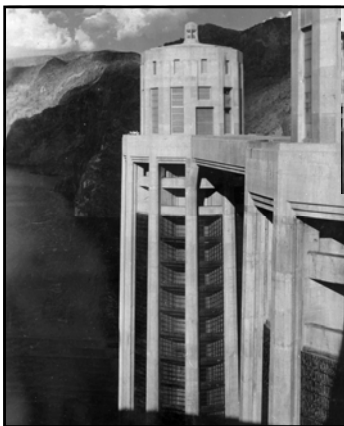
Left: the Arizona Intake Towers as seen from the crest of the dam (September 1936). Above: Boulder Canyon. Looking upstream from the top of Hoover Dam. Arizona Intake Towers at left (April 1938).
