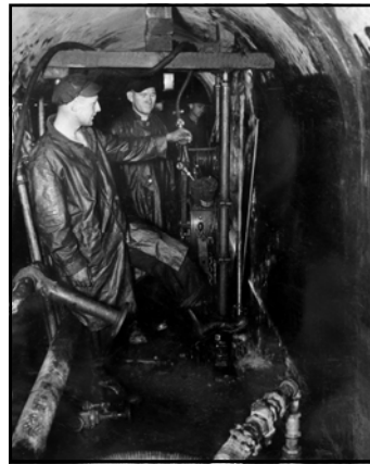
Diamond drill crew working on center hole A-4 (located at the approximate center of the inner gorge in the 553 gallery; June 1939)
