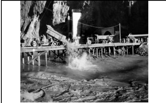
Dumping materials at temporary pile (trestle) bridge to complete diversion of the Colorado River (after blast; November 13 th 1932)
