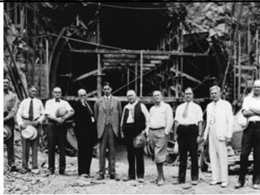
Inspection party in front of the outlet portal of a diversion tunnel. City Manager Sims Ely, Construction Engineer Walker Young, Six Companies Director H.J. Kaiser, Interior Secretary Ray Wilbur, Six Companies President W.A. Bechtel, MWD Engineering Chairman W.L. Honnald, Six Companies Director S.D. Bechtel, MWD President W.P. Whitsett, Six Co. Superintendent Frank Crowe (September 1932).
