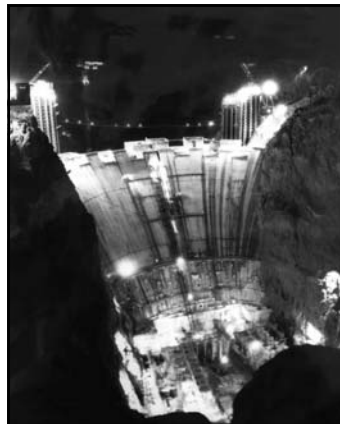
Hoover Dam construction at night (as seen from Lookout Point; September 1934).
