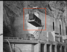
Loaded freight car on platform being lowered over 150-ton cableway into position at Nevada wing of power plant (November 1935)
