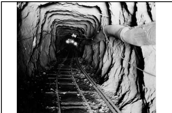
Arizona tunnel Adit (June 1931)
