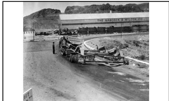
The 200-ton capacity La Crosse trailer used in transporting pipe sections from plant to dam slips on super-elevated roadbed between Boulder City and the Babcock and Wilcox Company plant (July 1934)
