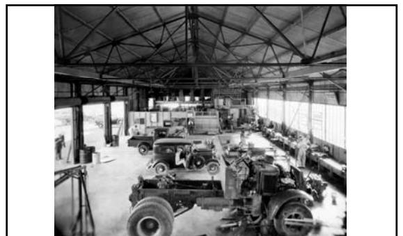
Interior view of Six Companies' garage and automobile repair shop in Boulder City. Complete facilities were installed for overhauling all classes of equipment (August 1932).
