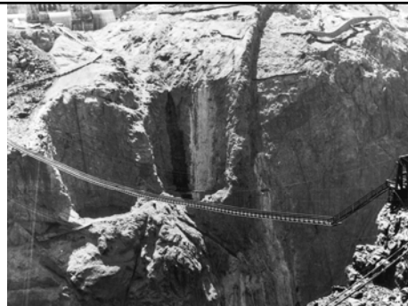
Cat-walk spanning canyon over Upstream Cofferdam (August 1933)
