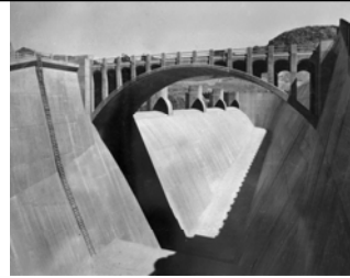
Open channel of the Arizona Spillway and the Highway Bridge (as seen from atop the arch of the inclined tunnel; September 1936). The Spillways each have a capacity of 200Kcfs totaling 400Kcfs. If the Spillways were operated at full capacity, the energy of the falling water would be about twenty-five million horsepower. The flow over each Spillway would be about the same as the flow over Niagara Falls, and the drop from the top of the raised Spillway gates to river level would be approximately three times as great as Niagara Falls.
