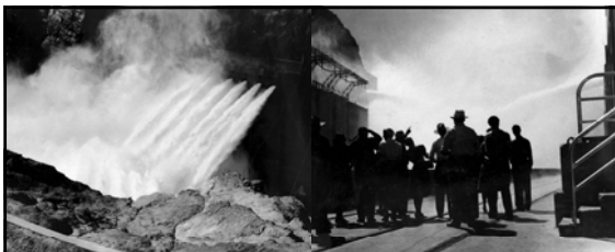
Left: view of the Nevada canyon wall Valve House showing all of the 84-inch needle valves open (September 28 th 1940) Right: a few visitors braved the spray on the central section Powerhouse ramp to watch the Valve Houses' needle valves in full operation (September 28 th 1940) 723
