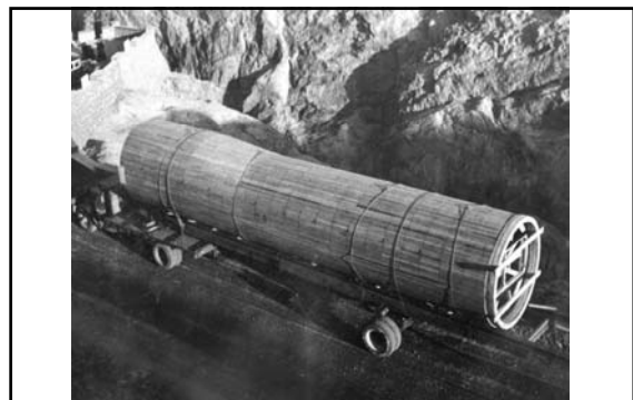
Form for radial Inspection Gallery en-route to Hoover Dam (December 1933) 360
