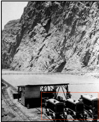
Six Companies Compressor Station (Arizona side; June 1931)
