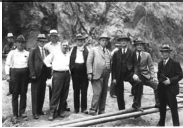
Group of notables who witnessed the pouring of the first concrete in Hoover Dam. Left to right: H.J. Lawler - Director, Six Companies Inc.; Walker R. Young - Construction Engineer, U.S.B.R.; Frank T. Crowe - General Superintendent, Six Companies Inc.; C.A. Shea - Director of Construction, Six Companies Inc.; W.A. Betchel - President, Six Companies Inc.; R.F. Walter - Chief Engineer, U.S.B.R.; Theodore A. Walters - First Assistant Secretary of the Interior; Ed Clark and C.P. Squires - members of the original Colorado River Commission . 189
