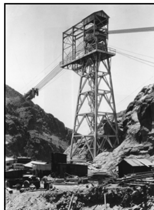
Head-tower of permanent 150-ton cableway (June 1933)
