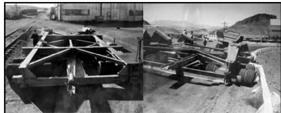
Two hundred-ton capacity (two-way) La Crosse trailer (for transporting sections of thirty-foot penstock pipe; July 1934) 252
