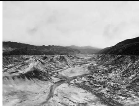
Empty reservoir after St. Francis Dam failure
