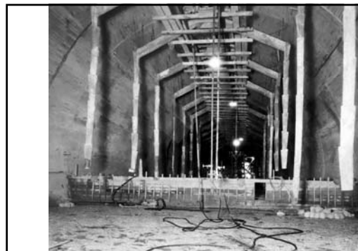
View taken from the upstream end of No. 4 Plug, looking downstream (showing method of pouring; April 1935) 538
