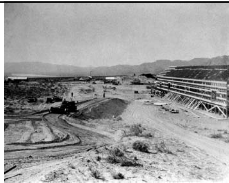
Six Companies warehouse and spur track (under construction; March 1931)
