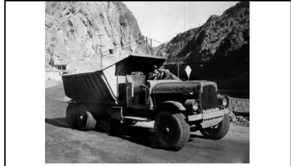
A Moreland truck of twelve cubic yards capacity, used in hauling muck from upper portals of the Diversion Tunnels. This truck has dual rear axle. (note the wire mesh protection over the hood and the protected headlights; January 1932). 248
