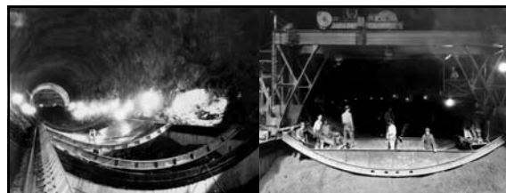
Left: first forty-foot slab of concrete poured in the lining of the Diversion Tunnel/s (March 1932) Right: movable template used in forming forty-foot slabs of invert lining (April 1932) 480
