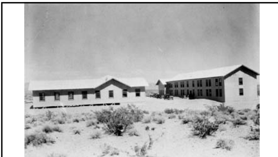
Six Companies office building (left) and dormitory (right; June 1931) 227
