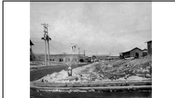
Indicative of the wide range of temperatures at Boulder City (which reaches 115-degrees in the summer), this photograph shows what was officially reported as the third snowstorm in seventeen years. The temperature dropped to 24-degrees (November 1931). 98
