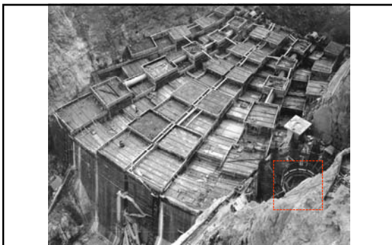
The dam as seen from construction trestle above Nevada Intake Towers (downstream Nevada Intake Tower seen in lower right; Nov. 1933)
