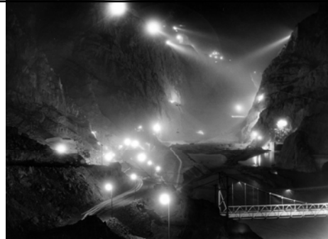
Night work at the dam site
