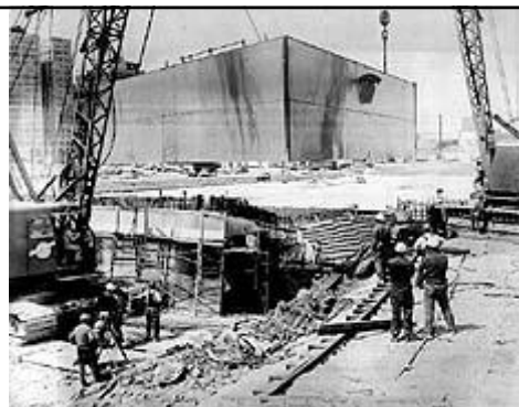
The first leg section being lowered onto the foundation (February 12 th 1963)
