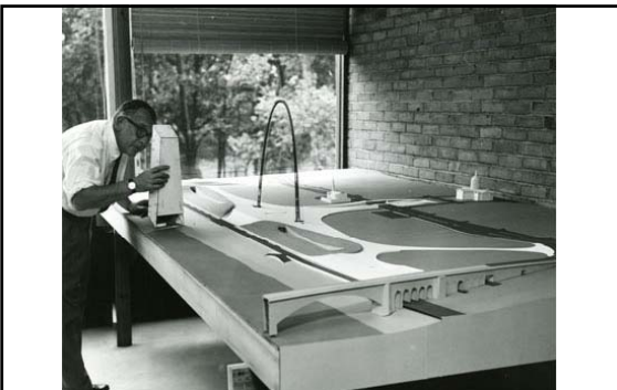
In his studio, architect Eero Saarinen using a scanning device to study a model of the Jefferson National Expansion Memorial , May 1961
