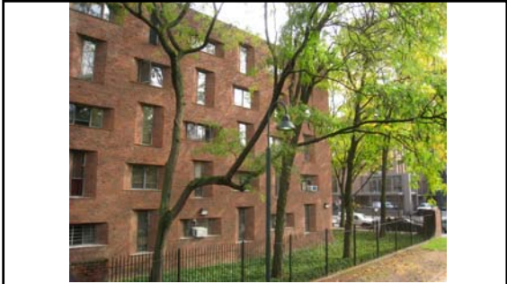
Hill College House (1958). One of the largest college houses (undergraduate dormitories) at the University of Pennsylvania . The building was unusual for its time, incorporating an interior atrium. In common with other buildings constructed at the height of the Cold War , the basement contains a fallout shelter, which links to the university's utility tunnels. 277
