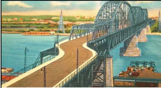
MacArthur (formerly St. Louis Municipal ) Bridge (1912)
