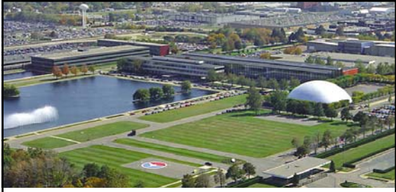
The General Motors Technical Center in Warren, Michigan had futuristic nuances. GM's Chief of Design Harley Earl conceived of the idea, picked the location and chose the local architectural team of Eliel and Eero Saarinen to design it. Before completion, the complex was christened: "The Versailles of Industry" and the name stuck. It was nationally heralded in the media at its opening in May 1956. The twenty-two acre lake was a central element of the Tech Center. On the west side was a gigantic fountain that formed a wall of water 115-feet long and 50-feet high. A smaller decorative fountain, designed by the sculpture Alexander Calder , was placed at the northwest corner of the lake.
