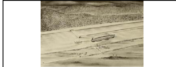
"...The uncertainty of safety of navigation under all tidal conditions led to consideration of a new concept: the installation of a tidal control structure at each end of a long restricted reach to limit the velocities of flow in a sea-level canal. It is contemplated that one structure and gate would be located close to the Pacific entrance and another 24 to 25 miles north thereof. The check gates would be moved alternately into position across or out of the channel at intervals of 6.2 hours or some multiple thereof when the Pacific is at the same level as the Atlantic. Under these conditions, the maximum velocity of flow would be approximately 2 knots at the Pacific entrance and less elsewhere. It is also contemplated that structures for gates would be built close to the Atlantic entrance where, if a gate were installed and employed alternately with the Pacific gate, the maximum velocity could be held to approximately 3 knots..." RE: excerpt from the Atlantic-Pacific Interoceanic Canal Study Commission report, 1970 Above: caption: "Artist's sketch of a Tidal Check at the entrance to a Bypass Channel"
