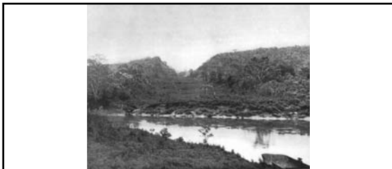
5—BIRD'S-EYE OF LOCKS AND DAM. CHAGRES RIVER IN THE FOREGROUND. THERE WILL BE WEIR IN THE BEND CUT BEYOND THE RIVER.
