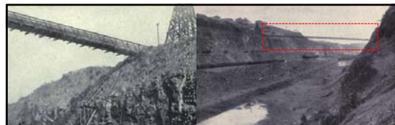
Above: caption: "Culebra Cut at Empire Suspension Bridge. Bottom of cut to be 57 feet lower than the train cars."
