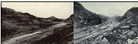
Left: view looking south toward the eastern bank of Culebra Cut, opposite Contractor's Hill, showing the terraced bank ca. 1890. This was the condition the French Canal Company left the cut in when they ceased operations. Work in the cut did not resume until 1905.
