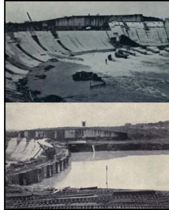
Top: caption: "Gatun Spillway looking South-West, showing downstream face of Ogee Dam, June 6, 1912"
